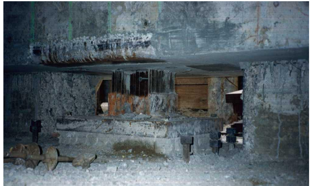
Cutting hole for jacks and column removal
