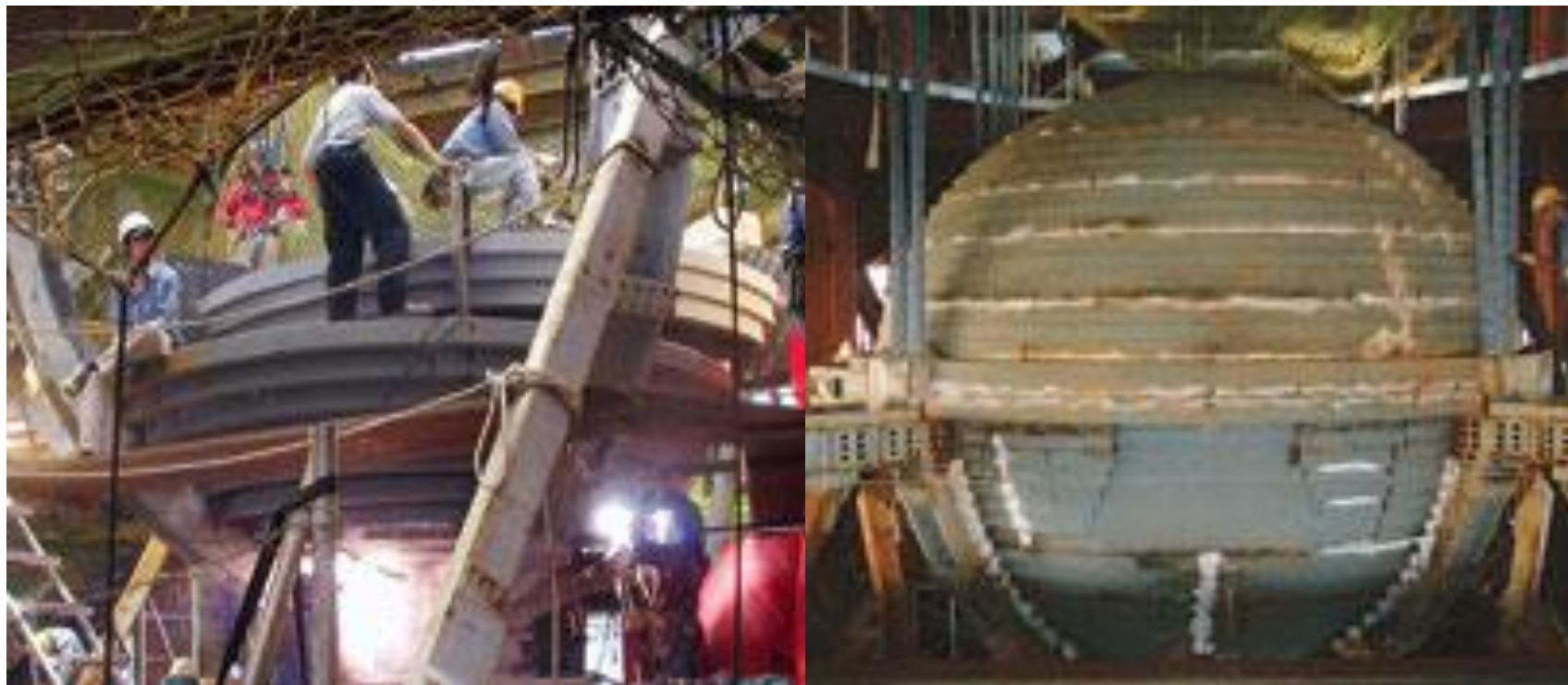
Assembly of the Tuned Mass Damper
