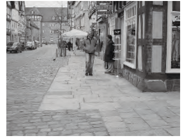
In the pedestrian zone in Melsungen, old pavement slabs from Berlin were reused in a very precise way.
