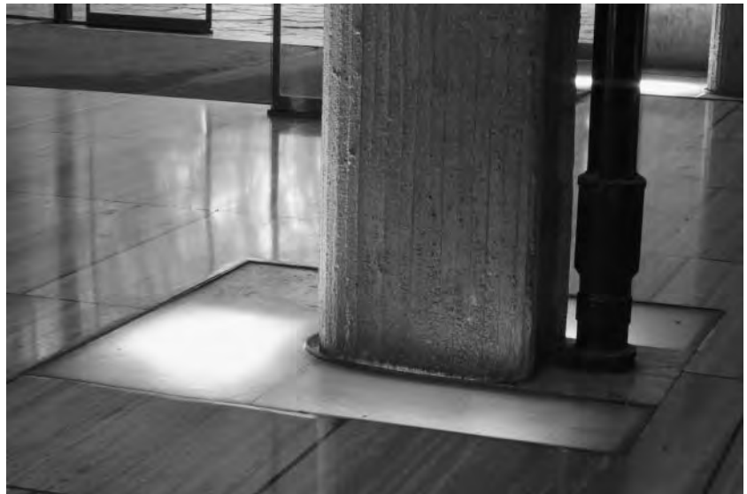
Figure 3.15 Lights in hall at base of pilotis, Unité, Marseilles Michelet (1952)
