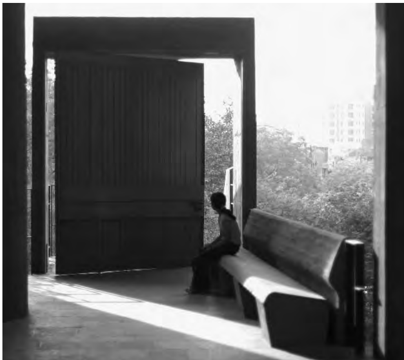
Figure 5.12 Bridged entrance to Mill Owners' Association Building, Ahmedabad (1954)
