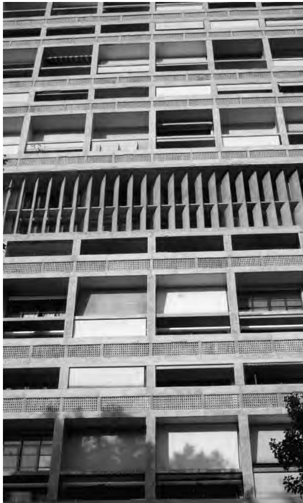
Figure 3.3 Brise soleil, Unité, Marseilles Michelet (1952)
