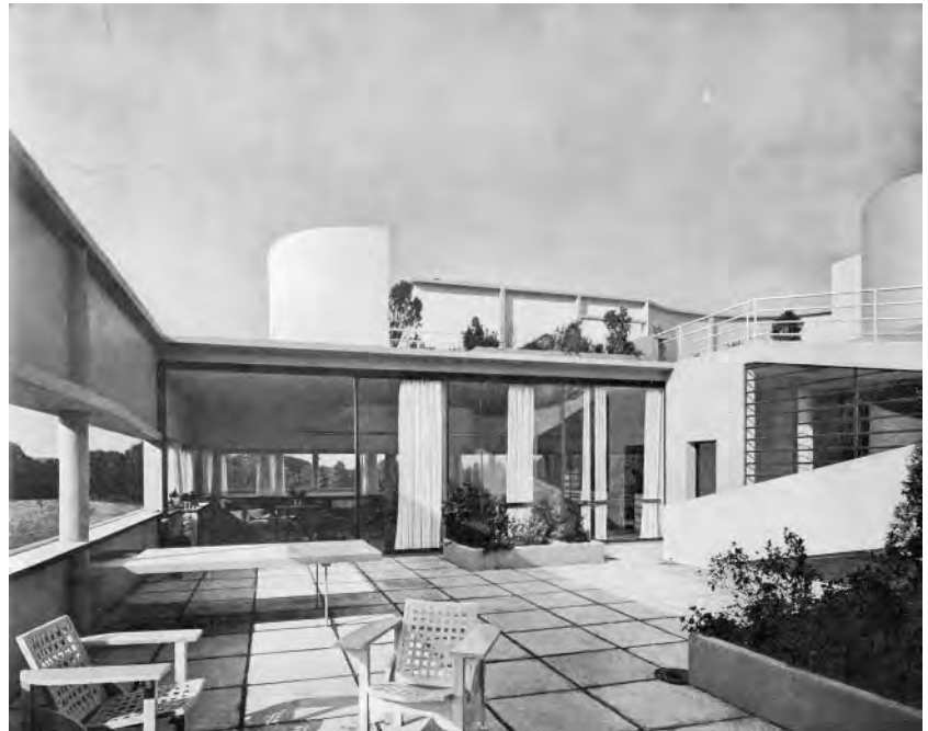
Figure 6.2 Table in roof garden of Villa Savoye (1930)
