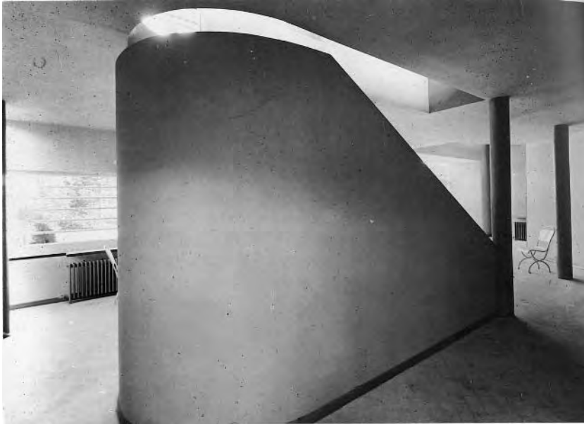
Figure 4.6 Stairwell Villa Savoye (1930). Photo from Le Corbusier's Oeuvre Complète
