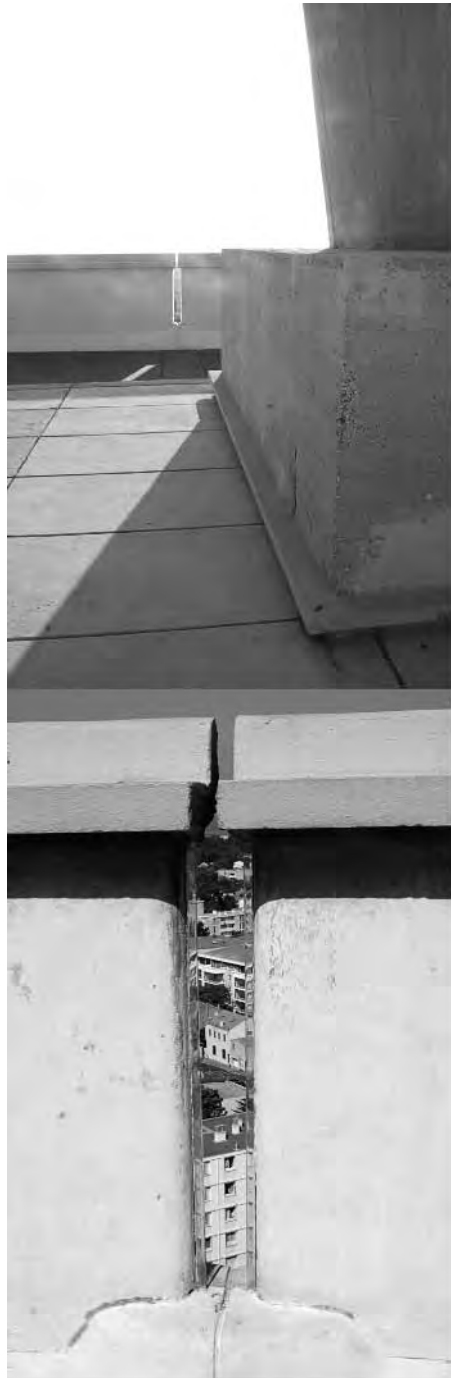
Figure 0.1 Expansion joint in parapet on the roof of the Unité Marseilles (1952)
