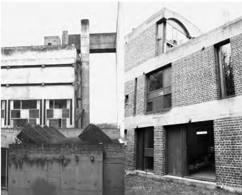
Figure 2.15 Details of exterior Maison Jaoul B (1955) and of La Tourette (1953–59)
