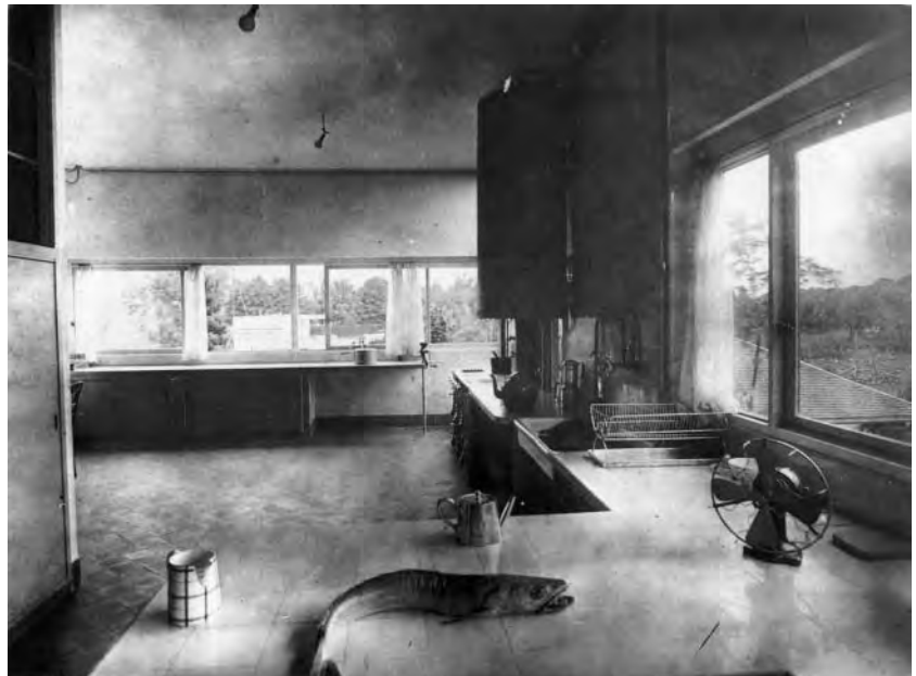
Figure 6.29 Kitchen, Villa Savoye (1930) from Le Corbusier's Oeuvre Complète
