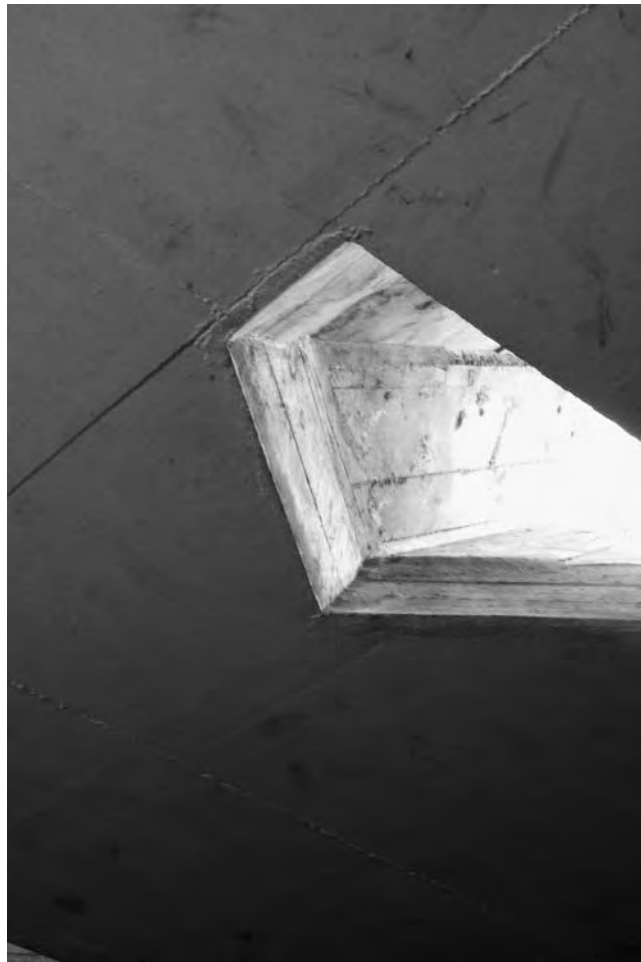
Figure 3.9 'Mitraillette' rooflights over the sacristy La Tourette (1959)
