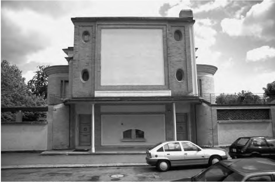
Figure 4.22 Exterior of Villa Schwob (1917) Charles Edouard Jeanneret (Le Corbusier)
