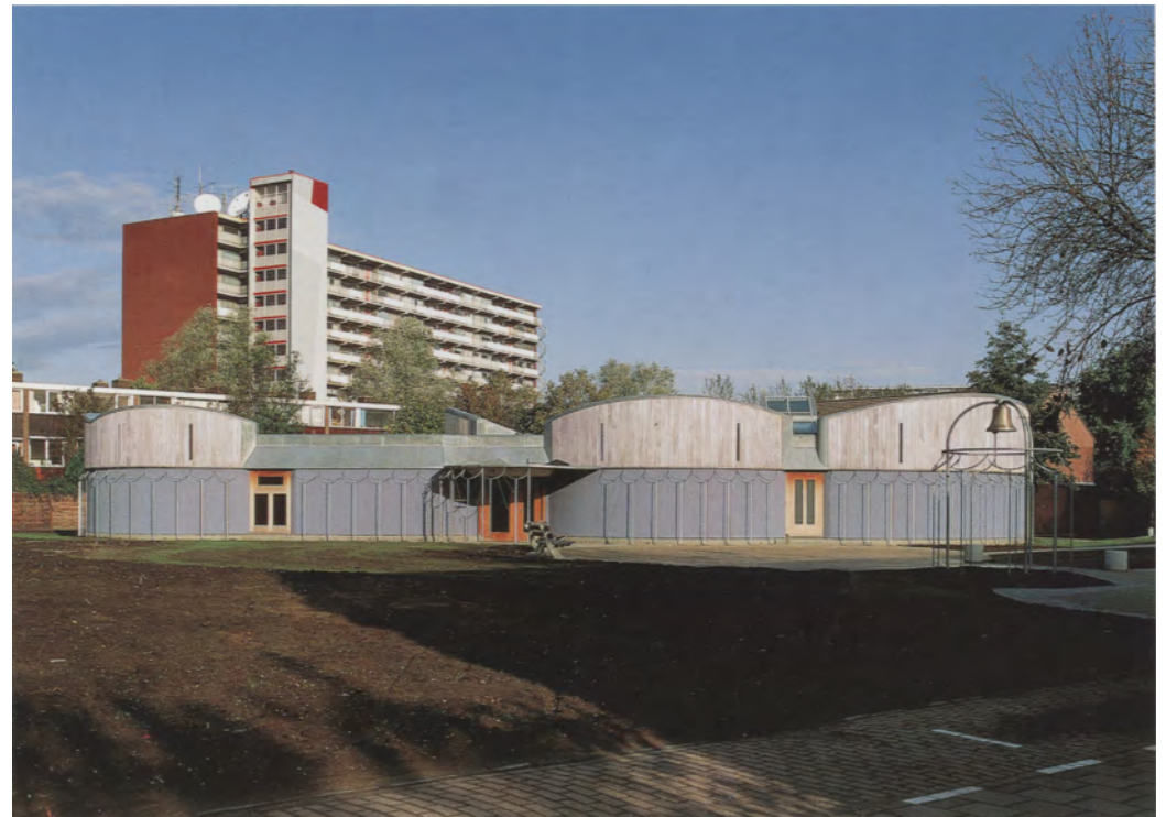
Entrance from the south, under the zinc roof on the right the ancillary rooms | View from the north, on the left the profane functions, on the right the sacred functions, on the far right the bell frame
