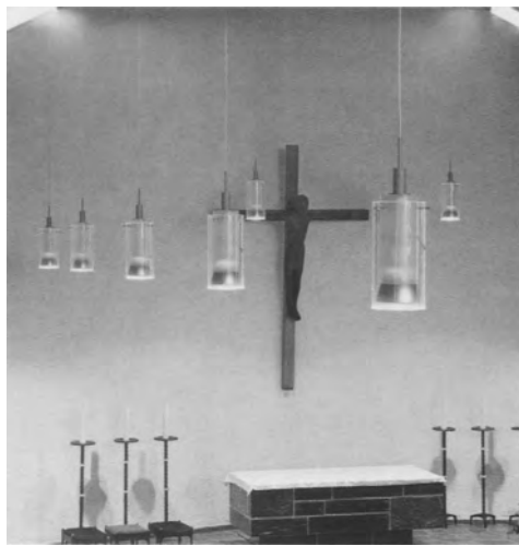
6 Karl Hans Neumann, Church of St Joseph, Münchingen, 1962 Directional light: dual-state switchable glass cylinder light fittings provide directional light for the altar and pews. The lighting provides additional reading light by day and illuminates the church service in the evenings. The matt silver reflector is visible inside the transparent housing of the light fitting
