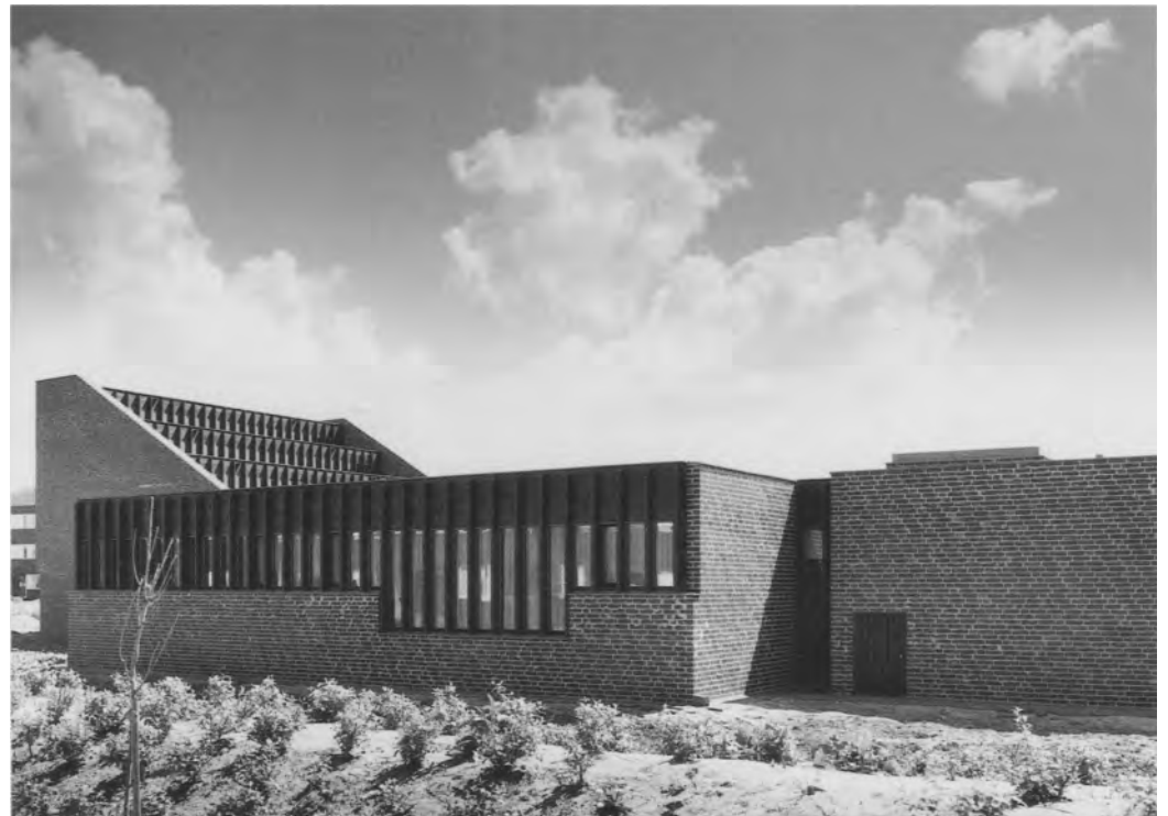
View from the southeast, entrance in the background | View from the northwest, in front the row of windows of the youth centre, behind the stepped roof of the nave | Parish hall, in the top centre the opening for the bells | Internal courtyard looking to the southwest, youth centre in the background | Nave of the main church with fourfold stepped skylight, right the transition to the parish hall, left the vertical shaft with the bells
