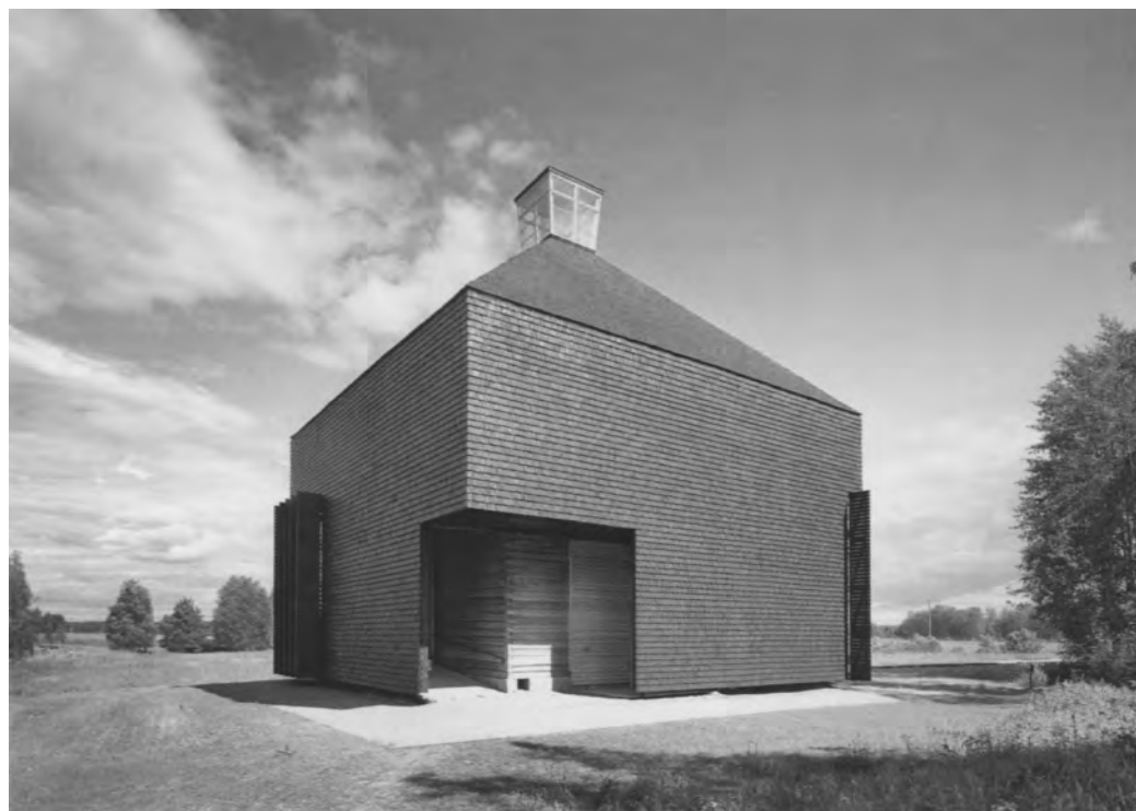
View from the northwest with the shutters | View from the southwest, the entrance to the sacristy on the right of the near corner, to the left the ramp leading to the vestibule | Entrance with ramp in east-west direction, a section of the room-high shutters is visible in the background | Vestibule with the banks of the river in the background | The church looking towards the door to the sacristy with the altar beside it
