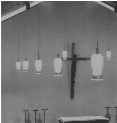
8 Karl Hans Neumann, Church of St Joseph, Münchingen, 1962 Diffuse light: a translucent inner cylinder containing an economical compact fluorescent lamp produces diffuse ambient lighting for daytime church services
