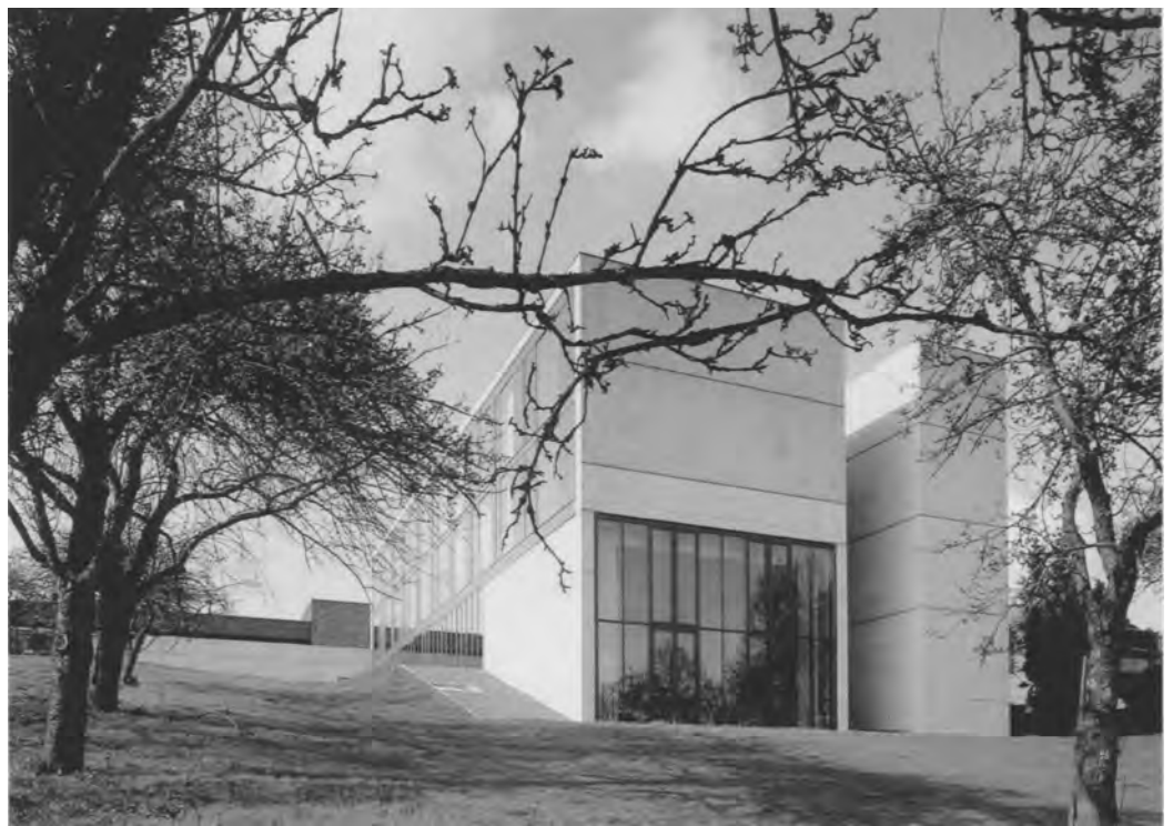
Entrance face opposite the abbey church | Rear of the building, the hall in the broader of the two blocks, to the left the guest room windows | Steel-and-glass bridges between both wings, in the background the abbey church | Room for prayer and contemplation with hidden rooflight | Cell with view westwards
