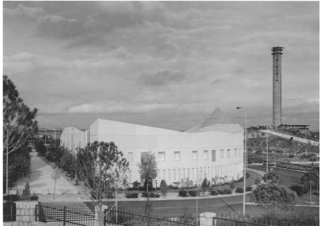
View from the east, left the church, right the parish hall | View from the south, behind the windows ancillary rooms below, dwellings above | View from the north, behind the stone wall the garden | The church, to the right as if floating, the sculpture above the altar, on the left the pews made of toble.
