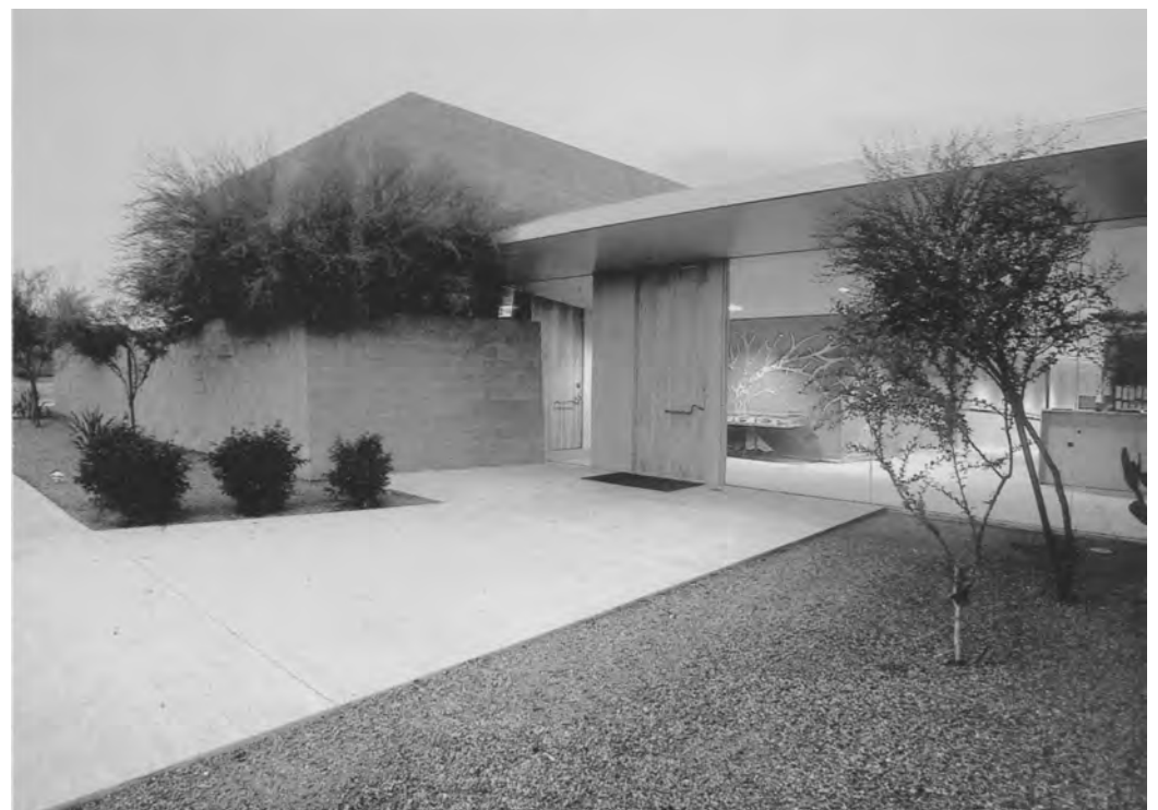
View of the synagogue from the northeast showing concrete masonry | Main entrance, on the right the passage through to the courtyard, on the left the art garden, walled on three sides, with the synagogue behind it
