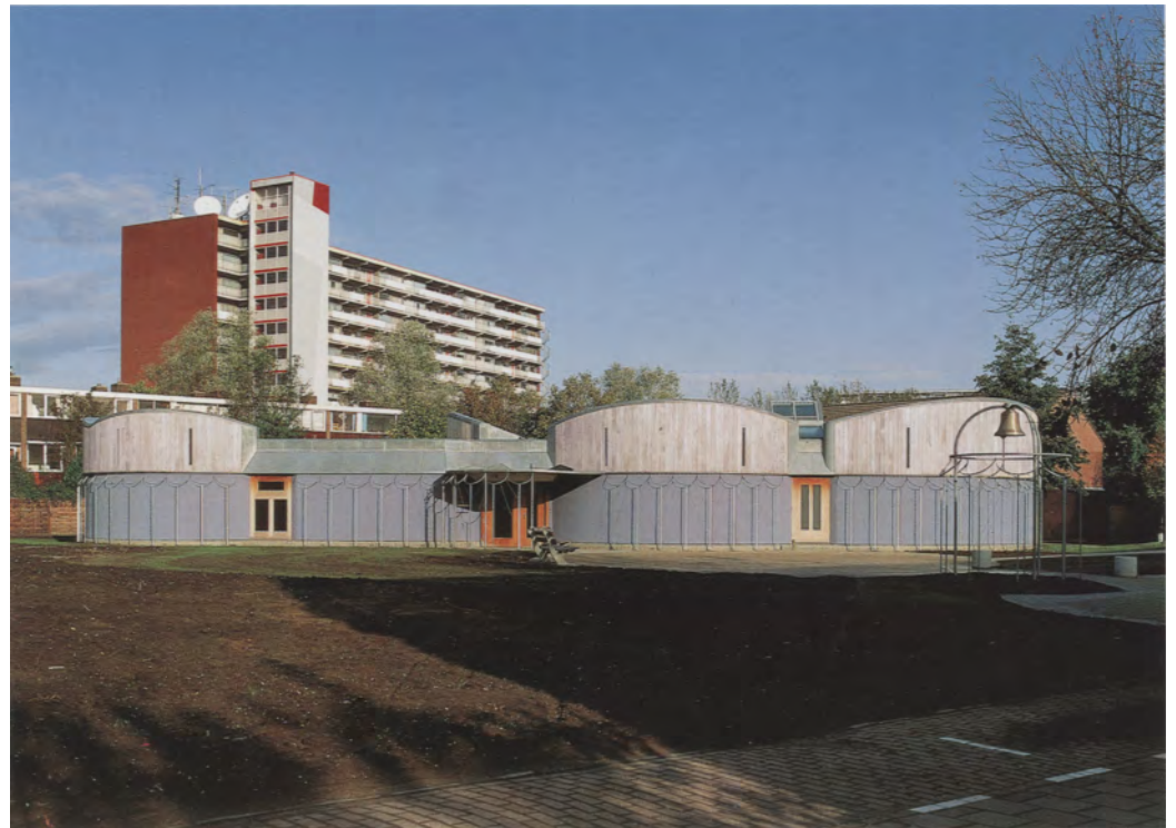
Entrance from the south, under the zinc roof on the right the ancillary rooms | View from the north, on the left the profane functions, on the right the sacred functions, on the far right the bell frame
