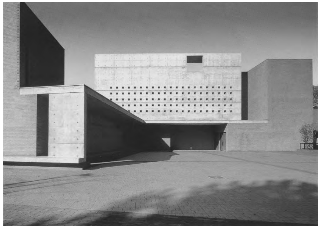
View from the southwest, at the back on the right between the towers of the baptistry and campanile, the priest's residence | Courtyard with chapel and corridor on the left, the concrete facing of the main building | View southwest with the island of the altar on the left, the gridded wooden panels in the concrete ceiling contain lighting and heating elements | The Chapel of Our Lady on the northeast side of the building | North face of the main hall with view into the garden court
