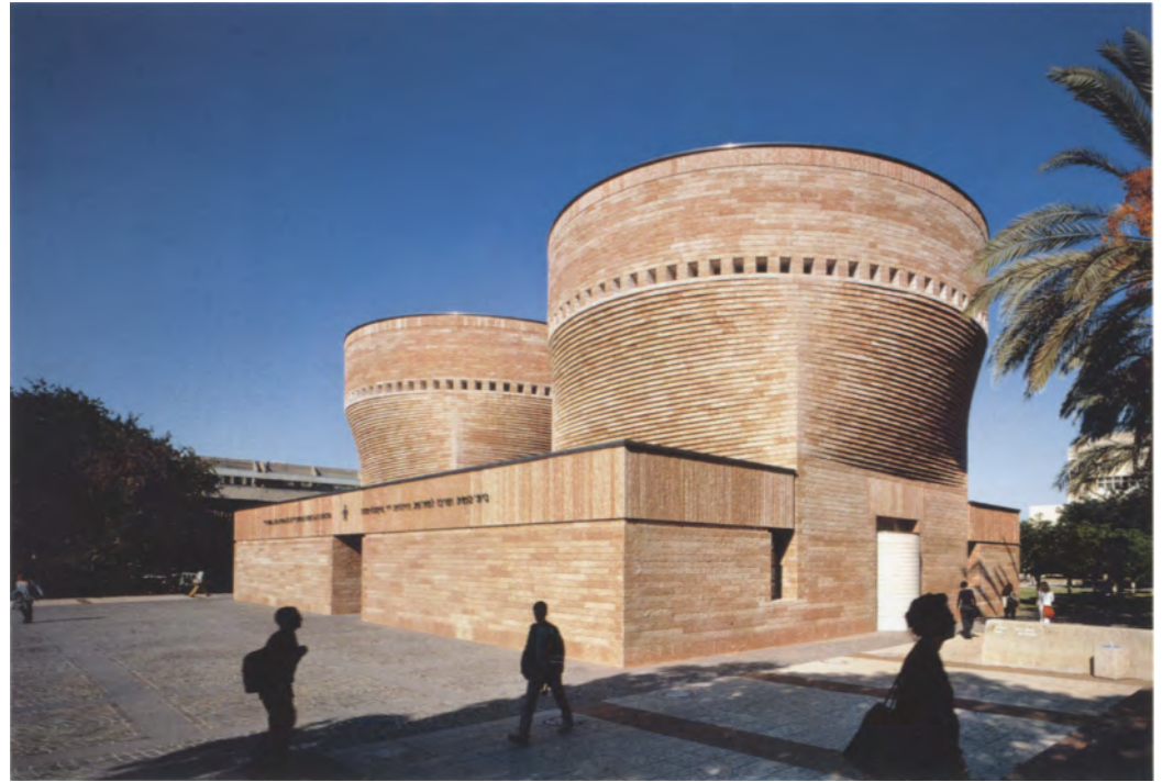
View from the north | View from the southeast | View of the orthodox synagogue from north | Masonry skin made of Pietra di Prun stone showing the transition from stepped to vertical brickwork
