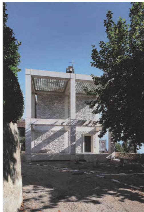
View from the southwest | View from the west towards the "forecourt" | Stepped portal of the oratory, to the right the fresco with the depiction of the Annunciation | View of the altar zone with two of the three light slots in the background
