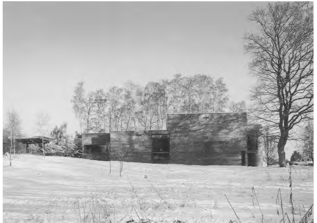
The church hall from the east, clear glass mounted in black steel frames | View from the west, right the high space of the church, left the low canopy
