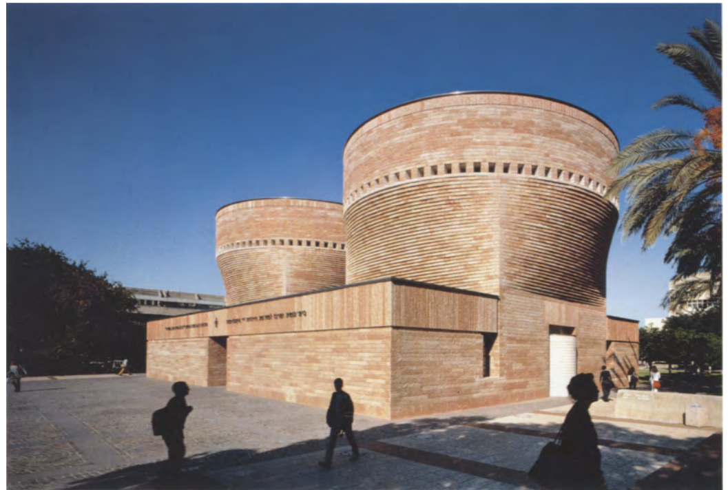
View from the north | View from the southeast | View of the orthodox synagogue from north | Masonry skin made of Pietra di Prun stone showing the transition from stepped to vertical brickwork
