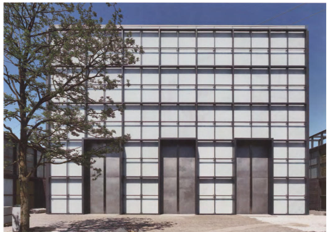
Night-time view of arcade, cloister, tower and pavilion | Front face of the pavilion with external structural framework and translucent panels of stone-glass | Interior view of the pavilion with altar and pews in the background, coffered ceiling above | Cloister, to the right some of the filled glass panels
