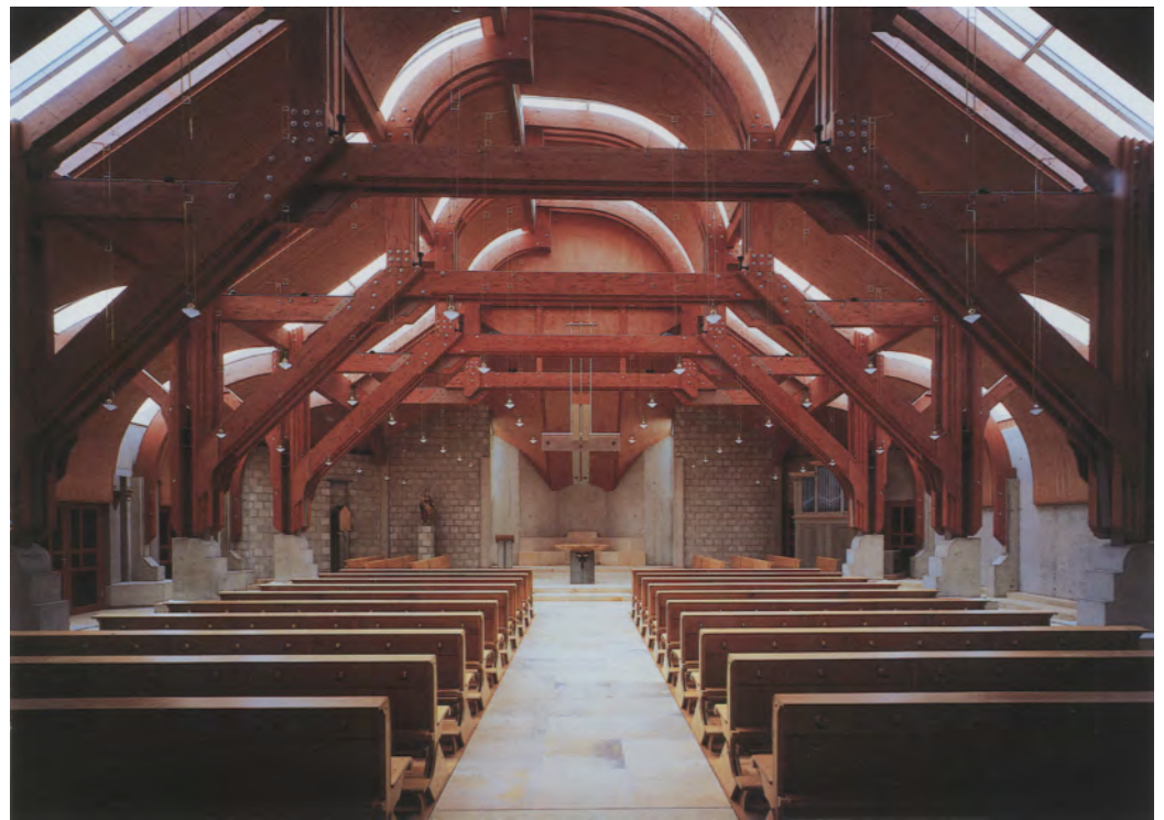
Entrance to the church | Central aisle towards the altar | View from the ambo and altar towards the entrance, on the left a footing of the laminated truss beams | Strips of boarding and glass between each pair of laminated truss beams, in the background the baptistry
