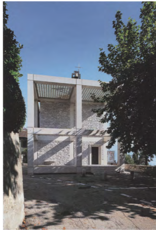
View from the southwest | View from the west towards the "forecourt" | Stepped portal of the oratory, to the right the fresco with the depiction of the Annunciation | View of the altar zone with two of the three light slots in the background
