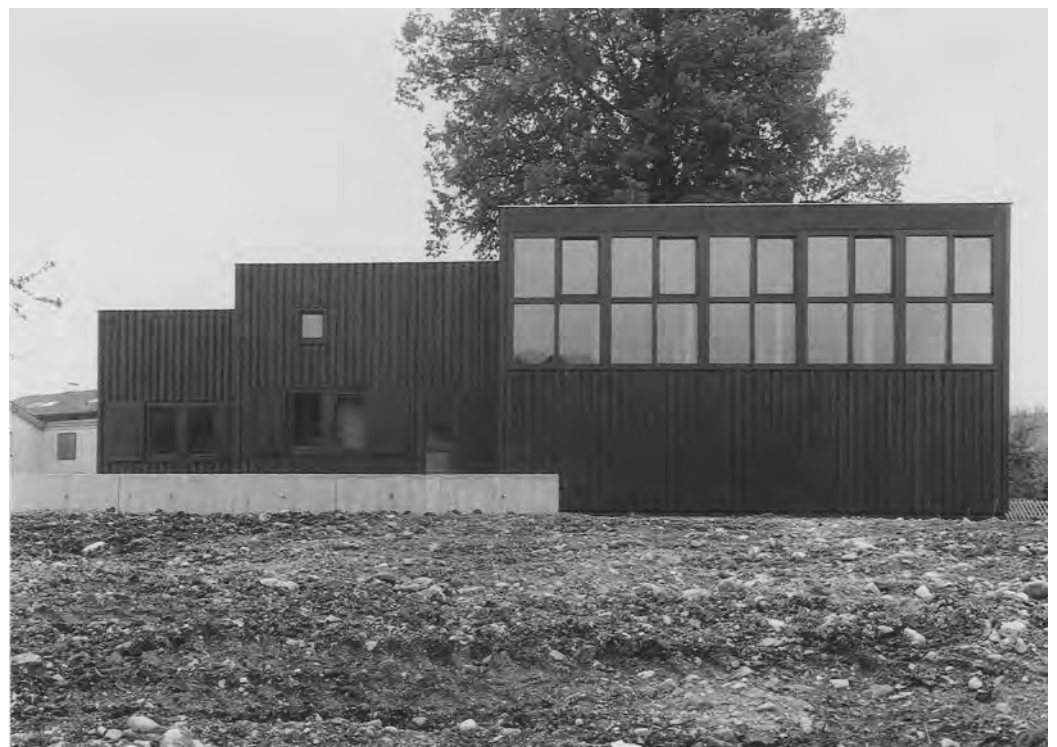
View from the south | View from the north, left the seating wall | Part of the "entrance hall" with way through to the church space | View from the hall looking west, above right the mullioned windows
