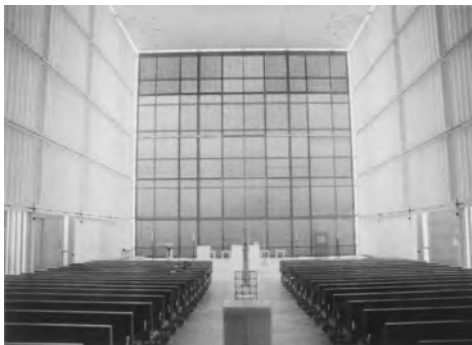
3 Allmann Sattler Wappner, Sacred Heart of Jesus Church, Munich, 2000 The church space is enclosed by a wooden shrine placed within a translucent rectangular glass volume. The mean daylight factor around the altar is 6.2 per cent. Towards the back of the pews, this value drops to 2.5 per cent as the structure of the wooden slats becomes more closed.
