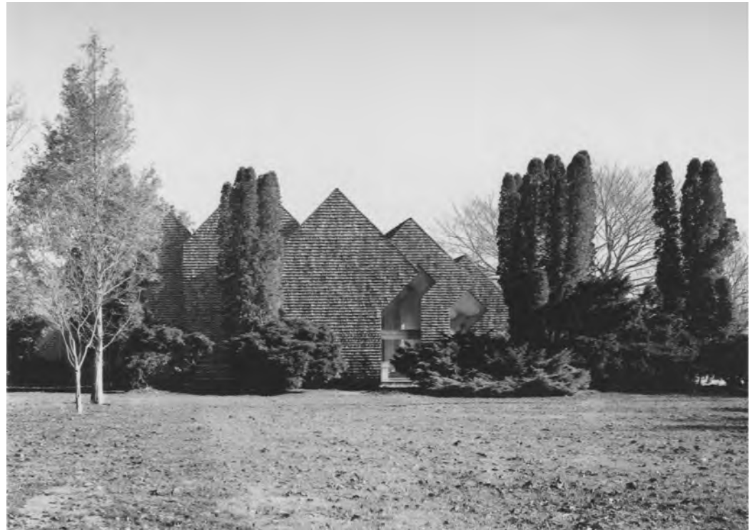
Anteroom with view westwards | View from the west showing the series of pointed gables
