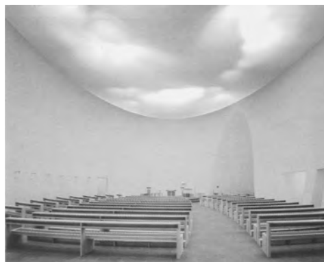
5 Königs Architects, Church of St Francis, Regensburg, 2004 Light falls through a translucent membrane hung beneath the sawtooth roof providing a diffuse light within the church. When the sun shines, the sawtooth roof casts shadows on the membrane; when the sky is overcast the membrane provides a bright even light. When it is dark, lights mounted between the roof and membrane throw cloud-like formations onto the membrane. The daylight factor near the altar is 1.5 per cent, around the pews a constant 1.2 per cent
