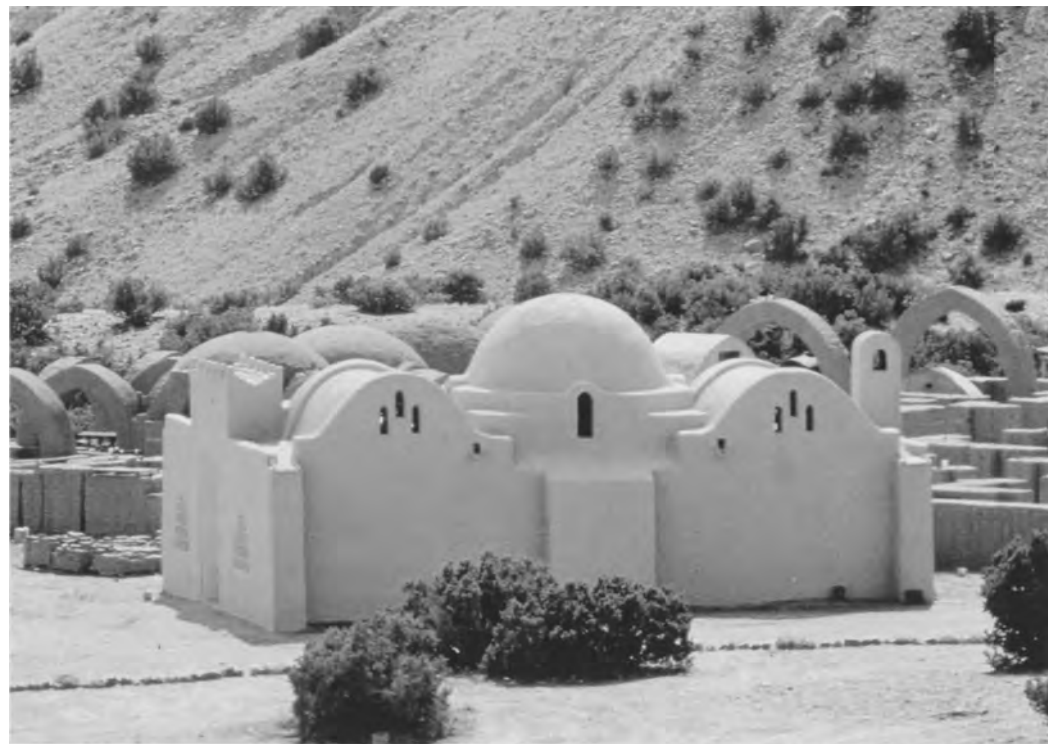
Aerial view of the partially completed complex of the mosque and school, mosque on the right | View of the mosque from the southeast, the mihrab is visible as a projection in the centre of the wall
