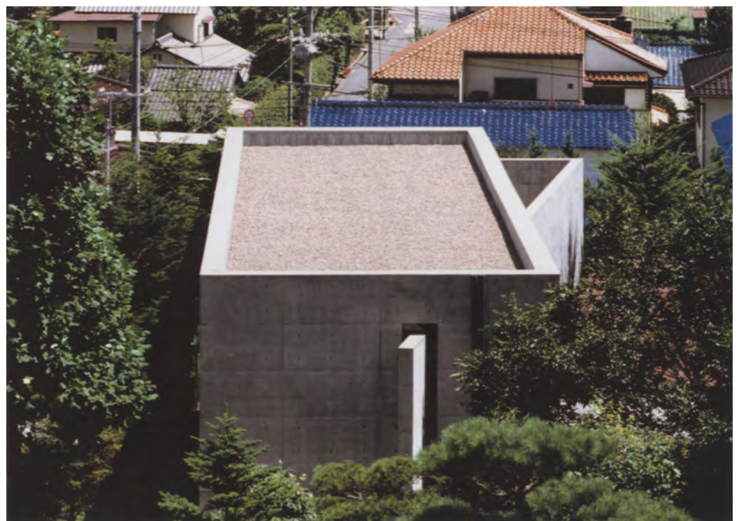
View from the north | View of the rear wall with the sign of the cross | Full-height glazed section of the west wall with a reflection of the sign of the cross | West side with the long flank of the diagonal wall; just visible on the right, the "vestibule"
