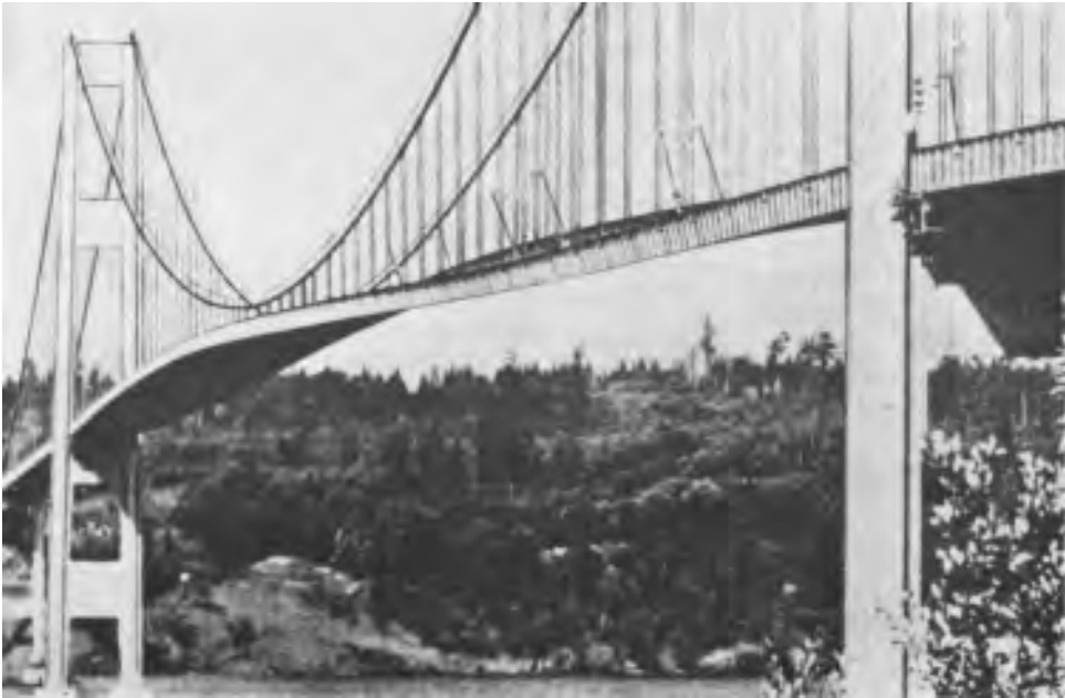
Figure 2.4. Instantaneous photograph of the galloping Tacoma Narrows bridge in the anti-symmetric torsional mode before collapse [from Scruton (1971)].
