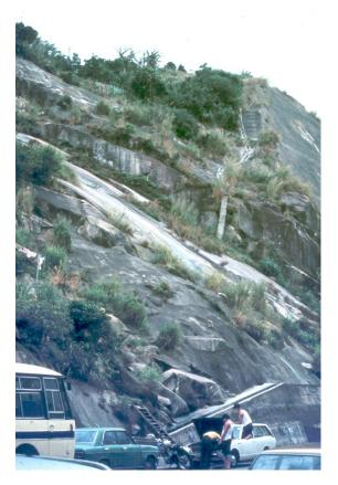
The potentially unstable slope under consideration is visible in the background of this photograph. It is obvious from this photograph that the sheet joint surface continues under the potentially unstable slope. Hence, from the evidence of the small scale failure, it can be deduced that the factor of safety of the slope in question is not very high.
