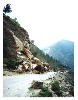
Figure 3: A rock slide on a road caused by the undercutting of sheet joints in a granite slope. In hard rocks such as granite, failure can occur very suddenly if the factor of safety of the slope is close to 1. A rise in groundwater levels during a heavy storm or ice jacking in winter may be sufficient to induce failure.
