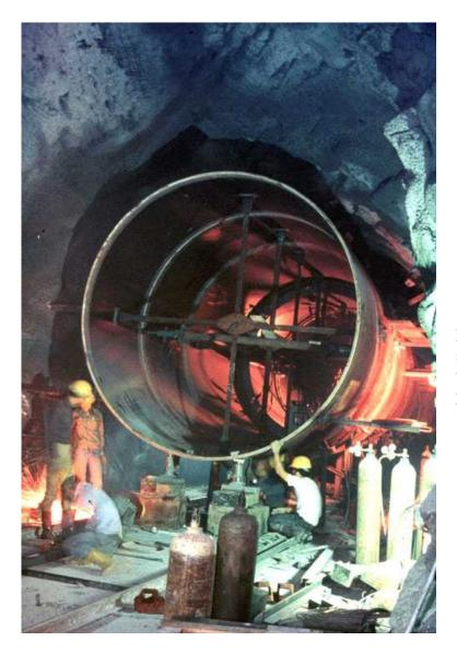
Figure 13: Installation of steel lining in a pressure tunnel in a hydroelectric project.
