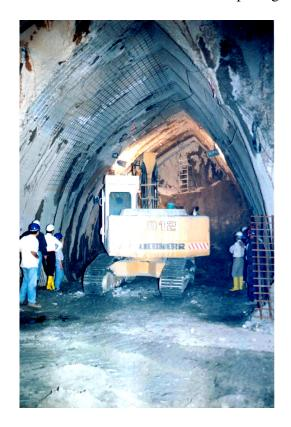
Figure 27: Side drift in the Athens Metro Olympion station excavation that was excavated by the method illustrated in Figure 25. The station has a cover depth of approximately 10 m over the crown.
