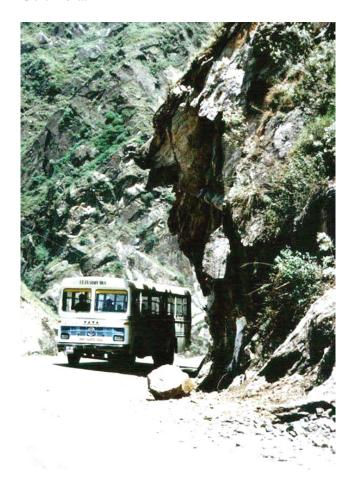
Figure 1: A rock slope on a mountain highway. Rockfalls are a major hazard on such highways
