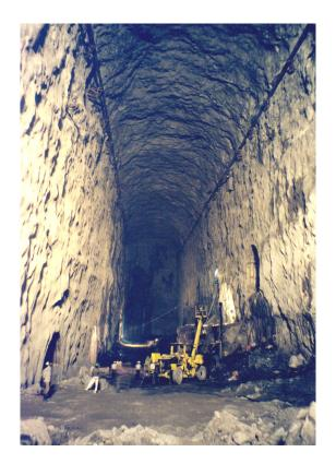
Figure 22: Partially completed 20 m span, 42.5 m high underground powerhouse cavern of the Nathpa Jhakri Hydroelectric Project in Himachel Pradesh, India. The cavern is approximately 300 m below the surface.
