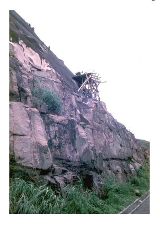
Figure 10: Drilling horizontal drain holes into the face of one of the benches of the Sau Mau Ping slope.
