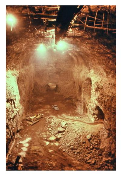
Figure 7: A view of the 25 m span Rio Grande power cavern during excavation of the lower benches.
