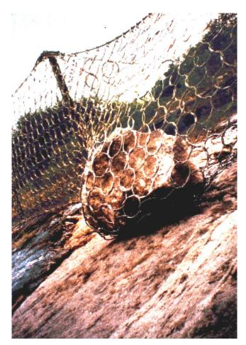
b: Geobrugg ring net shown restraining a boulder. These nets can be designed with energy absorbing capacities of up to 2500 kNm which is equivalent to a 6 tonne boulder moving at 20 m per second.
