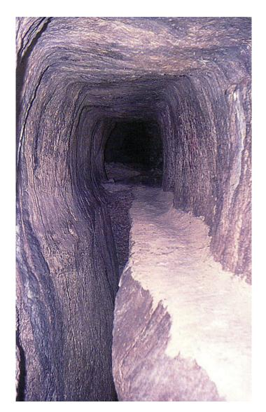
Figure 5: The 1036 m long Eupalinos water supply tunnel was built in 530 BC on the Greek island of Samos. This is the first known tunnel to have been built from two portals and the two drives met with a very small error.
