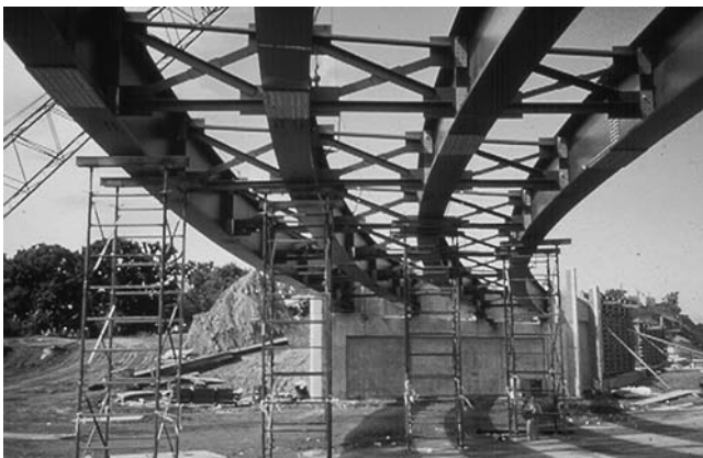
Fig. 6.2 Curved girder bridge erection bracing.
