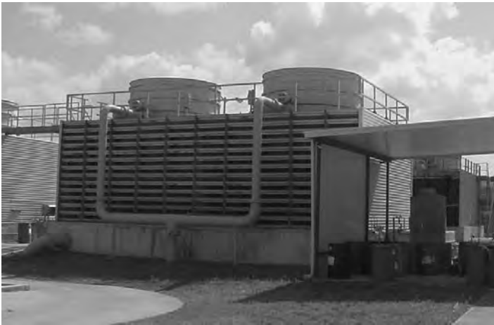
Figure 6.5.1. Cooling Tower for Example Problem
