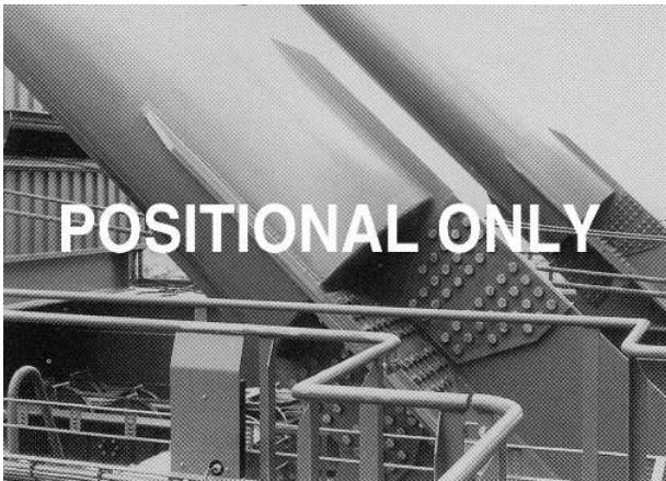
Fig. 7.3.1 Bolted connection
