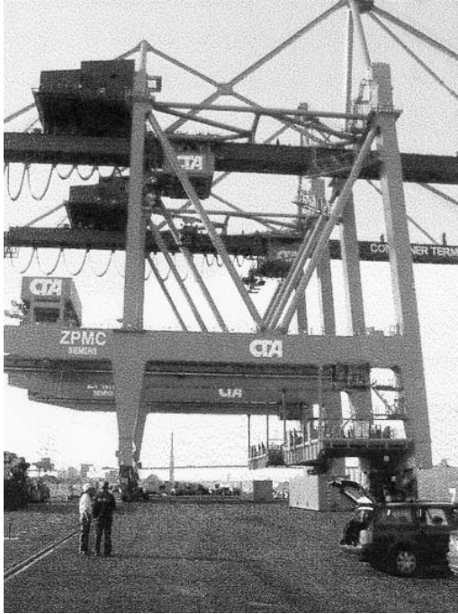
Fig. 6.12.3 Crane with laser scanners
