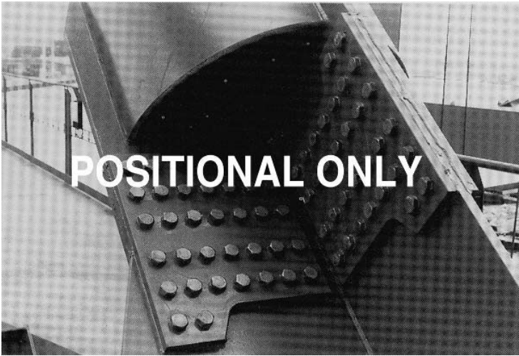
Fig. 7.5.8 Bolts in a back tie
