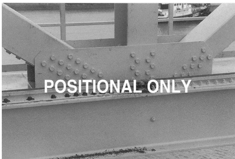
Fig. 7.4.3 Bolted construction
