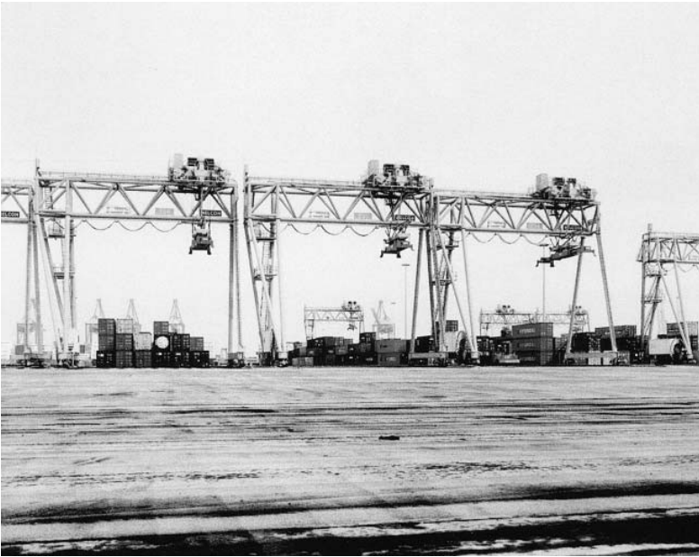
Fig. 6.13.1 ASCs with Spreader Positioning Systems
