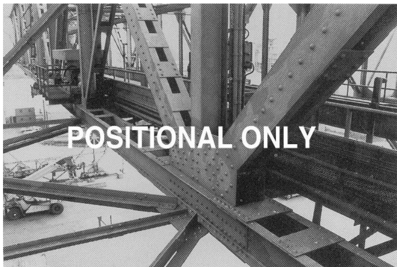
Fig. 7.4.2 Riveted construction
