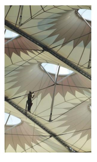
GMP, Olympic Stadium, Kiev, Ukraine, 2012 Membrane construction is a field that shows how new materials and construction methods can create innovative details, such as the trussed skylights in the new roof of the Olympic Stadium in Kiev which was conceived in close collaboration with engineers Schlaich Bergermann & Partner (sbp).
