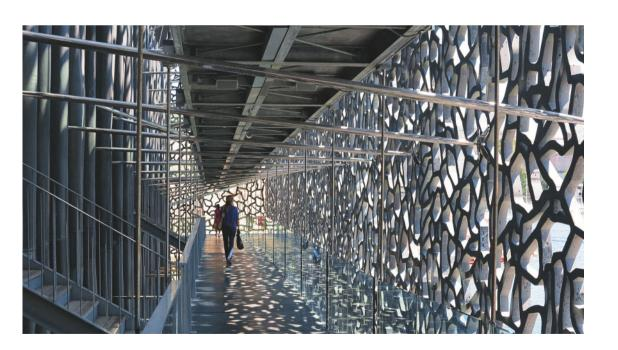
Rudy Ricciotti, Musée des Civilisations de l'Europe et de la Méditerranée (MuCEM), Marseille, France, 2013 The museum is the first building utilising ultra-high-performance concrete (UHPC) on a large scale. The fixation of the net-shaped diaphanous facade elements, however, is by means of 'frog fingers', a traditional method borrowed from glass construction.
