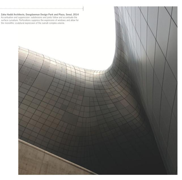
The tessellation of the aluminium facade follows a rule (script) that converts the smooth differentiation of degrees of curvature into the (stepped) differentiation of degrees of subdivision.
