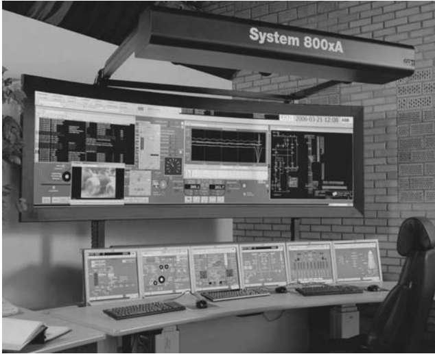
FIGURE 8.3 Large screen used to show details for a large group so that discussions can be made to solve problems together.
