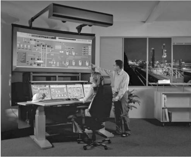
FIGURE 8.2 Modern control: The demonstration system at ABB.
