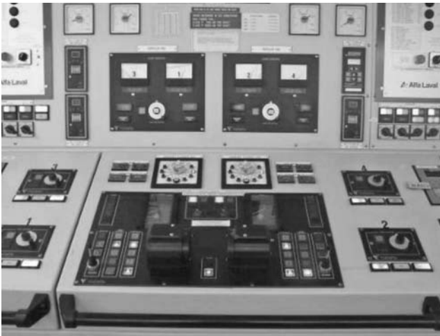
FIGURE 9.15 Functional grouping of instruments. (Photograph from E. Wagner. With permission.)
