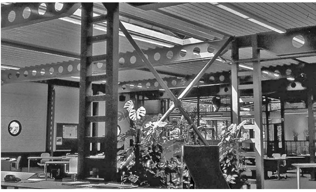
Figure 6.32. Battened columns
