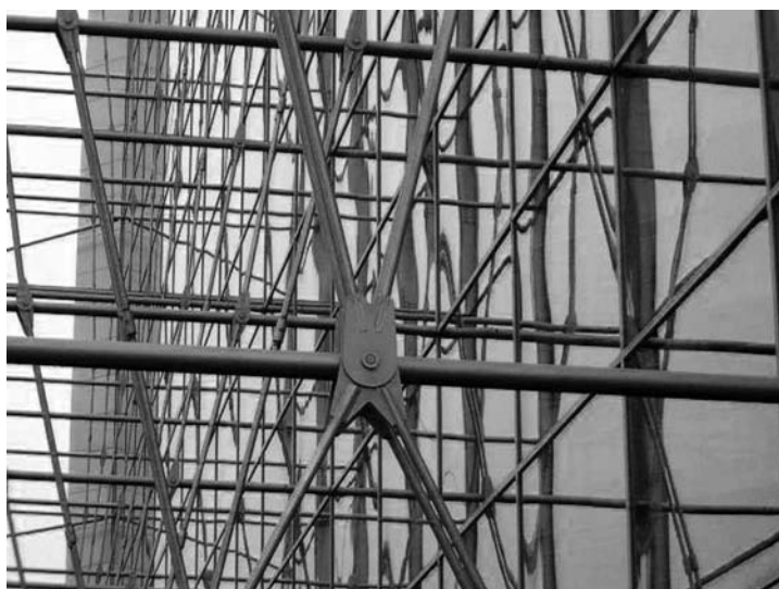
Figure 5.3. External diagonal bracing system (Sanomatalo Building, Helsinki)
