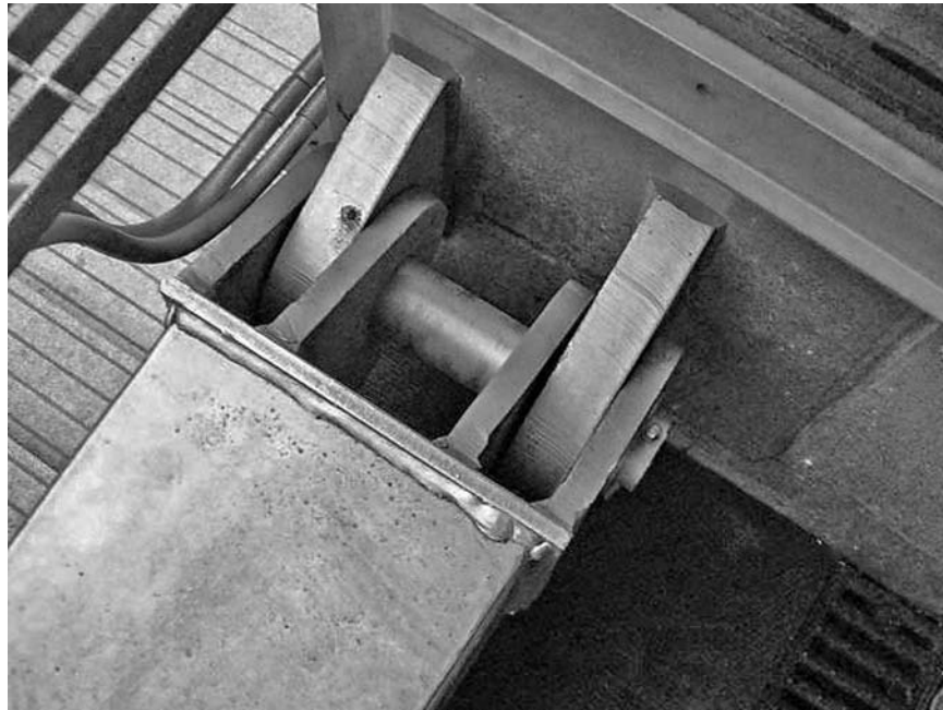
Figure 12.4. Pin connection
