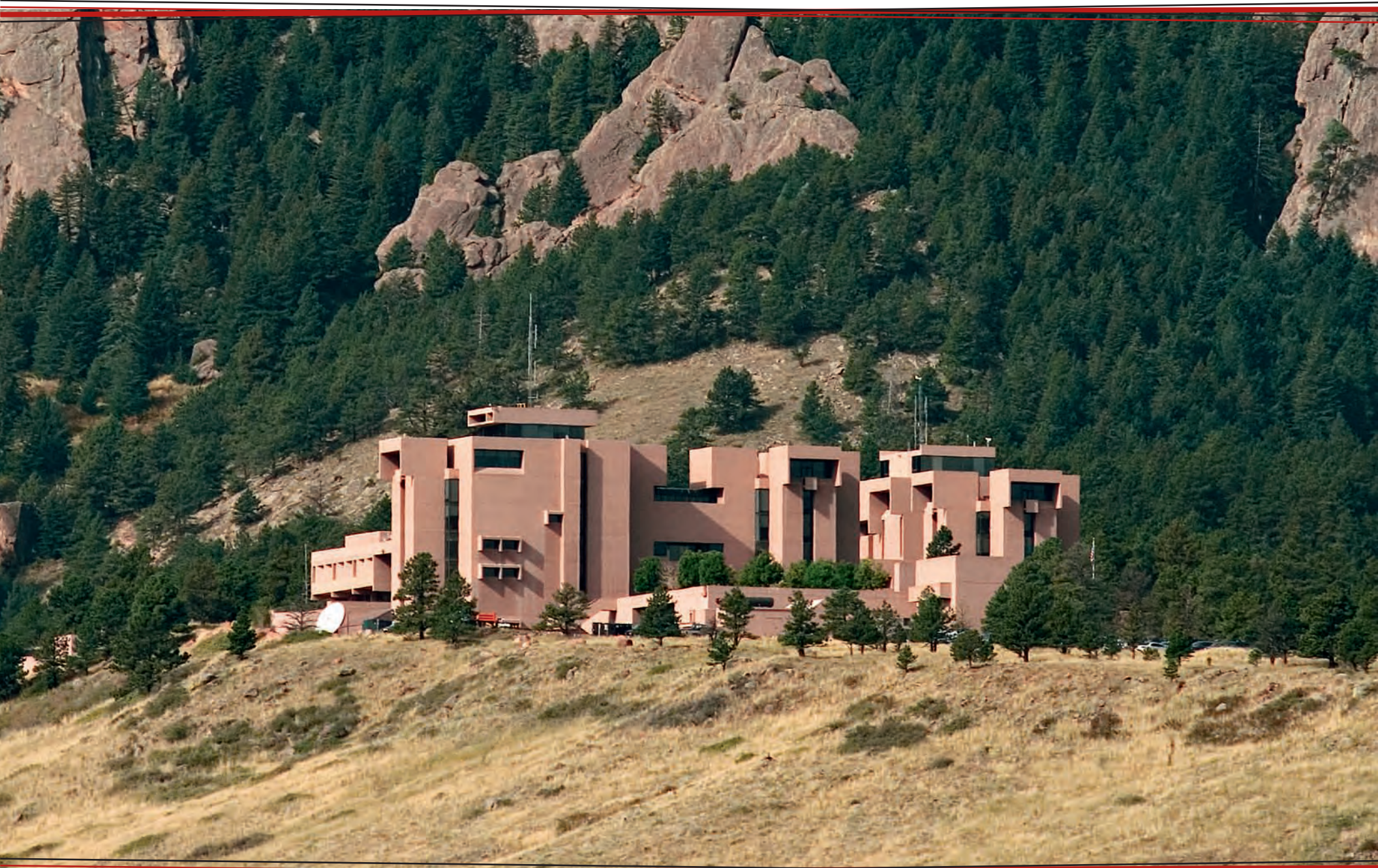
PEI'S FINISHED NCAR BUILDING NESTLES IN THE FOOTHILLS OF THE DRAMATIC COLORADO ROCKY MOUNTAINS, ECHOING THE RUGGED ROCK OUTCROPPINGS THAT RISE ABOVE IT.
