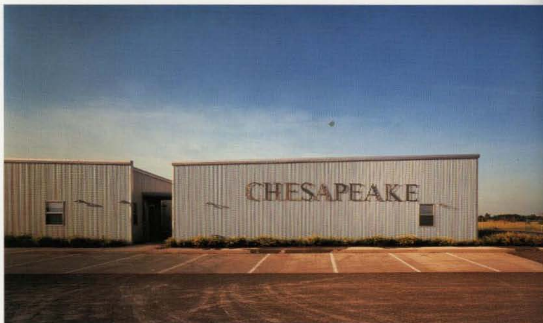
Chesapeake Waynoka Field Office Waynoka, Oklahoma, USA Elliott + Associates Architects 6 Partial north elevation 7 Service garage looking west Opposite: Entry courtyard looking south Photo credit: Robert Shimer/Hedrich-Blessing
