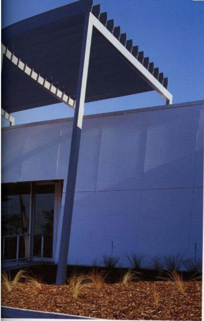
Snapfresh Brisbane, Queensland, Australia Woods Bagot Pty Ltd 2 View to main entry 3 Entry feature structure 4 Window feature through to internal meeting room 5 Staff amenities Photo credit: David Sandison
