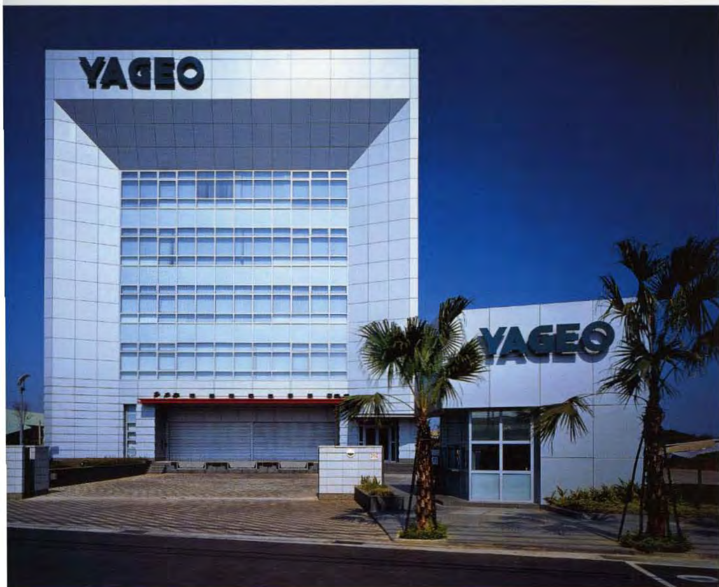
Yageo Corporation Kaohsiung Factory III Kaohsiung, Taiwan Haigo Shen & Partners Opposite: View from west 3 First floor plan 4 Front façade Photo credit: courtesy Haigo Shen & Partners
