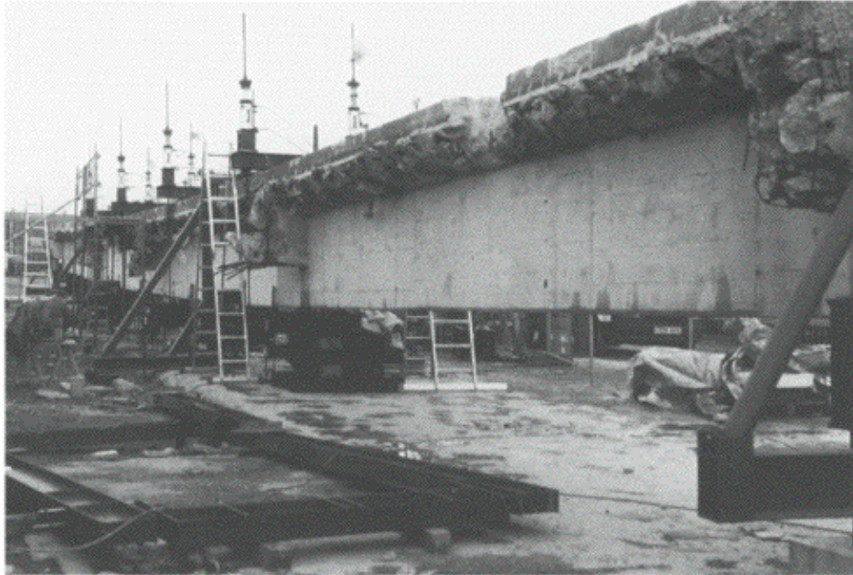
Figure 6.28 42 m prestressed concrete beam under final test load with 40 cm deflection.
