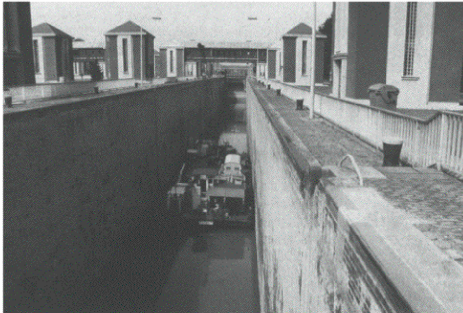
Figure 7.28 The currently inoperative basin of the double lock.
