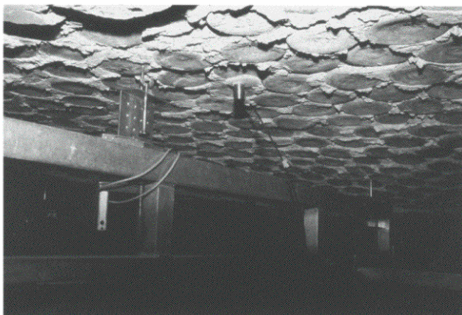
Figure 7.35 View from below the barrel vault with displacement transducers.
