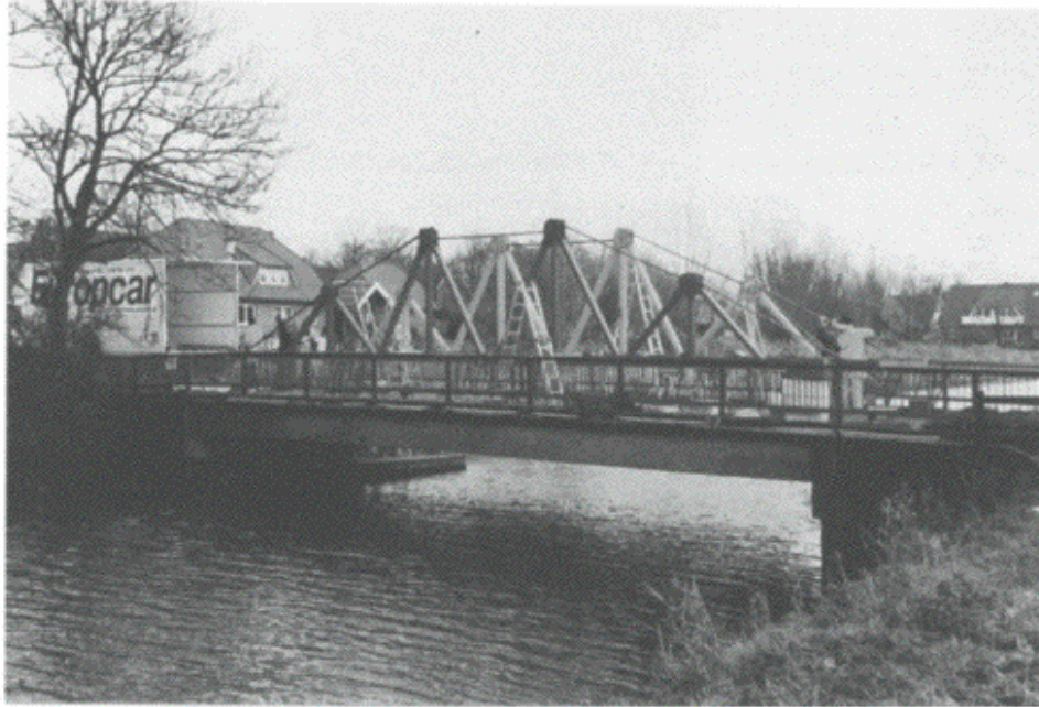
Figure 6.19 View of the bridge with loading frame.
