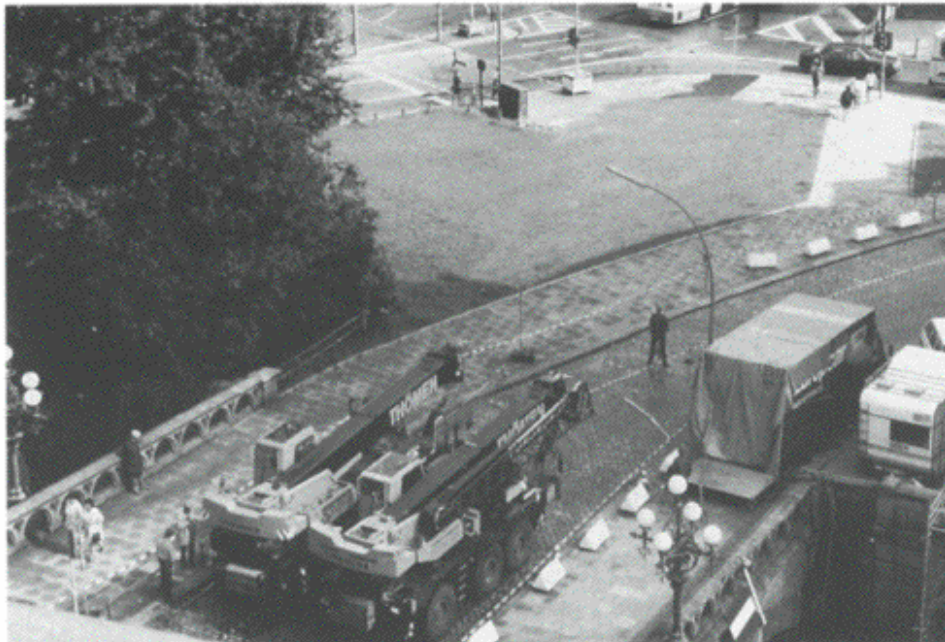
Figure 6.4 Mobile cranes as test load.
