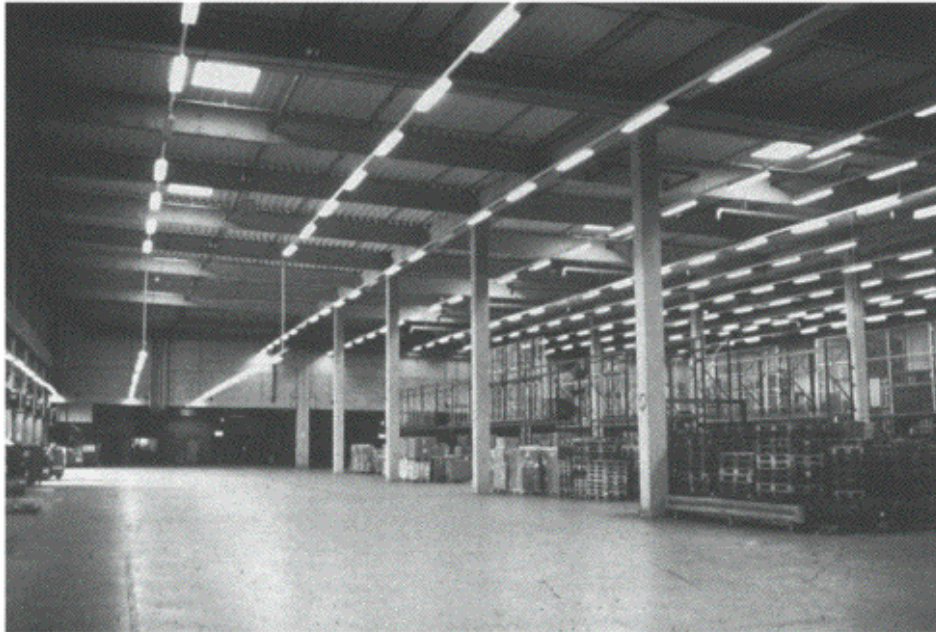
Figure 7.14 Stores building before installation of the high bay racking.
