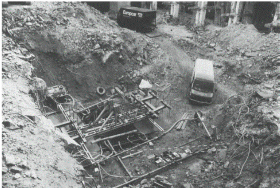
Figure 7.24 Excavation for the exposure of the test pile heads.
