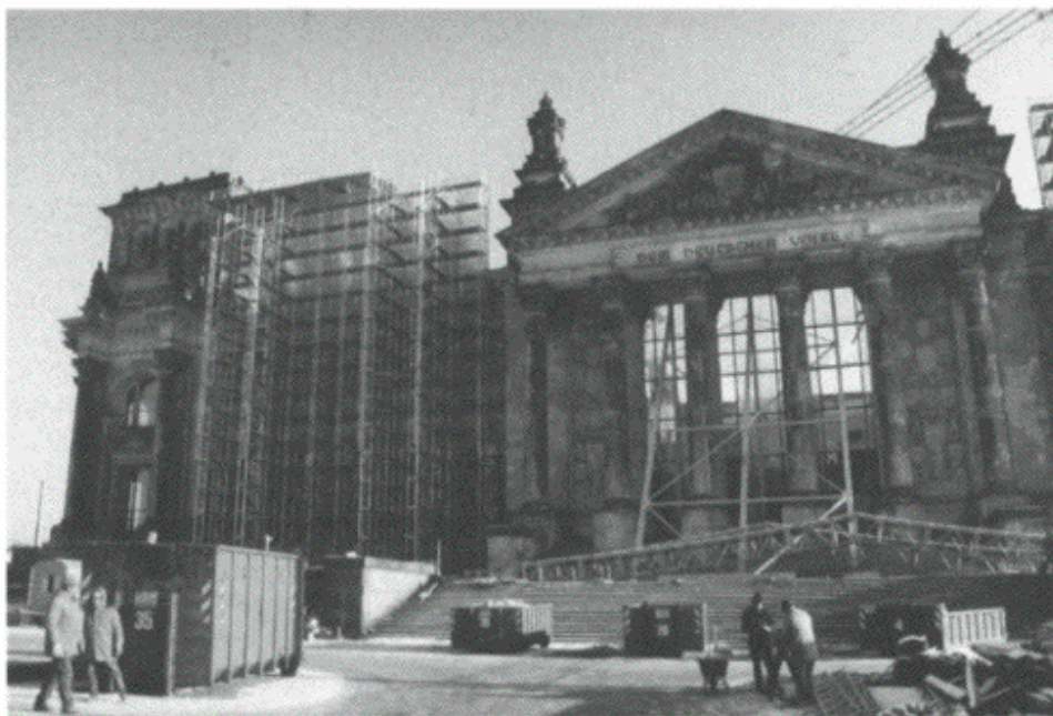
Figure 7.22 Main facade after removal of the internal structure.
