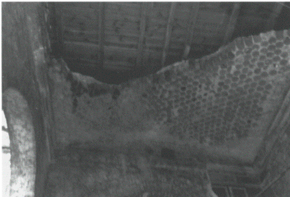
Figure 7.33 Barrel vault of clay pots with temporary roof.
