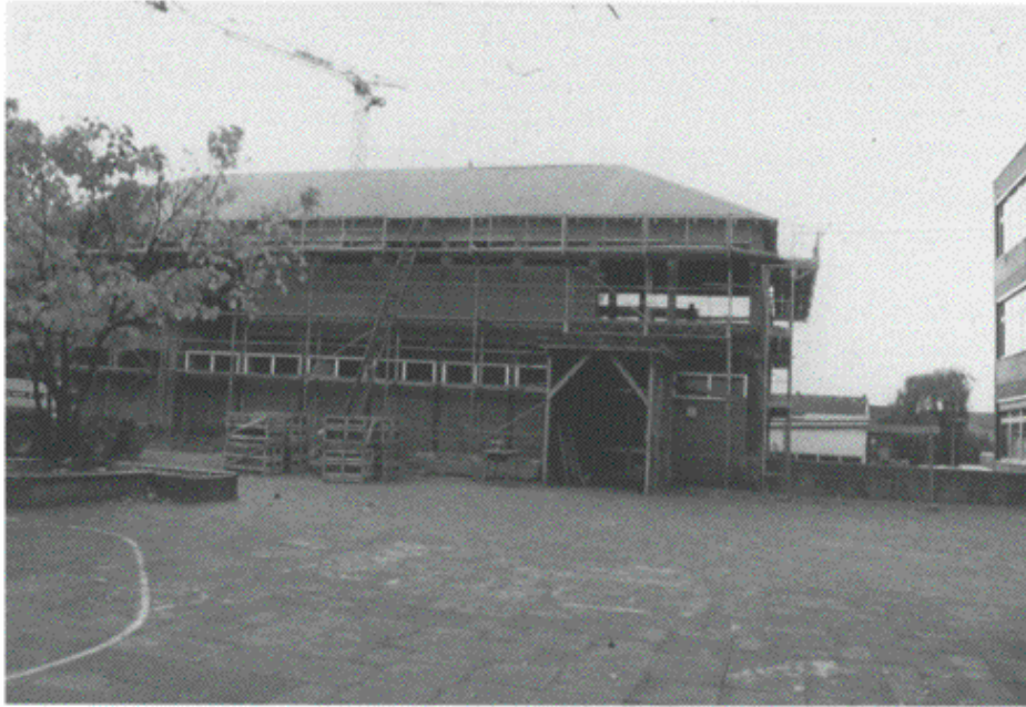
Figure 7.7 View of the building with the added level.
