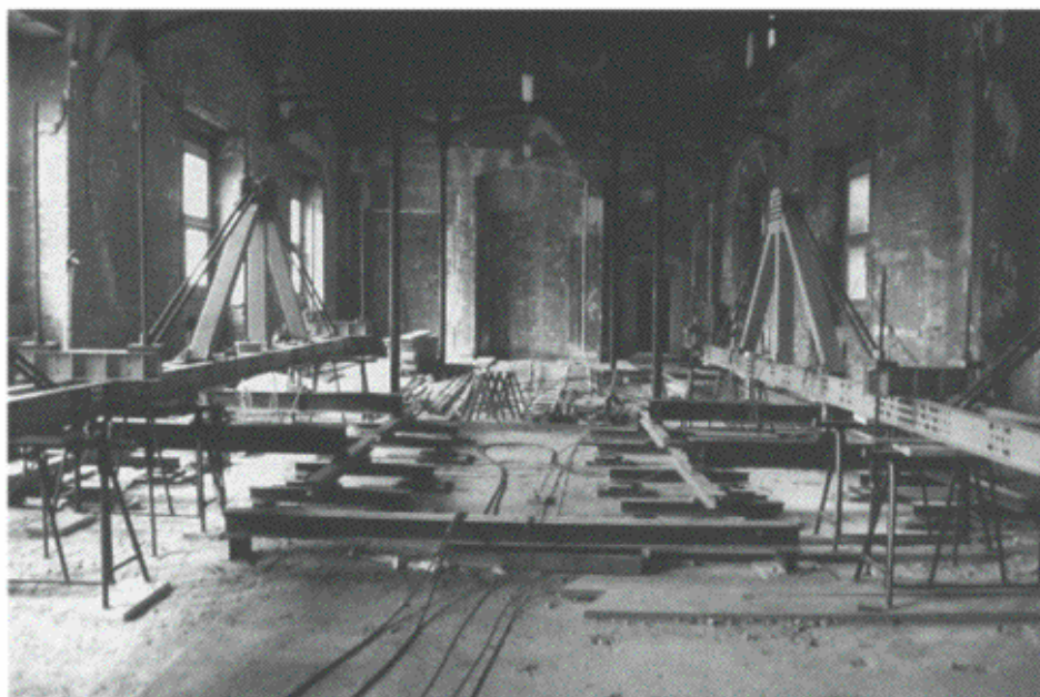
Figure 7.34 Loading device for the sampling tests.
