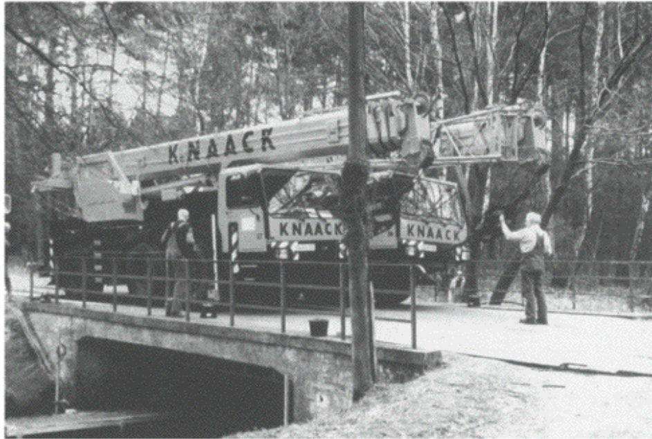
Figure 6.7 Production of the test load using two mobile cranes.
