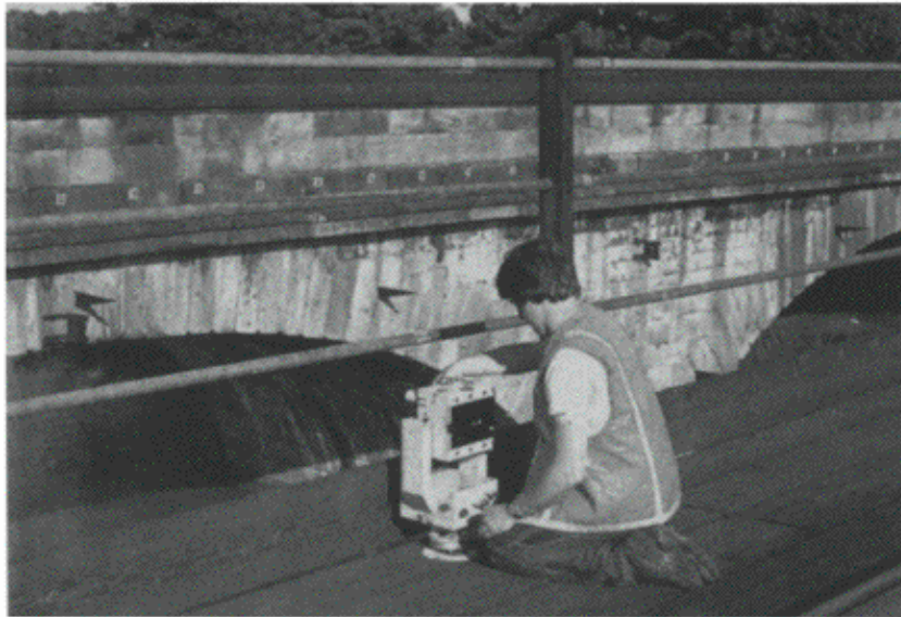
Figure 4.3 UMK being used to photograph railway viaduct. Visible on the viaduct are the targets used for the monitoring. Also visible are metal brackets which had been used for precise levelling surveys previously.
