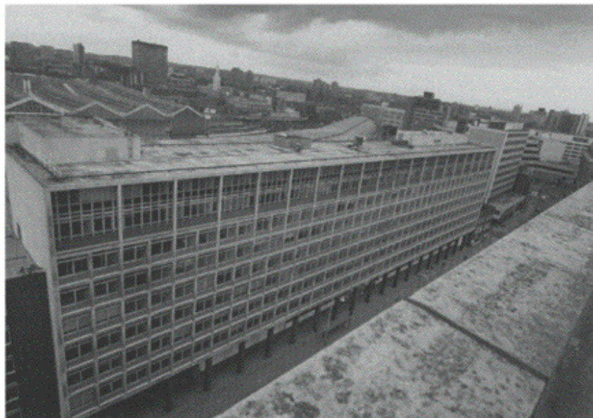
Figure 4.2 Sample UMK plate of building close to Waterloo Station, London. Plate taken for monitoring purposes related to Jubilee Line Extension tunnelling works.
