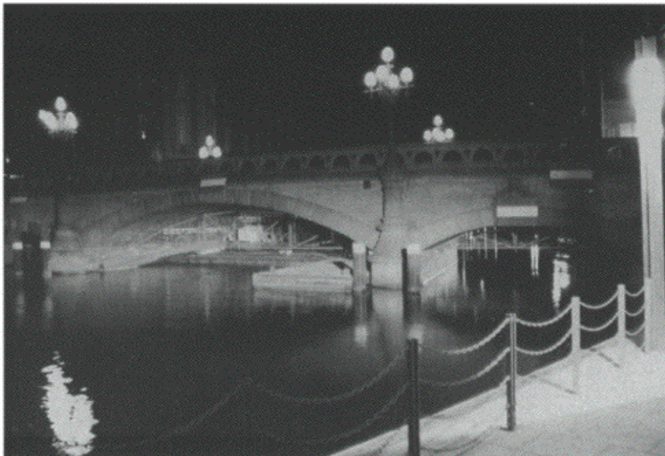
Figure 6.3 View of the bridge.
