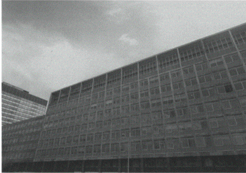
Figure 4.1 Sample UMK plate of building close to Waterloo Station, London. Plate taken for monitoring purposes related to Jubilee Line Extension tunnelling works.
