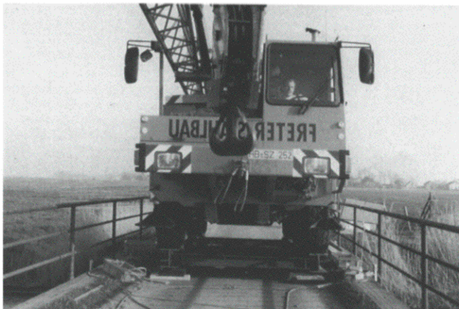
Figure 6.11 Mobile crane in the working position.
