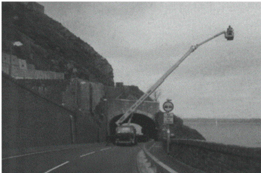
Figure 4.15 Hoist being used for A55 retaining wall photography.
