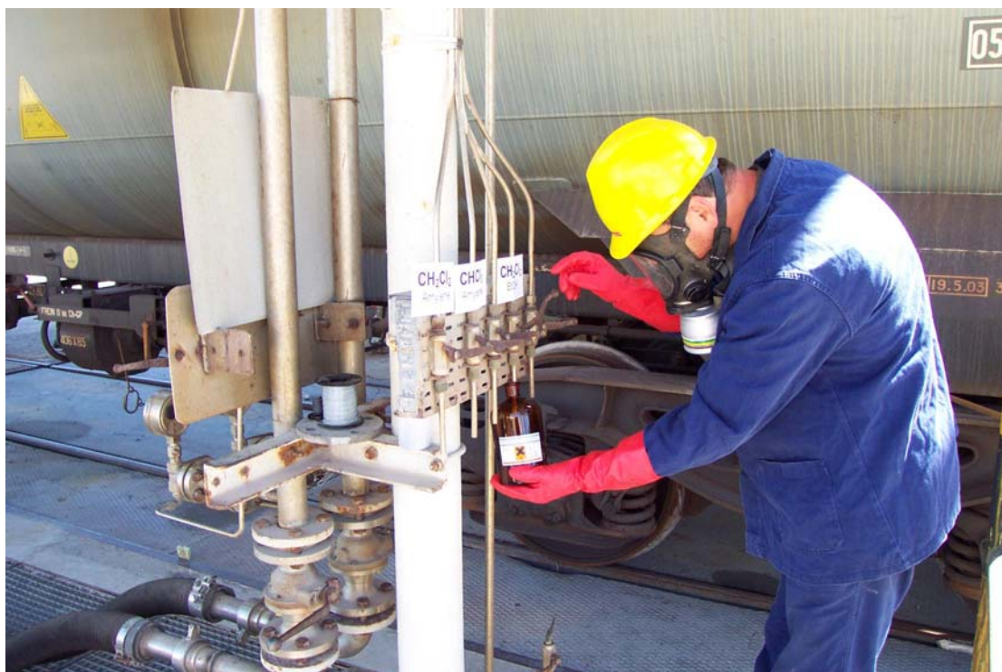
Sampling on pipeline during loading of a rail tanker
