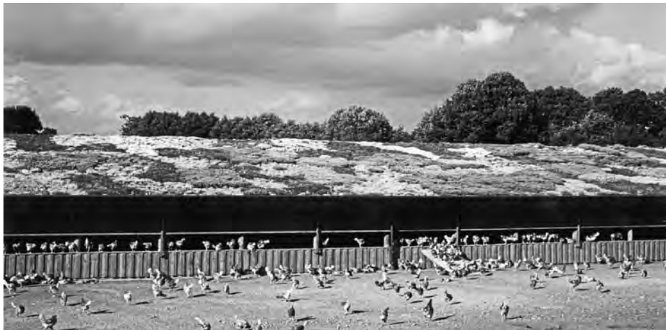
FIGURE 2-9 This multicolored living green roof is on a pitched roof of a chicken coop of this environmentally responsible poultry farm. (Photo: re-natur, 24601 Ruhwinkel, Germany)
