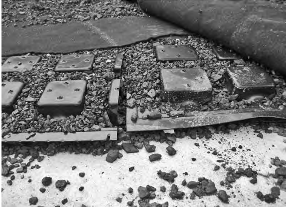
FIGURE 6-35 Drainage and reservoir panel close-up. The panel is filled with lightweight aggregate and covered with filter fabric to facilitate drainage and capillary movement of water.
