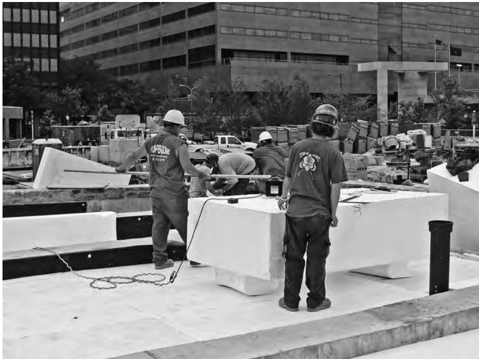
FIGURE 8-31 Installation of large blocks of EPs light-weight fill.
