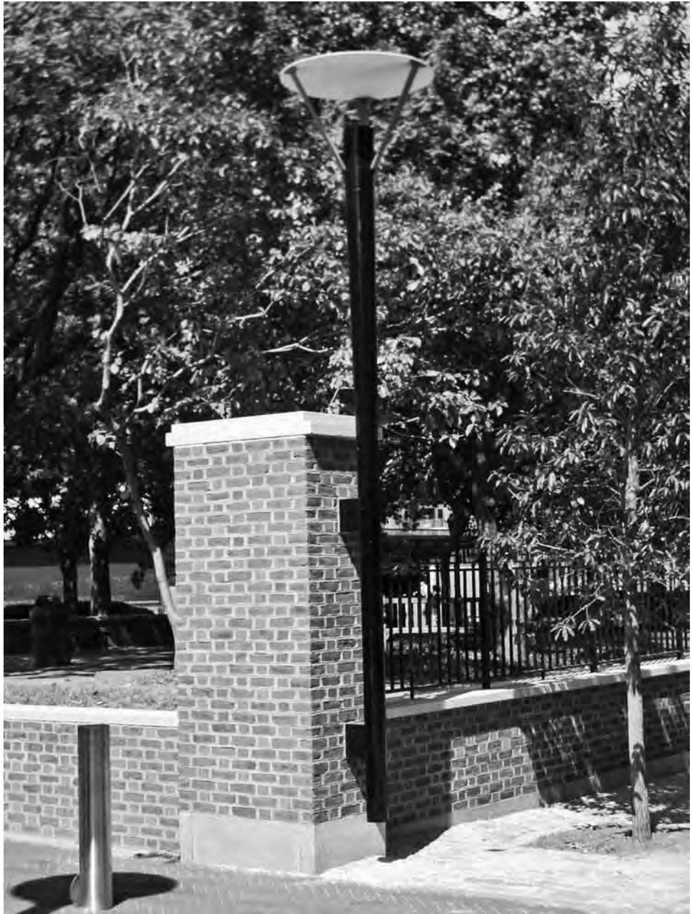
FIGURE 8-25b Completed wall and light standard are visible; existing parking structure, new structural system, and planting infrastructure are not visible.
