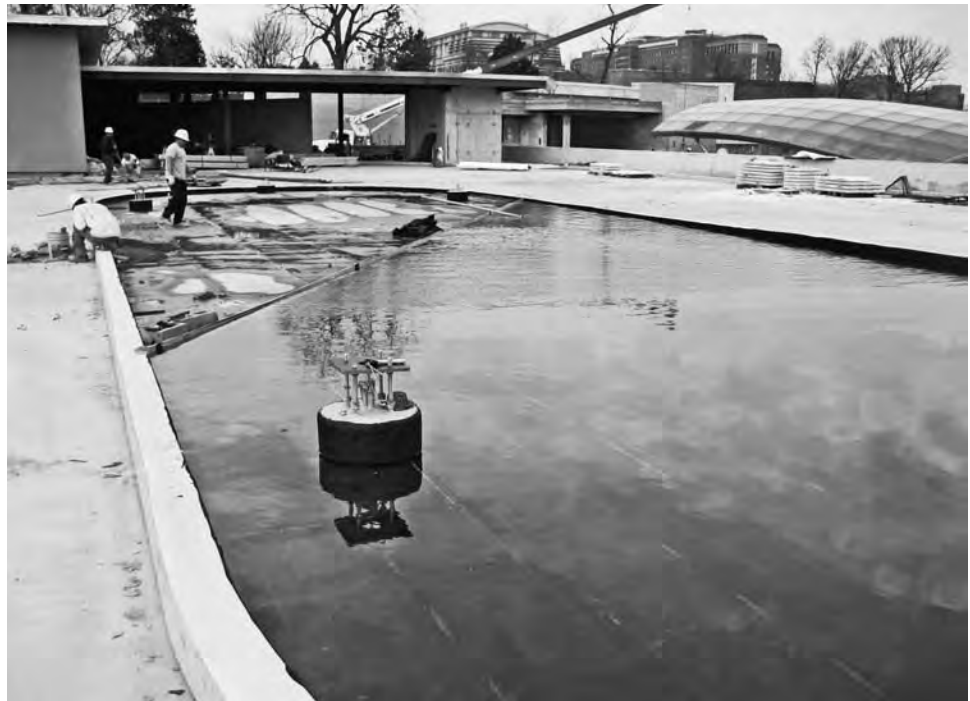
FIGURE 8-49 Flood testing of a waterproofed structural deck.
