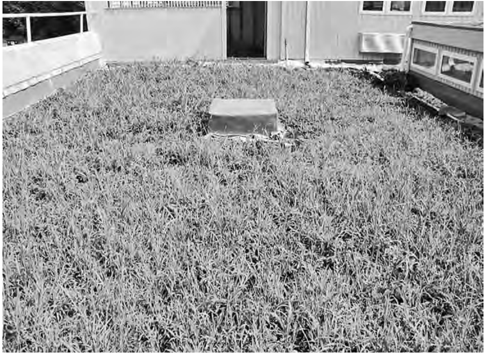
FIGURE 10-7a A living green roof overgrown with weeds.
