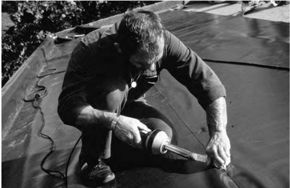
FIGURE 6-15 Heat-welding seams of waterproofing membrane. (Photo: re-natur, 24601 Ruhwinkel, Germany)
