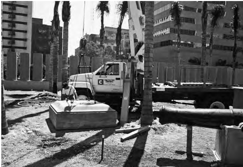
FIGURE 10-2a Construction sequencing and site access can dictate when trees must be installed, even when they can be easily damaged during the rest of construction.
