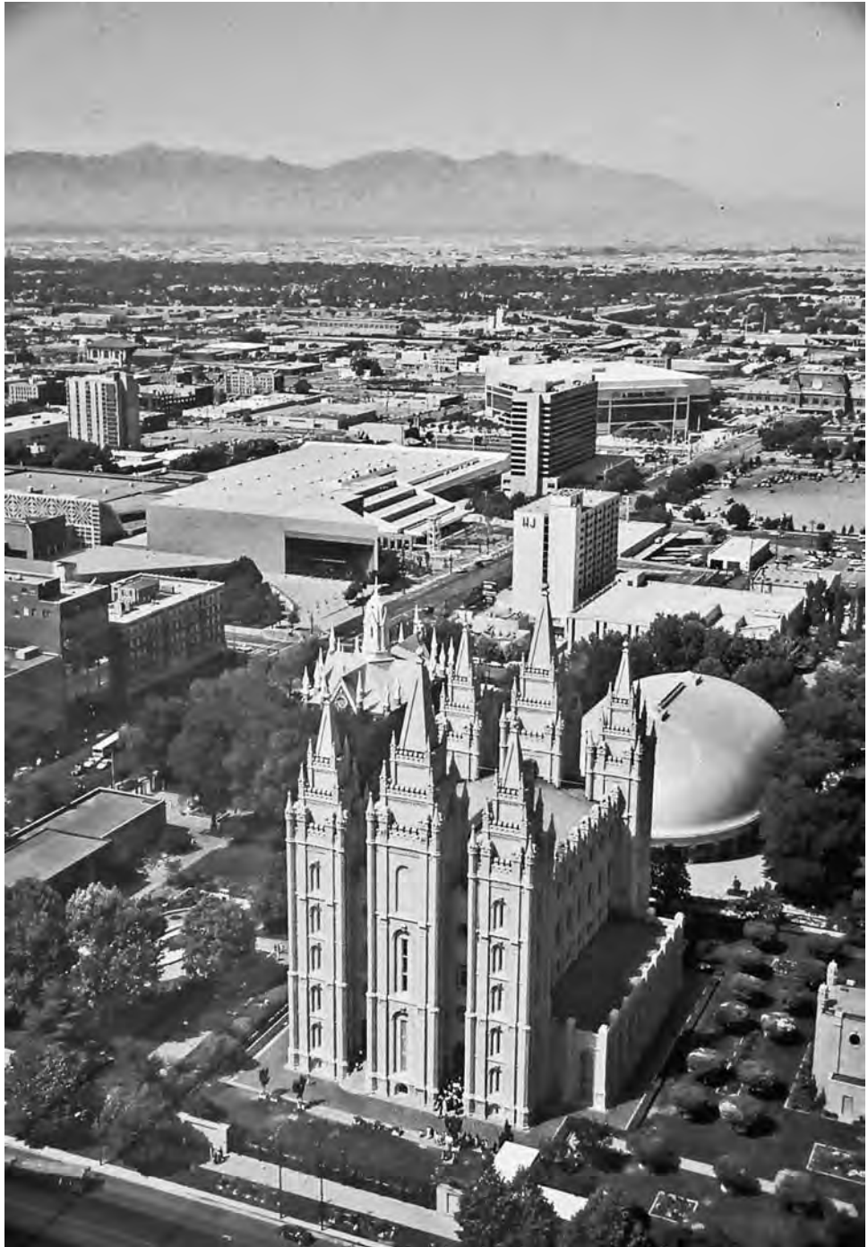
FIGURE 7-8 An overriding concern of the team was how to make a building this big reconcile itself with the Temple, the city, and the landscape beyond. (Photo courtesy of ZGF Architects)
