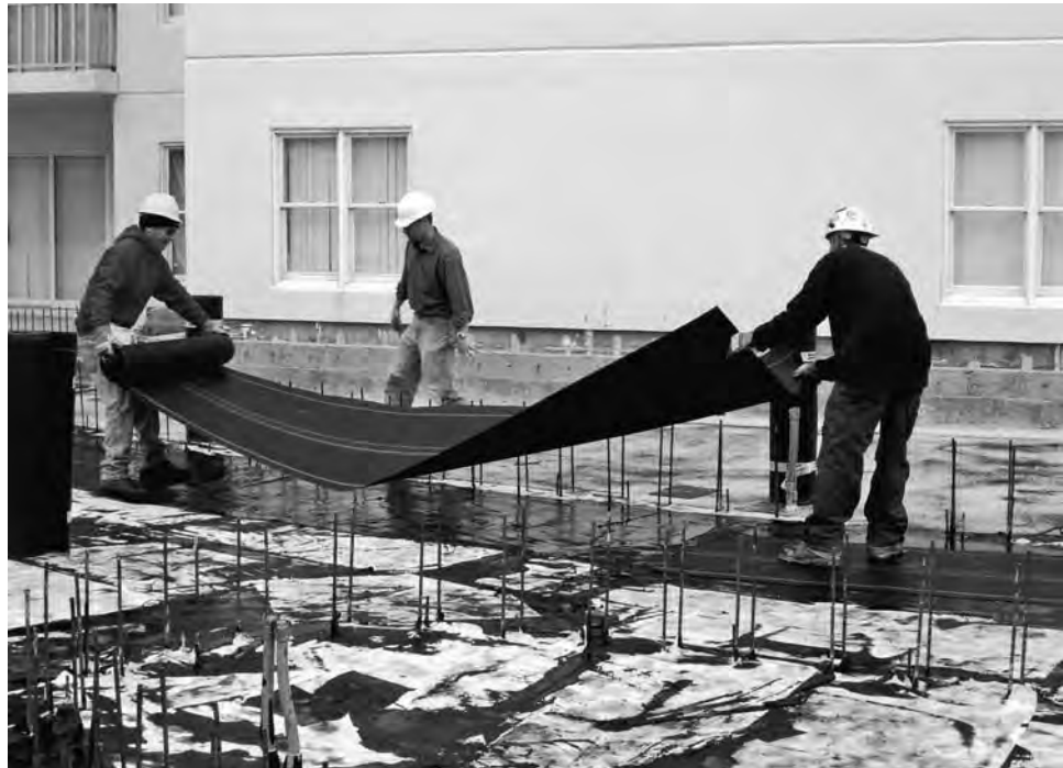
FIGURE 6-17 Application of membrane reinforcement. (Photo © Jeffrey L. Bruce & Co.)
