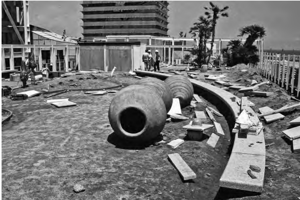
FIGURE 8-82 Completion of a landscape over structure often involves the coordinated installation of planting and site elements such as paving, walls, benches, and large-scale art elements.
