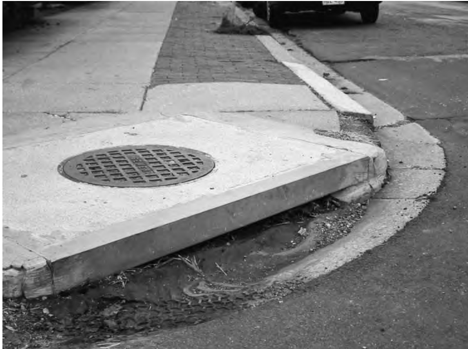
FIGURE 2-5 In addition to carrying surface pollutants from vehicles, stormwater runoff carries vast amounts of sediment to our sewers and eventually our waterways.
