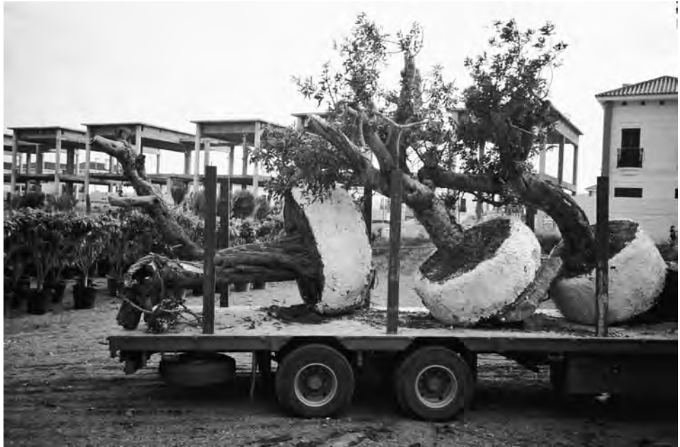
FIGURE 10-3a The contractor's responsibility for the care and protection of trees can start as early as their preparation at the nursery.
