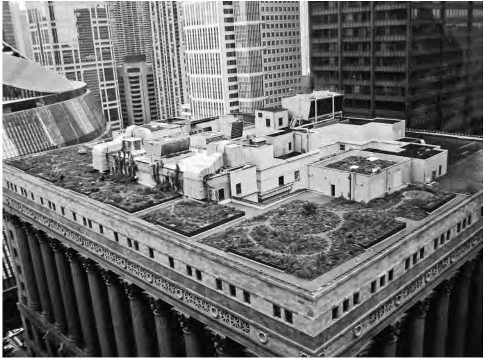
FIGURE 2-12 Chicago's City Hall green roof in contrast to adjacent black tar roof on other half of building.
