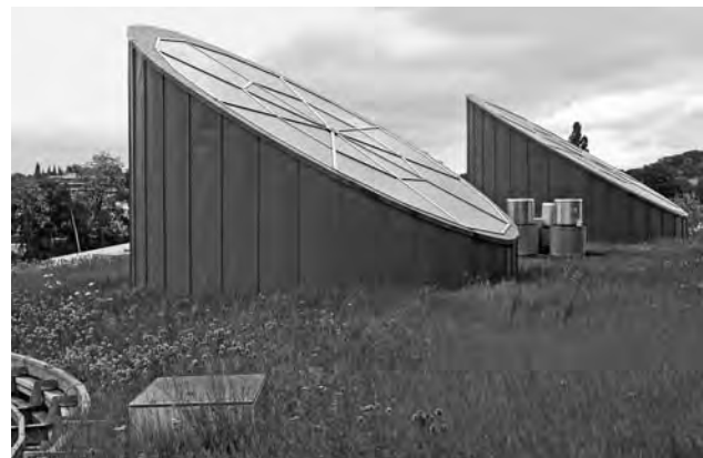
FIGURE 2-3 This living green roof has a 6-inch soil profile and is covered with a matrix of grasses. (Photo: Kai-Henrick Barth)
