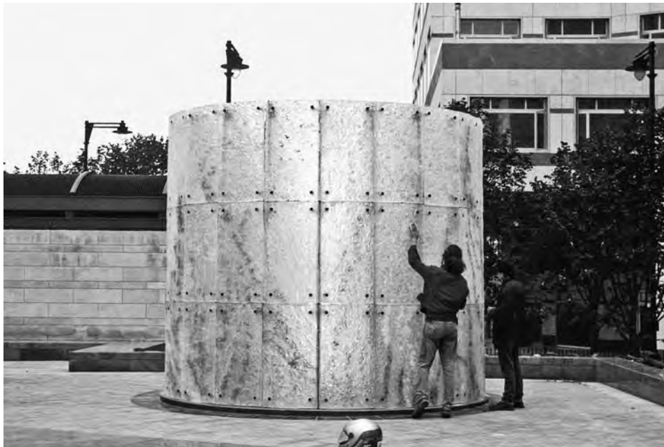
FIGURE 4-24 Working in collaboration with a glass artist, the project team integrated the ventilation shaft and equipment from the parking structure into the fountain design as part of a site-wide arts program.
