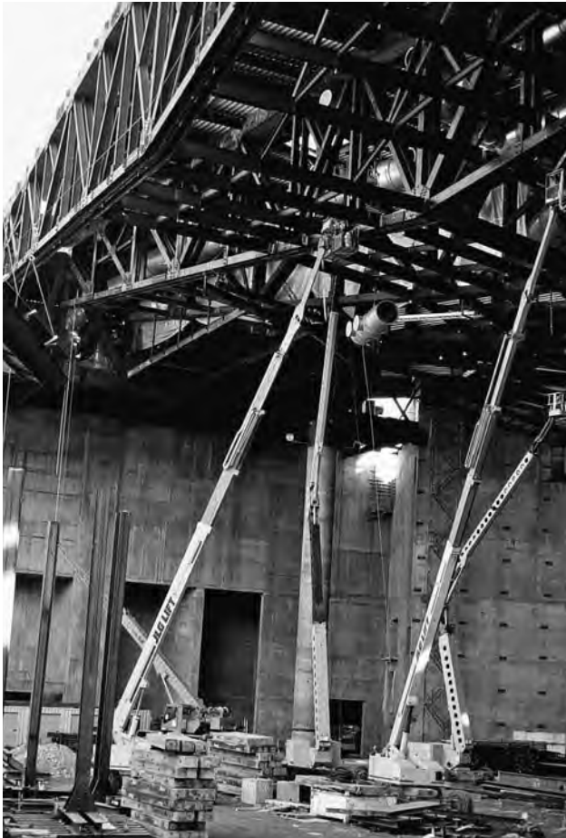
FIGURE 7-11 Loads and depths varied along the roof. (Photo courtesy of ZGF Architects)
