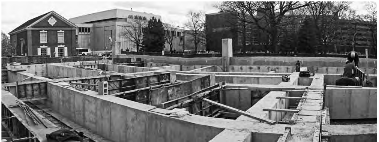
FIGURE 8-27 Concrete formwork and pouring of structural framing.
