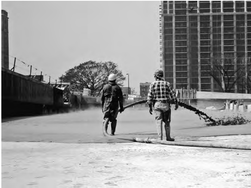
FIGURE 6-14 Pumping concrete for a topping slab. (Photo © Jeffrey L. Bruce & Co.)
