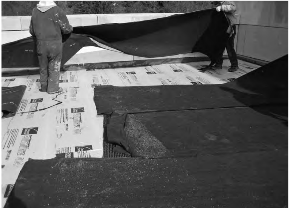
FIGURE 8-52 Removal of drainage system components in order to install correctly.
