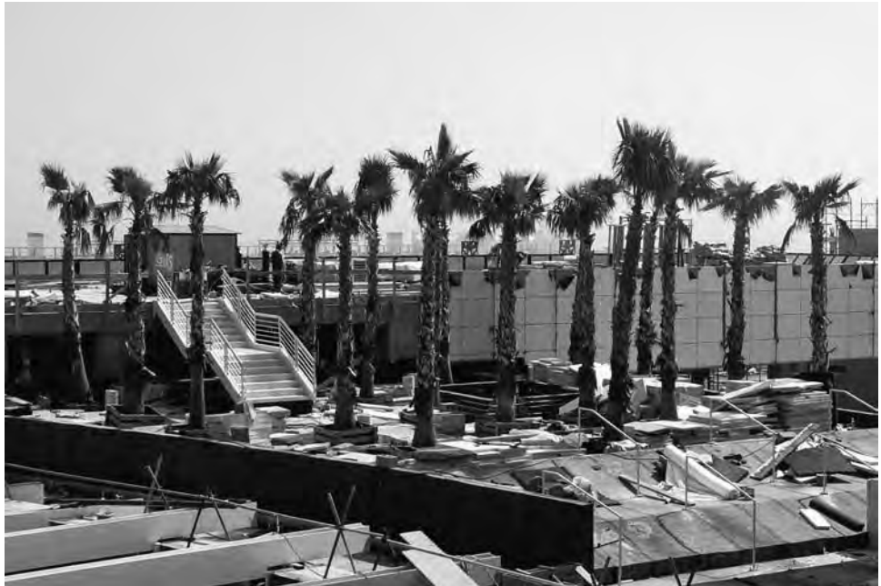
FIGURE 8-84a Installation of a palm grove.
