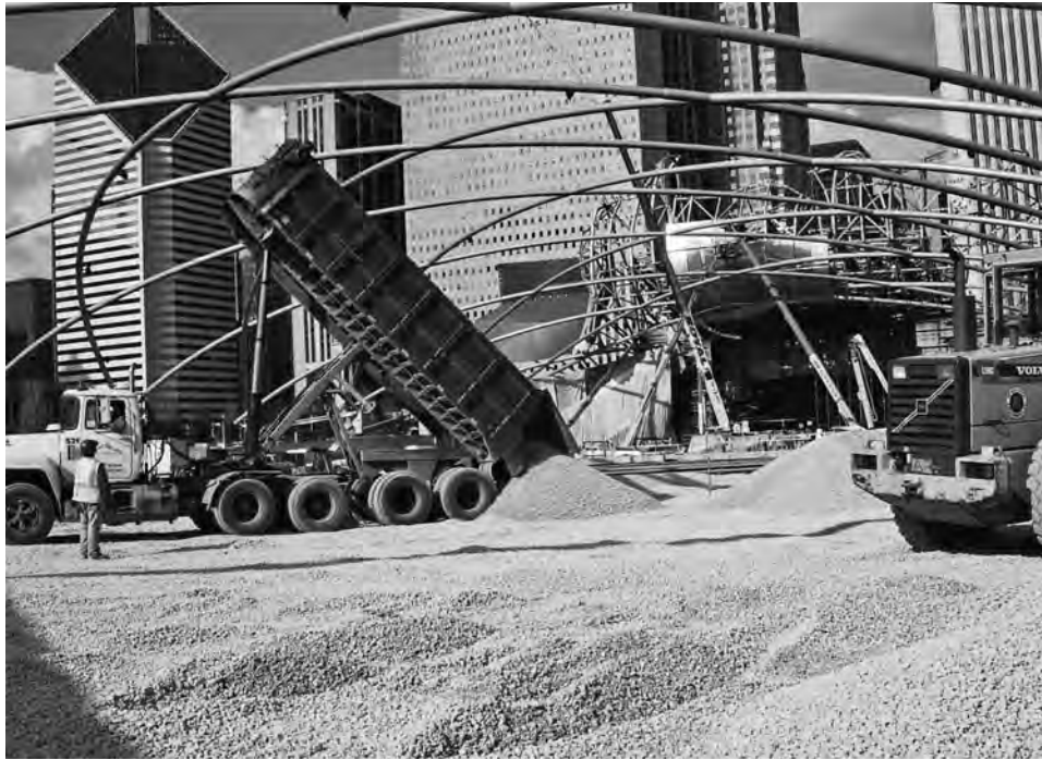
FIGURE 6-42c Installation of drainage aggregate. (Photo © Jeffrey L. Bruce & Co.)
