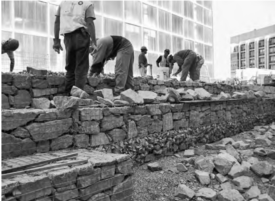
FIGURE 8-41 Construction sequencing required that these gabions be installed first. The gabions form a permeable shelved edge for the stormwater systems and were constructed on site. Note that the lowest level of the gabions is constructed with smaller aggregates. Smaller aggregates provide a graded system for the settling out of stormwater particulates.
