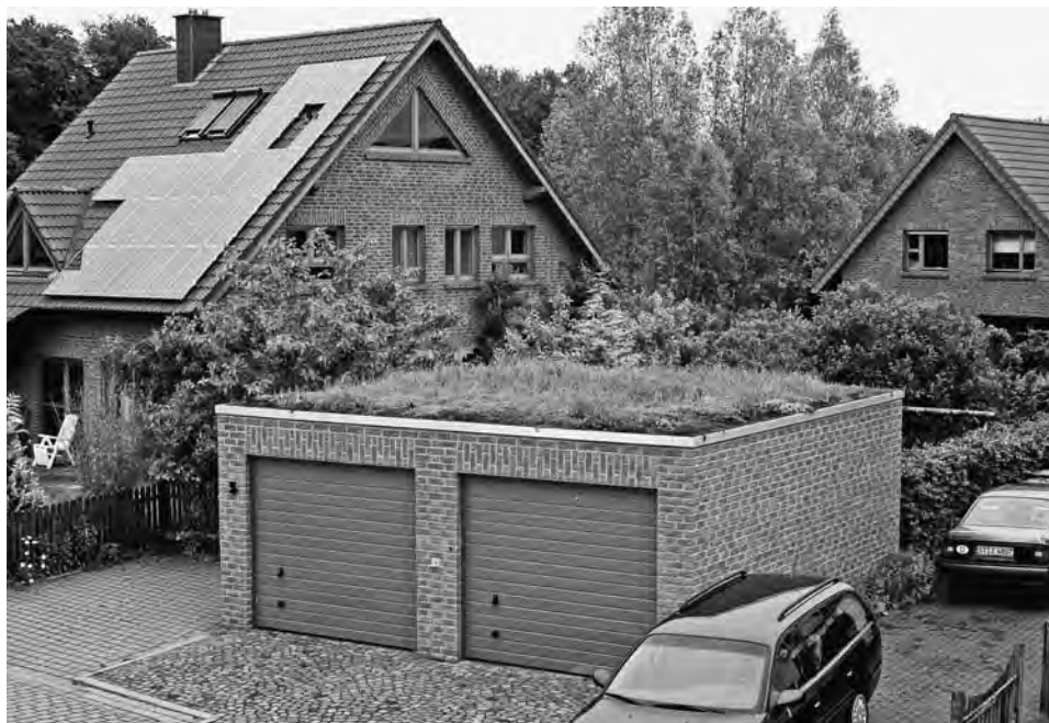
FIGURE 2-7 Living green roofs can be effective on a residential scale and provide visual continuity to the neighborhood setting. (Photo: Kai-Henrik Barth)
