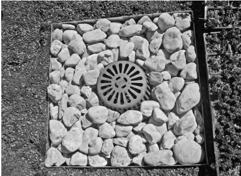
FIGURE 8-54 Drain collar installation. Drainage gravel surrounds the drainage opening for this living green roof to help ensure the free flow of excess stormwater. Growing medium is then installed around the collar.
