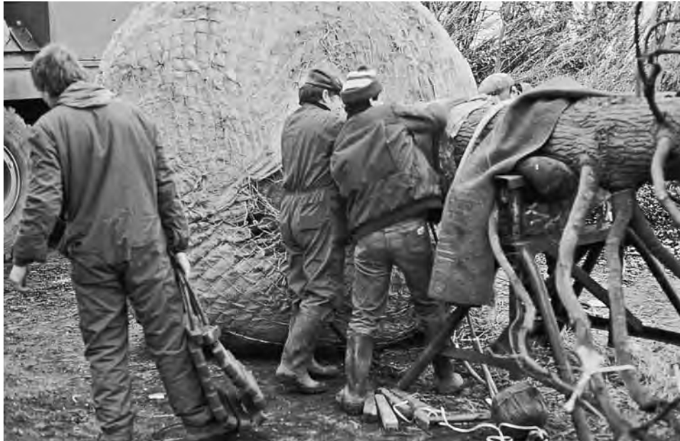
FIGURE 4-7 Installation of very-large-caliper trees in below-grade planters. The radial pattern reflects road circulation, building and open space configuration at finished grade.
