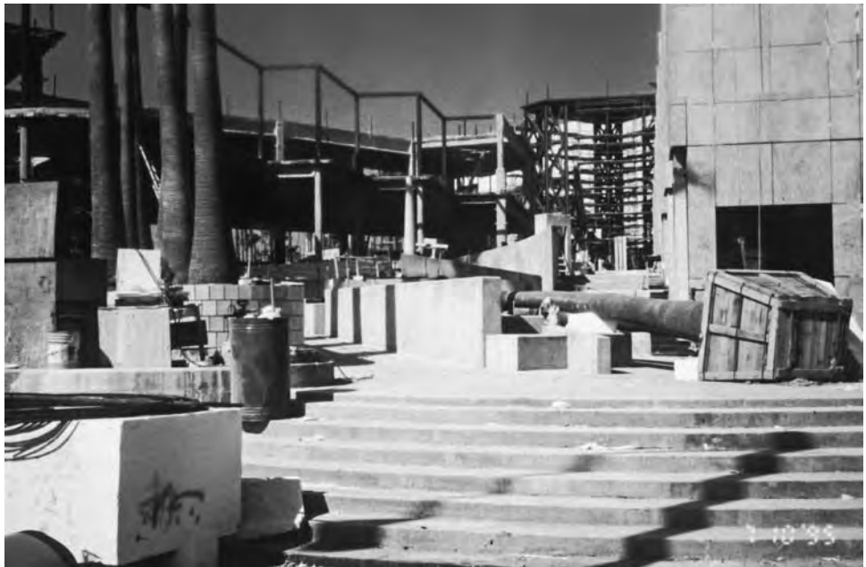
FIGURE 8-70 Palms in boxes were installed early in the site construction process.
