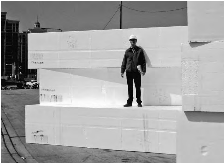
FIGURE 6-24 EPs blocks for lightweight fill over structural deck. (Photo © Jeffrey L. Bruce & Co.)
