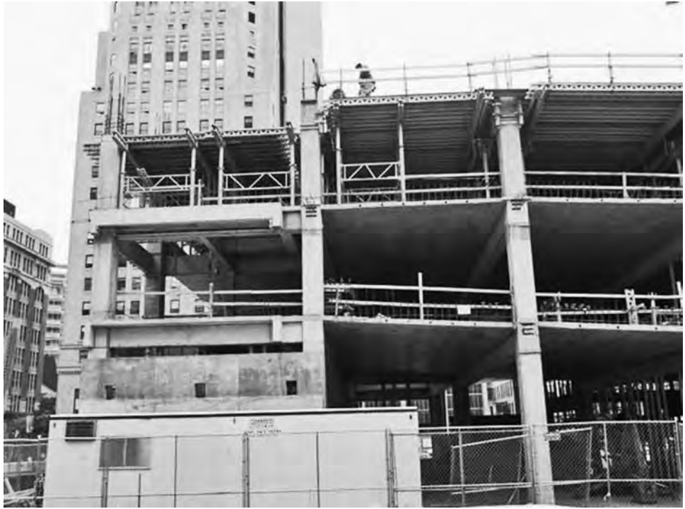
FIGURE 6-12 Achieving slope of a structural deck.
