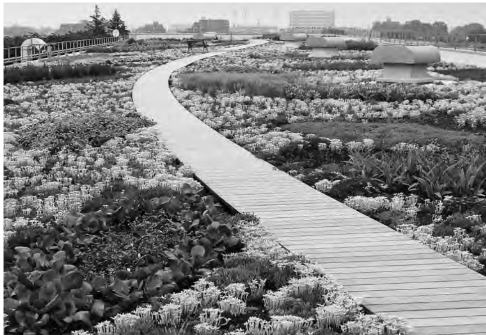
FIGURE 6-38 This simple boardwalk shows a clear demarcation between accessible walking surface and the part of the living green roof not intended for access and dynamic load. (Photo © Zinco)
