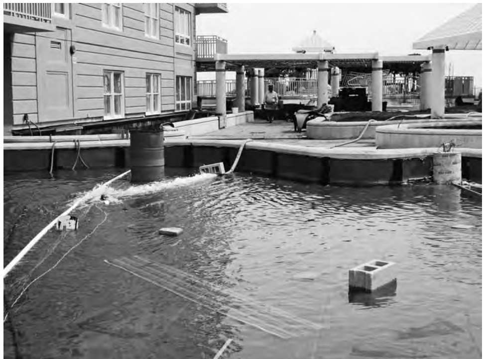
FIGURE 6-18 Flood testing of waterproofing membrane. (Photo © Jeffrey L. Bruce & Co.)
