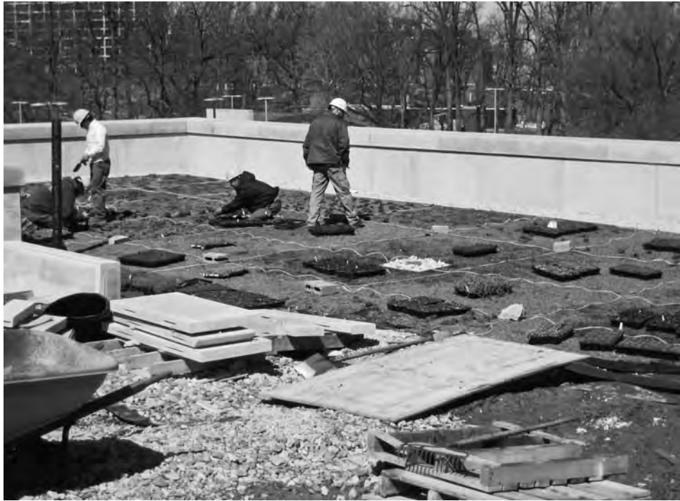
FIGURE 8-81 Installation of plants on living green roofs.
