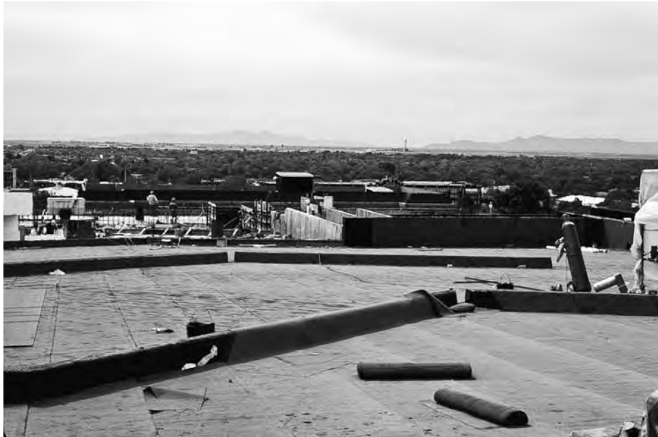
FIGURE 6-21 Installation of protection board over multiple surfaces.
