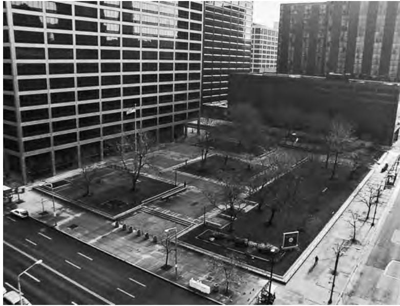
FIGURE 4-16 Existing conditions of buildings and an underutilized plaza in Cleveland.
