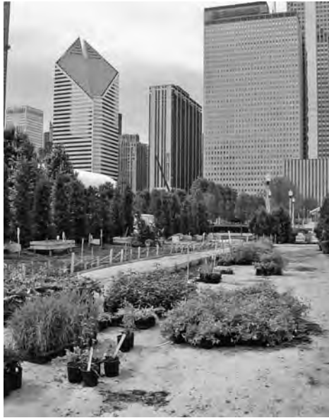
FIGURE 8-78 Construction staging required on-time delivery, suitable storage, and careful handling of plants on site. (Photo © Jeffrey L. Bruce & Company)
