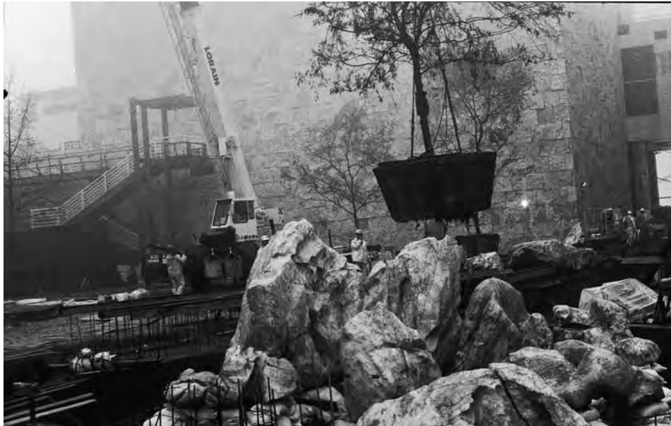
FIGURE 8-85 Boulders selected from the nearby Sierra Nevada were carefully placed on the site. Trees (in boxes) were installed subsequently.
