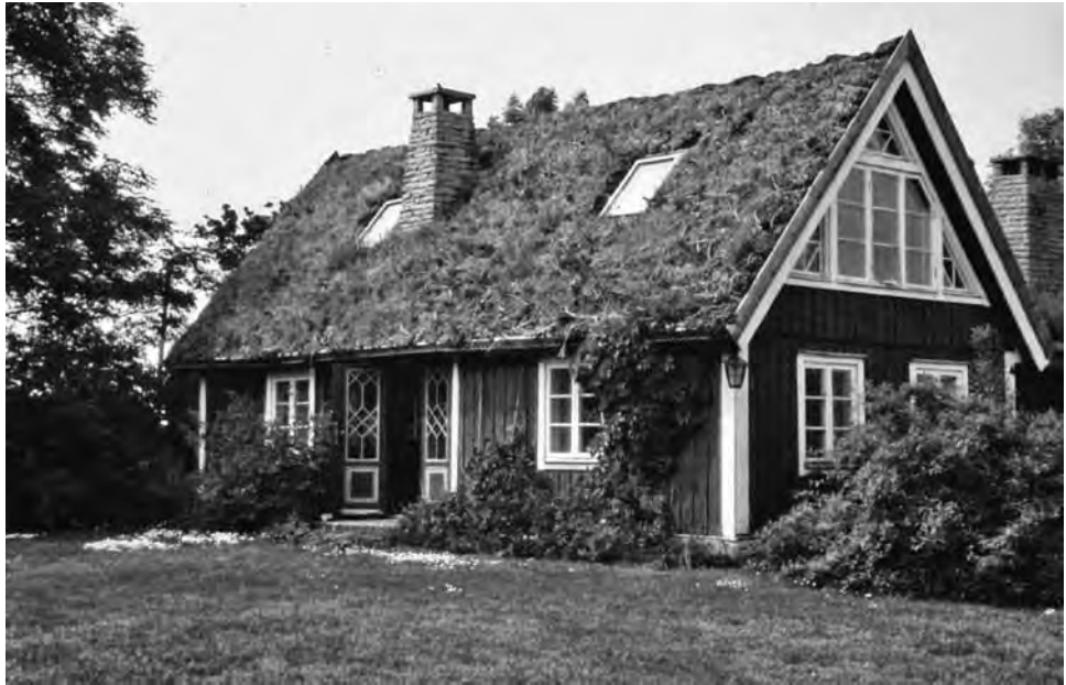
FIGURE 6-6 Steeply sloped roof with a living green roof application. (Photo by re-natur, Germany)
