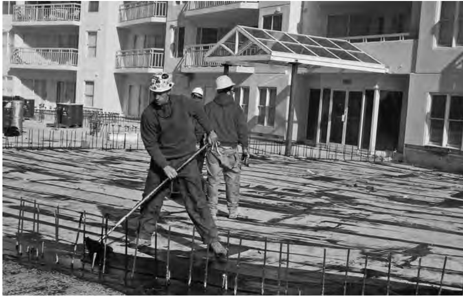
FIGURE 6-16 Hot-mopping of rubberized asphalt membrane. (Photo © Jeffrey L. Bruce & Co.)
