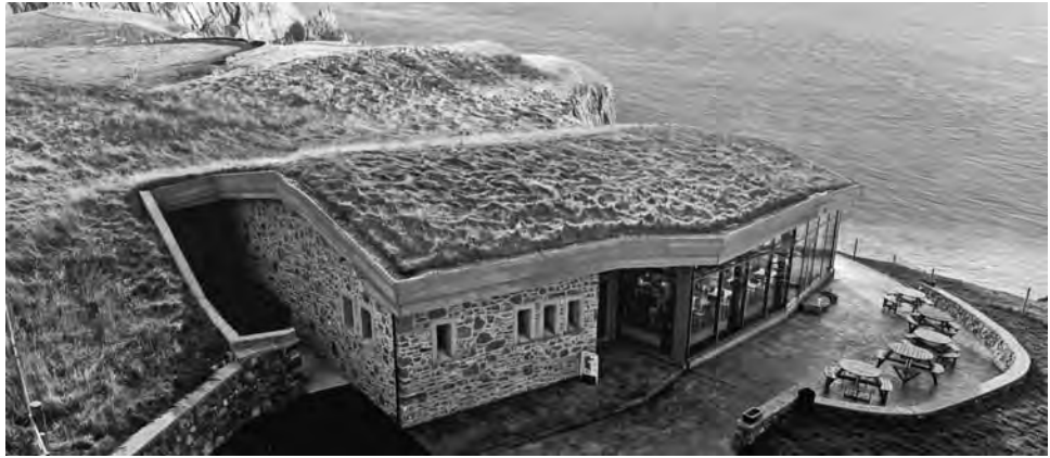
FIGURE 4-3 This use of a living green roof, although not accessible to human use, keeps the view of the natural landscape intact. (Photo: © Zinco)
