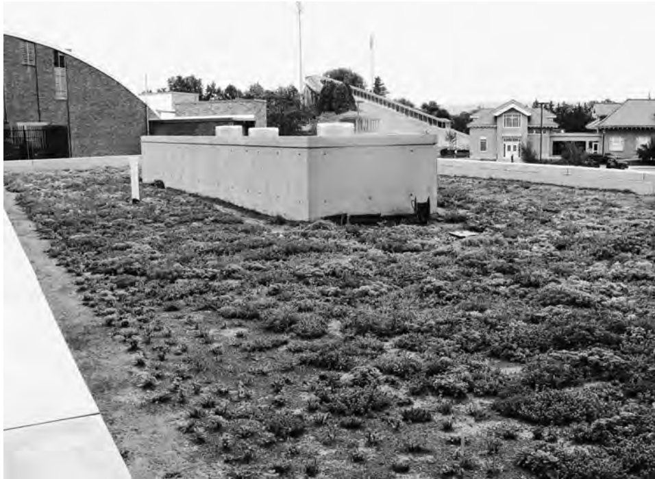
FIGURE 10-5a A freshly installed living green roof.
