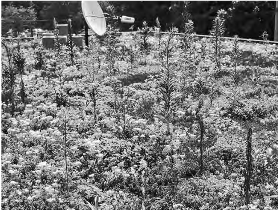
FIGURE 10-8 Despite the well-established living green roof plant cover, weed seeds embedded in the growing medium sprouted and need to be removed meticulously. Here, Canadian horseweed ( Conyza canadensis ), which can spread widely via windblown seeds, fortunately can be pulled easily.
