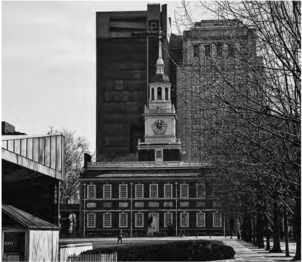
FIGURE 8-20 Existing conditions at the Liberty Bell Pavilion.
