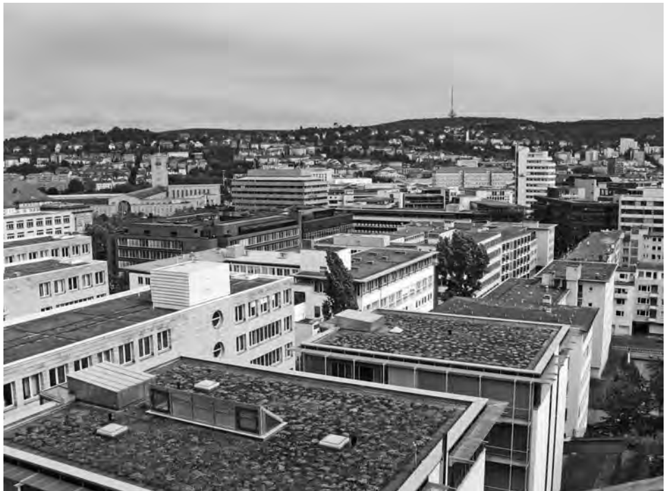
FIGURE 4-4 The city of Stuttgart has had some of the most effective municipal green roof requirements and incentives in Germany since the 1970s; now living green roofs are common in the urban landscape. (Photo: © Zinco)
