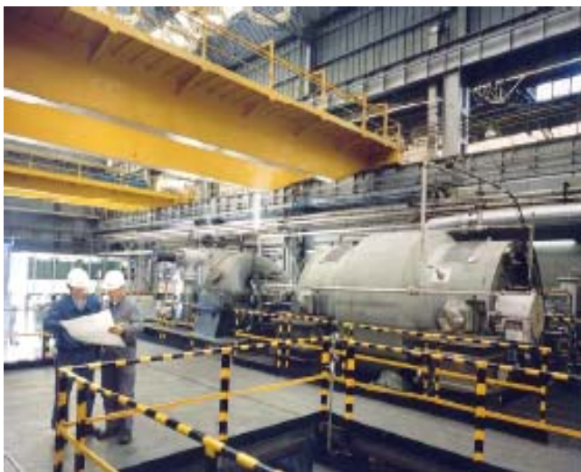
Figure 80. Indoor Test Stand.
