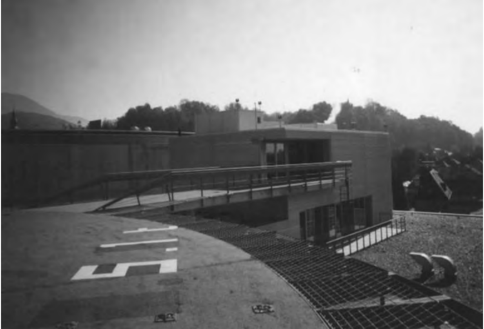
Figure 18-8 Electrically heated pavement - emergency heliport on the roof of the regional hospital at Salzburg, (Photo: A. Kazda)
