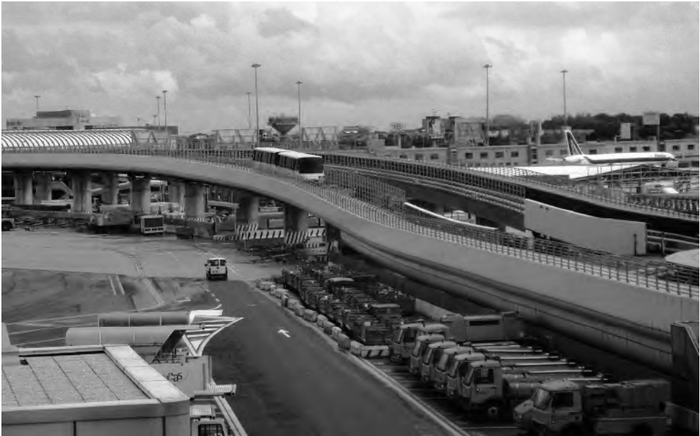
Figure 12-15 People mover system, shuttle type, connecting airport buildings at Roma – Fiumicino (Photo: A. Kazda)
