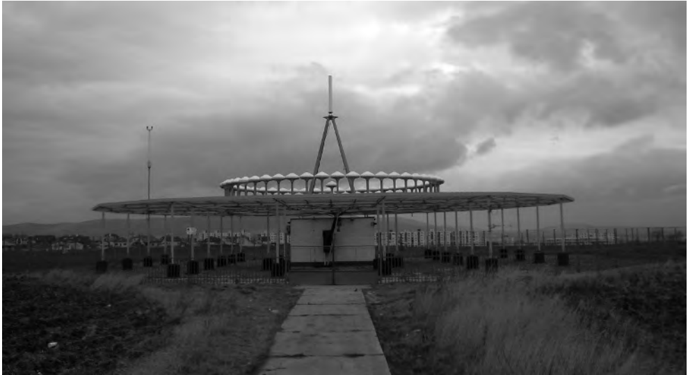
Figure 17-6 D-VOR/DME ground station Nitra
