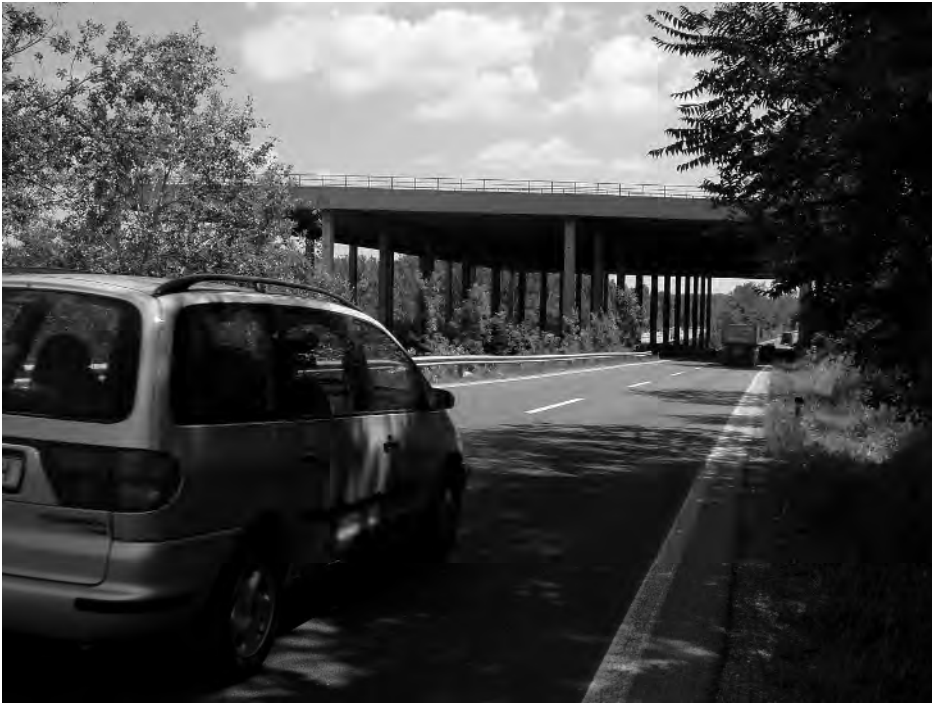
Figure 5-2 Large constructions are sometimes necessary to guarantee runway strip dimensions – Vienna Airport (Photo: A. Kazda)
