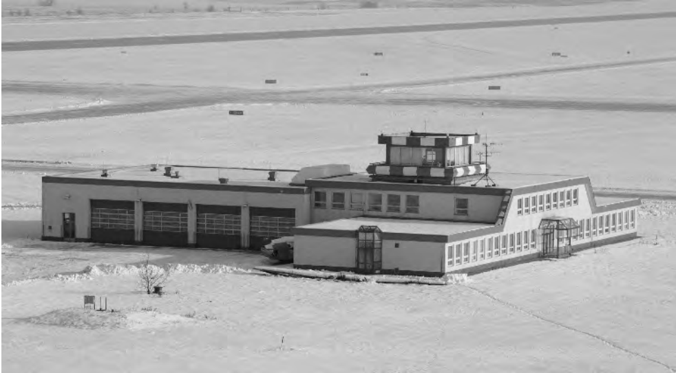
Figure 19-6 A fire station should be located in the centre of runway system (Photo: Courtesy of Bratislava M.R. Štefánik Airport)
