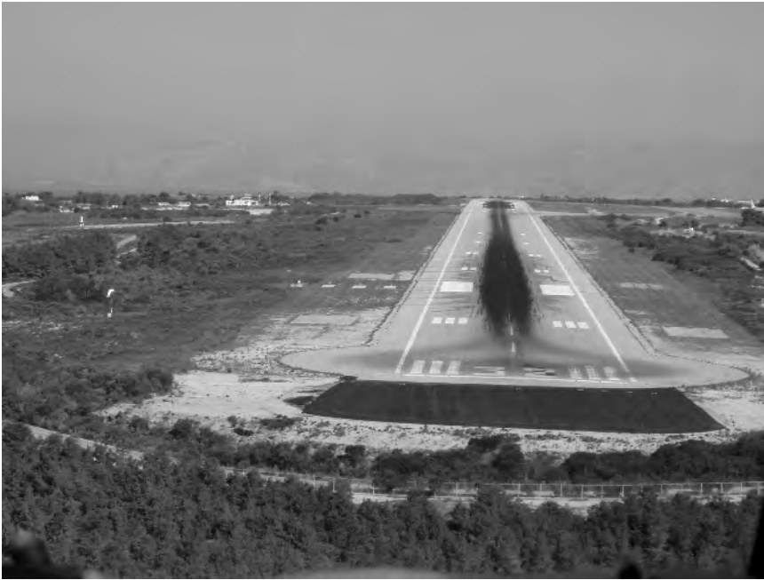
Figure 4-15 Turn pad at the runway end
