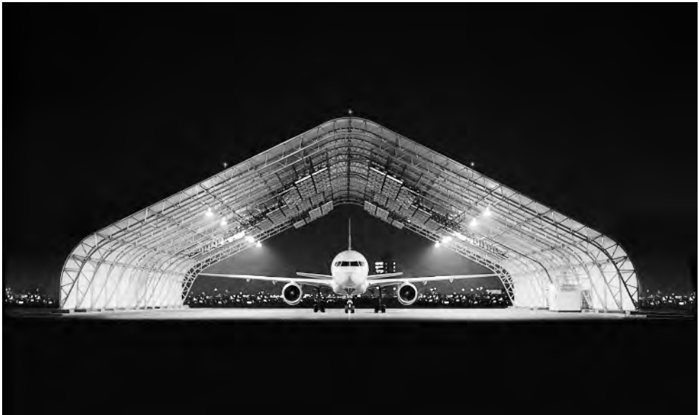
Figure 18-13 InfraTek de-icing facility of Radiant Aviation Services – RAS (Photo: Courtesy Oslo Airport)
