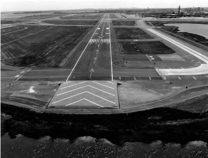
Figure 5-5 EMAS installation at Boston Logan Airport, courtesy ESCO ZODIAC Company
