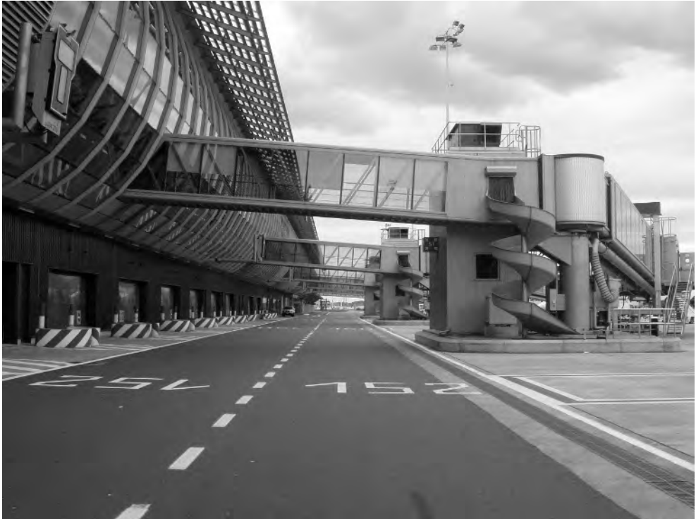
Figure 9-5 A part of the passenger boarding bridge crosses the service road (Photo: A. Kazda)
