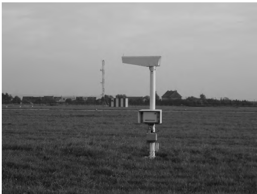
Figure 3-4 Part of RVR equipment in touchdown zone (ILS GP antenna behind) (Photo: A. Kazda)
