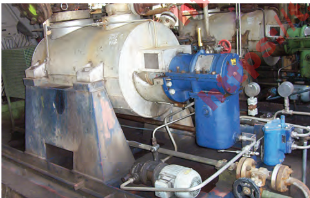
Figure 15. Barrel Pump at Site after Retrofit.
