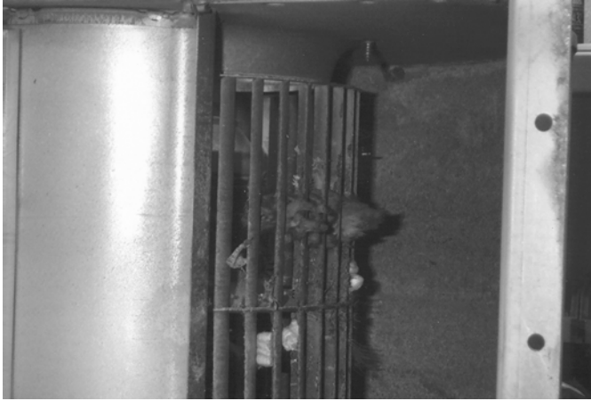
Figure 7-5. Foreign object in fan (Courtesy of ABB Inc.)
