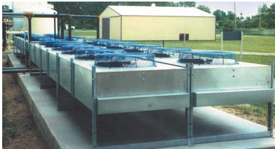
Fig. 3 — Air-cooled tower with top fans.
