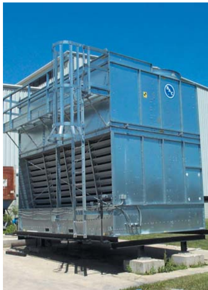
Fig. 6 — Counter-flow closed-loop pressurized evaporative cooling tower; requires a pan heater.
