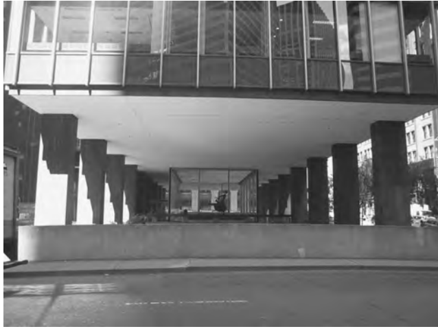
Figure 10.9 Example of column freely exposed to public access. The column supports the corner of a high-rise building.
