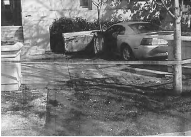
Figure 12.16 Concrete Planter Penetration
