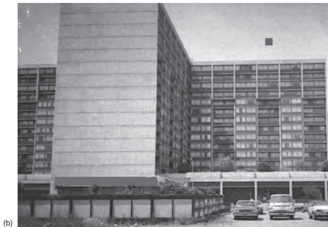
Figure 10.12 Reentrant corner plans: (a) Some plan types. (b) T-shaped building with two reentrant corners.
