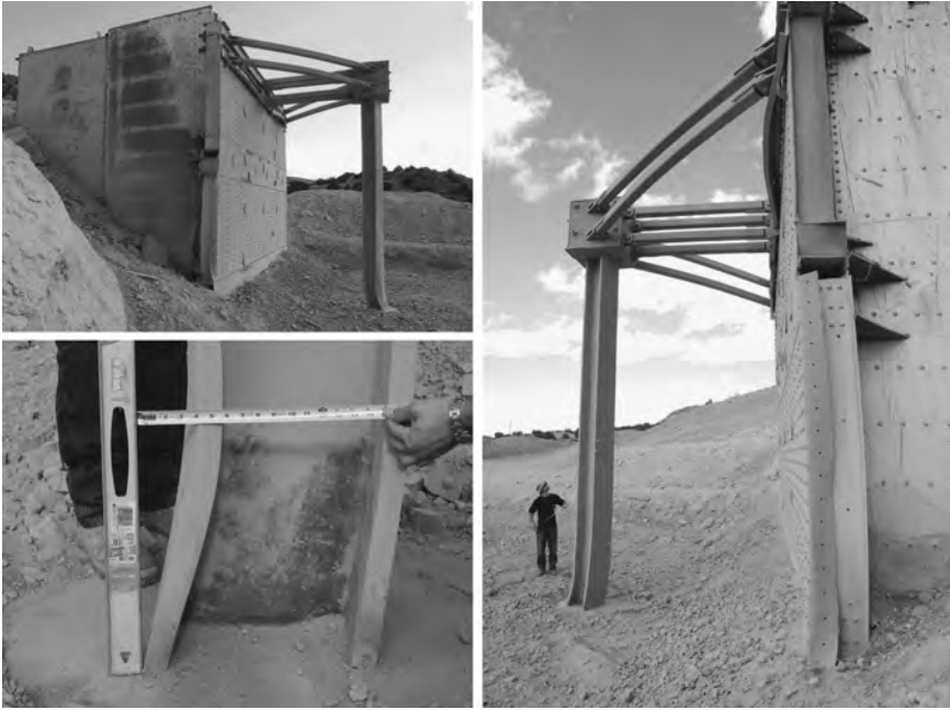
Figure 4.5 Steel Cross Section Distorted Due to Air-Blast Loading (Courtesy of American Institute of Steel Construction)
