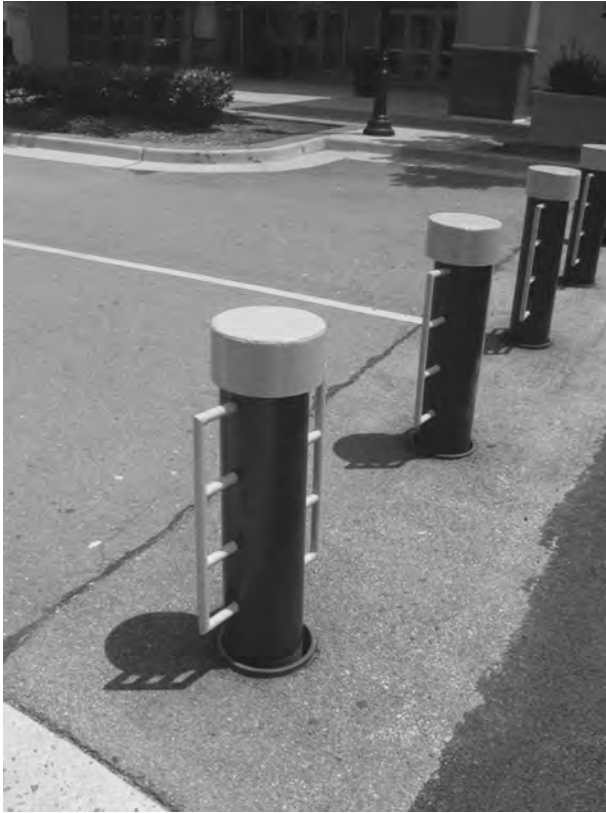
Figure 12.10 Removable Bollard
