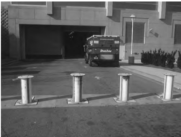
Figure 12.11 Operable (Pop-Up) Bollards
