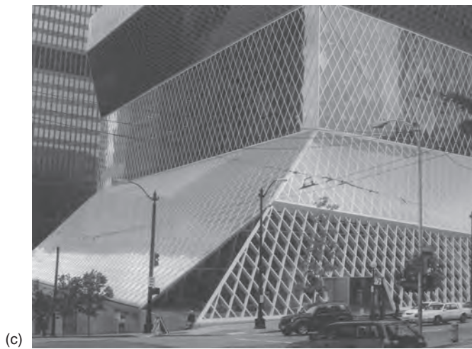
Figure 10.5 Types of Metal and Glass Curtain Walls. (a) Curtain wall framing expressing main building structure. (b) Uniform curtain wall framing over the façade. (c) curtain wall framing draped over rectilinear building forms.
