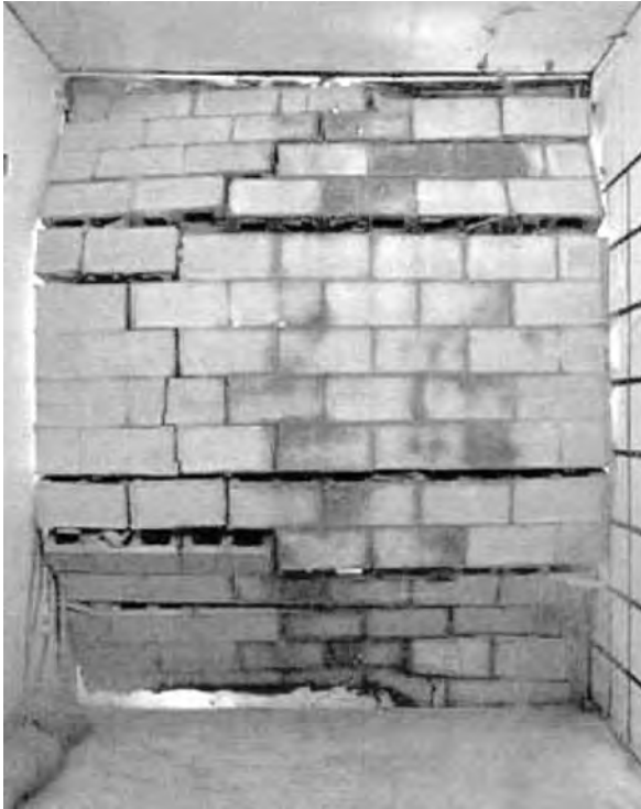
Figure 17.10 Example typical of the response expected from a CMU wall struck by a blast; at the time shown, the CMU is moving at several tens of feet per second (Photo courtesy of The Energetic Materials and Research Testing Center)
