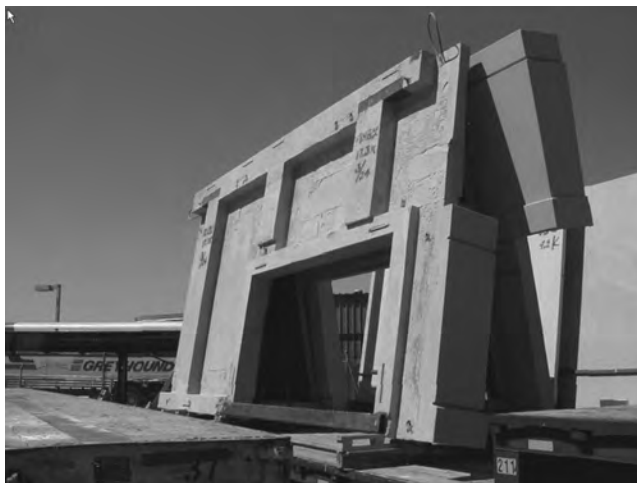
Figure 10.8 Precast Concrete Ribbed Wall Panels
