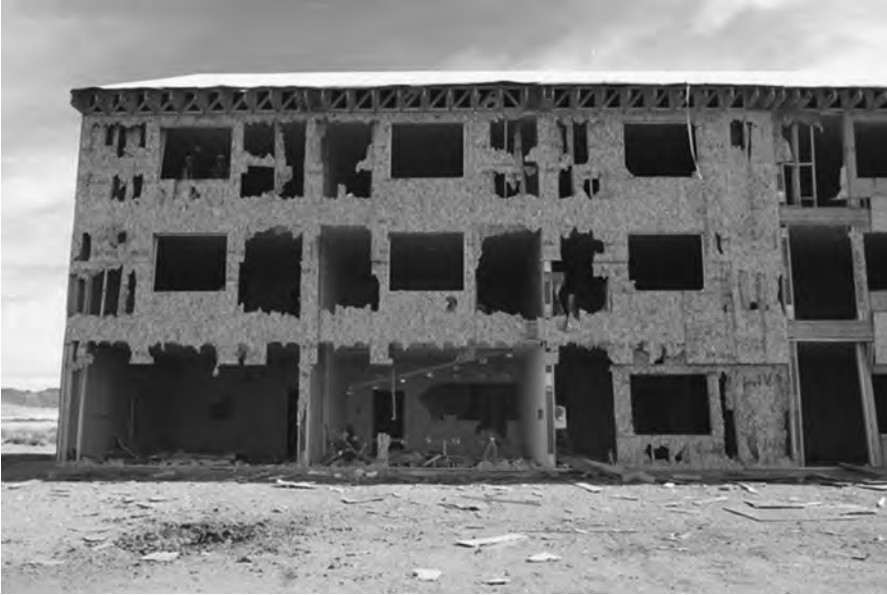
Figure 5.2 Full-Scale Building Testing
