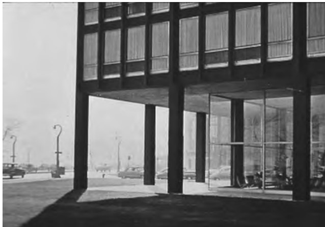
Figure 10.10 Example of public walkway beneath second floor of high-rise building
