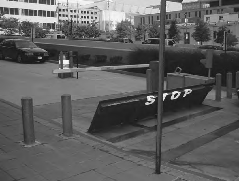
Figure 12.12 Wedge Barrier
