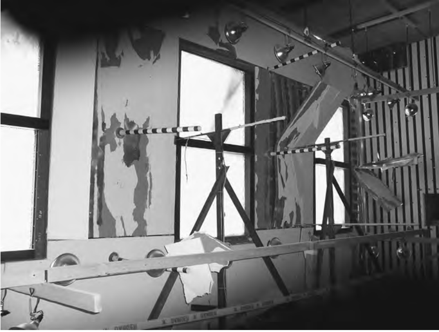
Figure 5.4 Digital Photography and Deflectio Measurement
