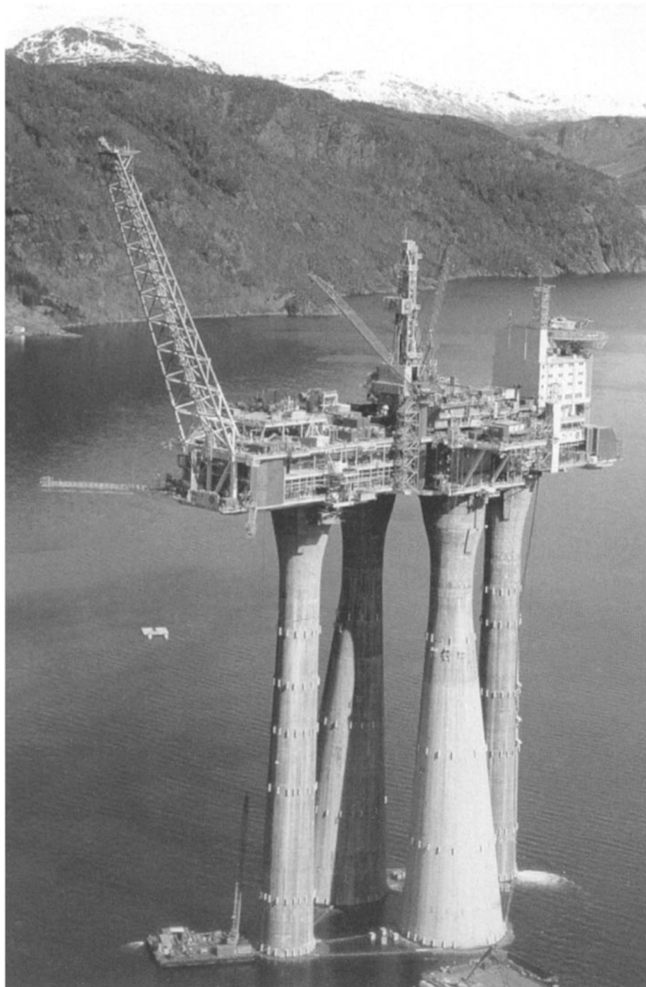
Fig. 1.2 Troll Gas, the largest platform of the CONDEEP type (by courtesy of Aker Maritime)
