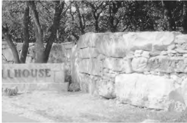
Figure 10-24 Dry-stack wall with large and small stones.
