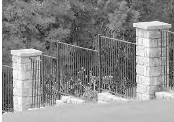
Figure 10-22 Allow for expansion and contraction of metal between masonry piers.
