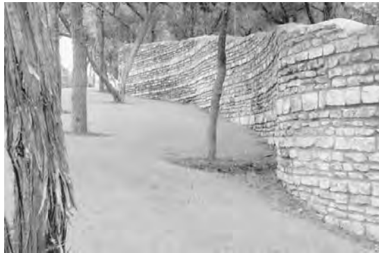
Figure 10-25 Mortared stone walls.
