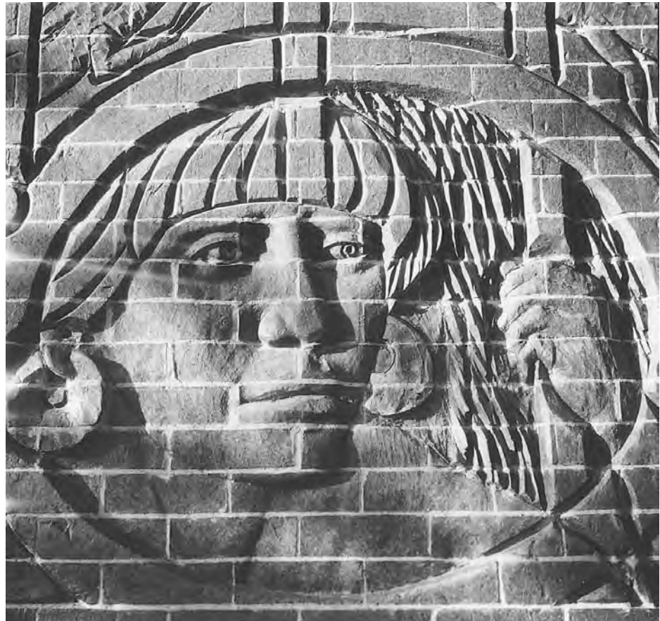
Figure 3-9 Sculptured brick is carved by the artist before the brick is fired. (Photo courtesy BIA.)
