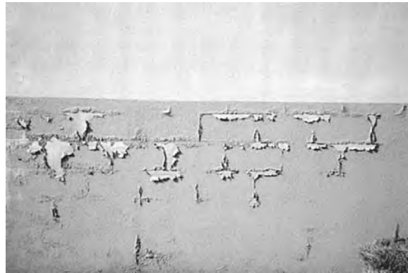
delamination of exterior coating
