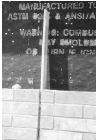
Figure 15-41 Remove boards or other non-compressible fillers used to keep mortar and debris out of expansion joints during construction.
