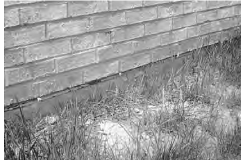
Figure 15-35 Cotton rope wicks spaced 16 in. on center. (Photos courtesy BIA.)
