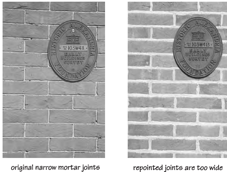
Figure 16-10 Original (left) and repointed (right) halves of building have very different appearance.
