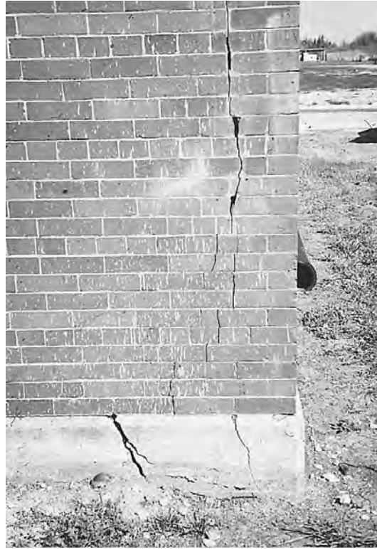
Figure 9-6 Opposing moisture expansion of brick and curing shrinkage of concrete slab can cause cracking at building corners if differential movement is not accommodated.
