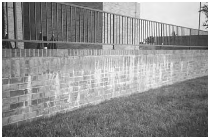
Figure 16-5 Calcium carbonate stain.
