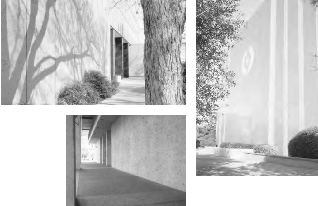
Figure 5-12 Stone veneer slabs.
