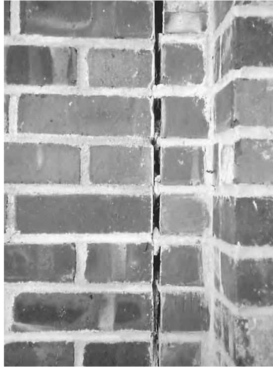
Figure 9-14 Mortar bridges across an expansion joint can cause localized spalling where movement is restricted.
