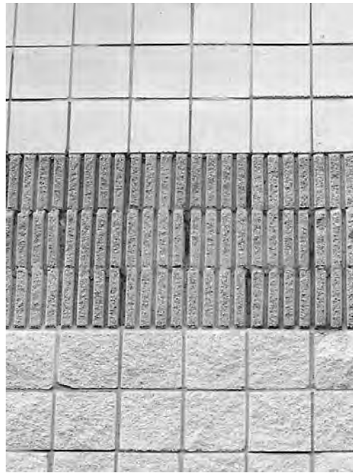
Figure 2-9 Smooth, split-ribbed, and split-faced concrete block.
