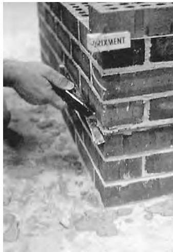
Figure 15-30 Trim flexible flashing flush with outside face of wall. (Photo courtesy BIA.)
