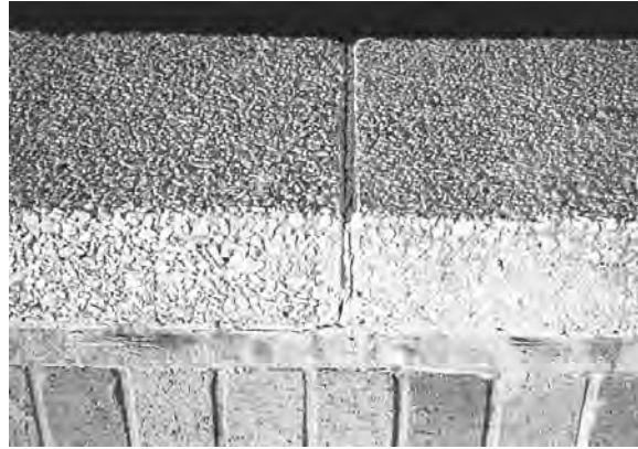
Figure 9-50 Rake out mortar joints in masonry copings and fill with bond breaker tape and elastomeric sealant to prevent water penetration through shrinkage cracks in mortar joints.
