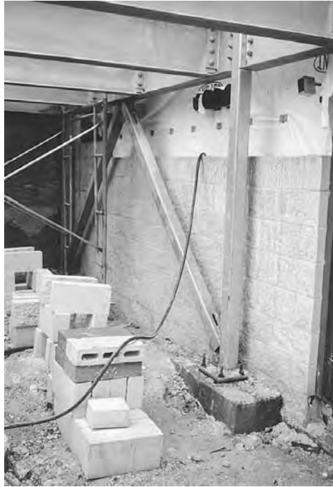
Figure 18-3 Garden hose placed briefly in wall cavity to test for obstruction of water flow to weeps.
