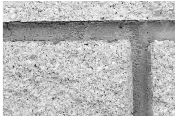
rough surface, bond line separations
