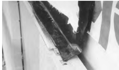
Figure 9-33 Lap moisture-resistant membrane over flashing.
