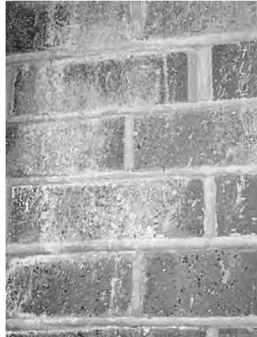
Figure 16-2 Efflorescence.
