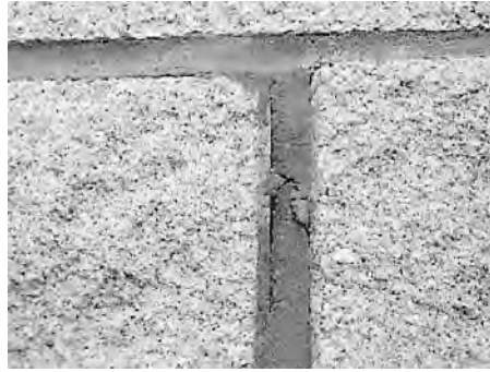
void in exterior mortar joint caused by poor workmanship
