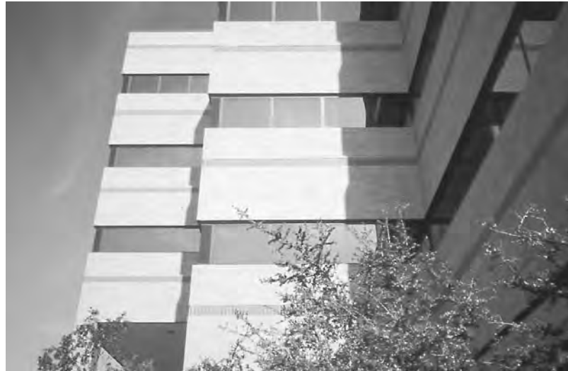
Figure 10-65 Strong horizontal color bands disguise wide soft joints at shelf angles.
