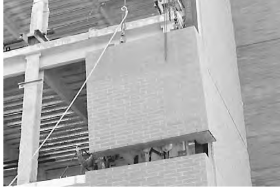
Figure 15-59 Lifting a prefabricated masonry panel into place.
