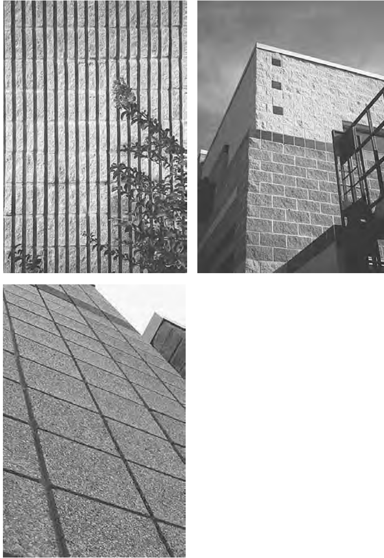
Figure 4-11 Ribbed, split-face, and burnished concrete block.
