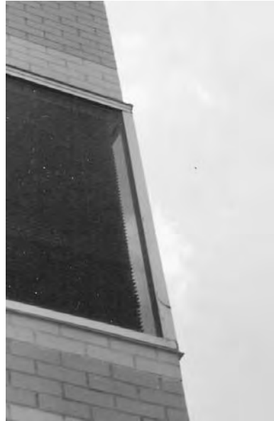
Figure 9-40 Protruding window invites leaks at head.
