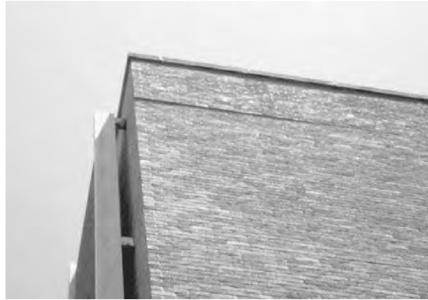
Figure 9-7 Parapets can expand and contract at a different rate than the building walls below.
