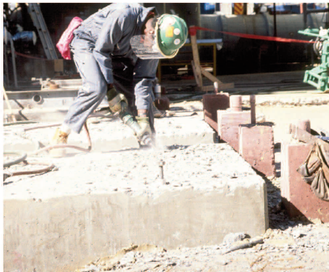
Figure 5. Exposing Aggregate.
