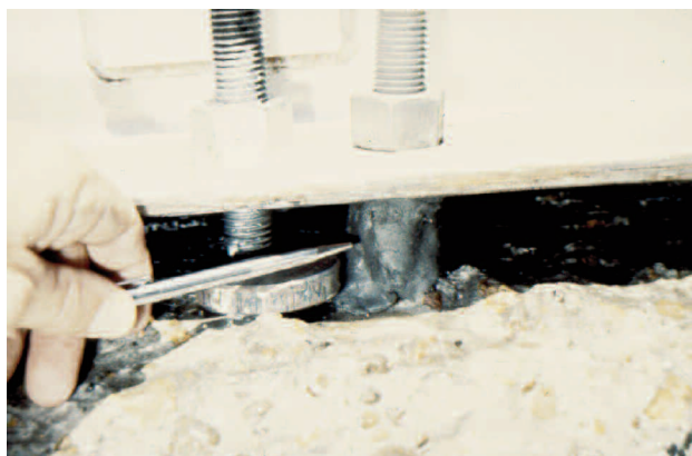
Figure 7. Wrapped Exposed Length of Anchor Bolt.
