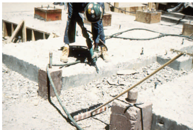
Figure 6. Chamfering of Foundation Edges.
