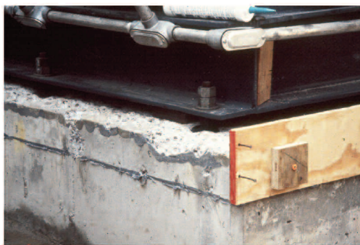
Figure 18. Form Design for a Two-Pour Method.
