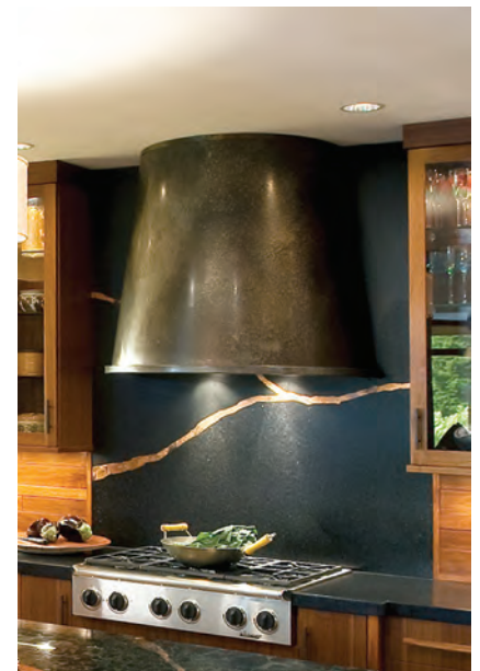
FIGURE 8.41 Overhead ventilation with eased and curved edges reduces the risk of head bumps for users who are tall or who have issues with vision.
