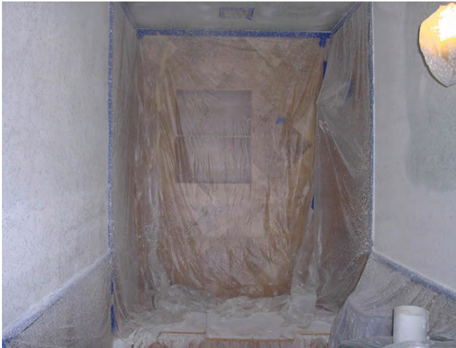
FIGURE 3.12 Plastic sheeting is essential for isolating the workspace from the living area.
