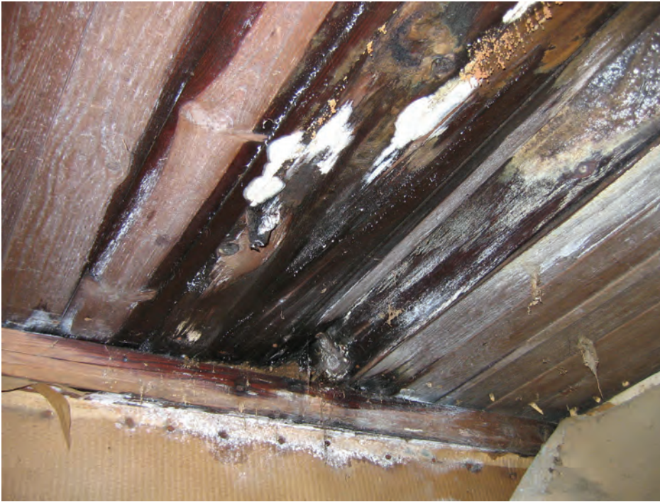
FIGURE 3.14 Growth of various types of mold on wood under flooring.
