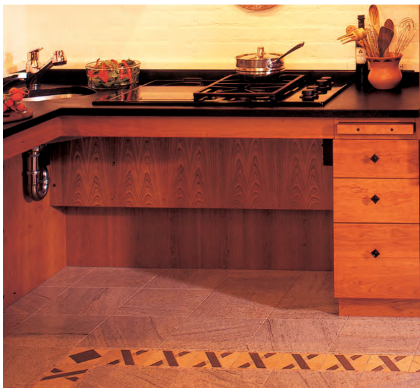
FIGURE 8.32 Side controls on the cooktop, a sink to one side, and a generous knee space improve access and function.
