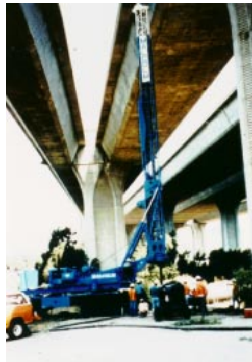
Figure 6-8: Drill Rig – Truck Mounted
