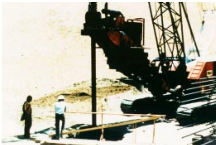
Figure 6-9: Drill Rig – Crane Mounted
