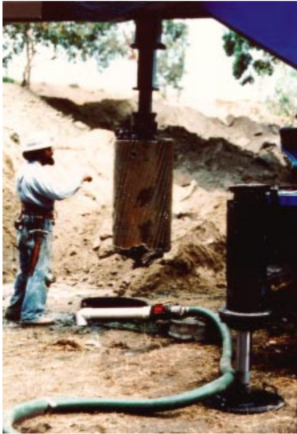
Figure 6-4: Drilling Bucket
