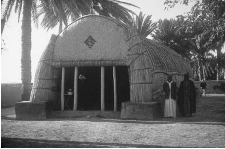
FIGURE 6. Arched reed hut (Arabic: madhaif ) typical for Iraqi marsh environments.
