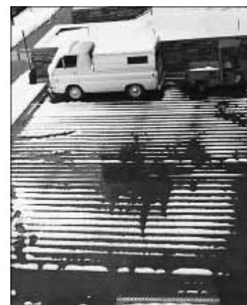
Melted snow pattern on a parking lot surface indicates the presence of underground hot water pipes used to aid snow removal. Energy from the water is conducted from the pipes to the pavement, where it causes the snow to melt.
