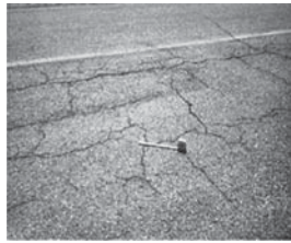
Block cracking
