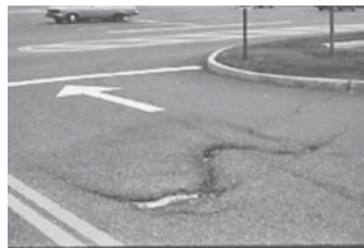
Slippage crack
