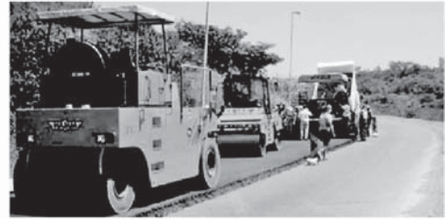
Paving 5 in. thick base layer with vögele paver and compaction with double drum vibrating roller and rubber-tired roller
