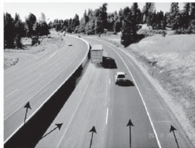
Recycled shoulder Recycled no.1 lane Mill and fill no.2 lane Recycled shoulder
