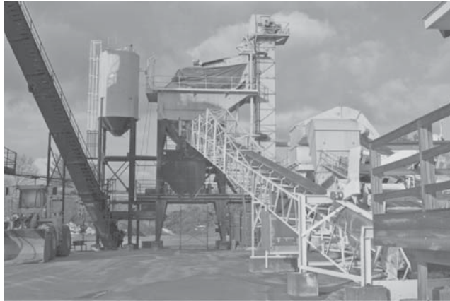
FIGURE 16.1 Hot mix asphalt plant. (Courtesy of Matthew Teto, All States Asphalt, Sunderland, MA.)
