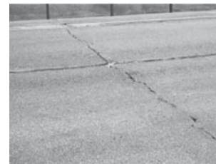
Reflective cracking
