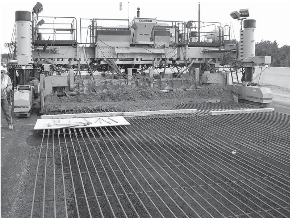
FIGURE 15.24 CRCP under construction.
