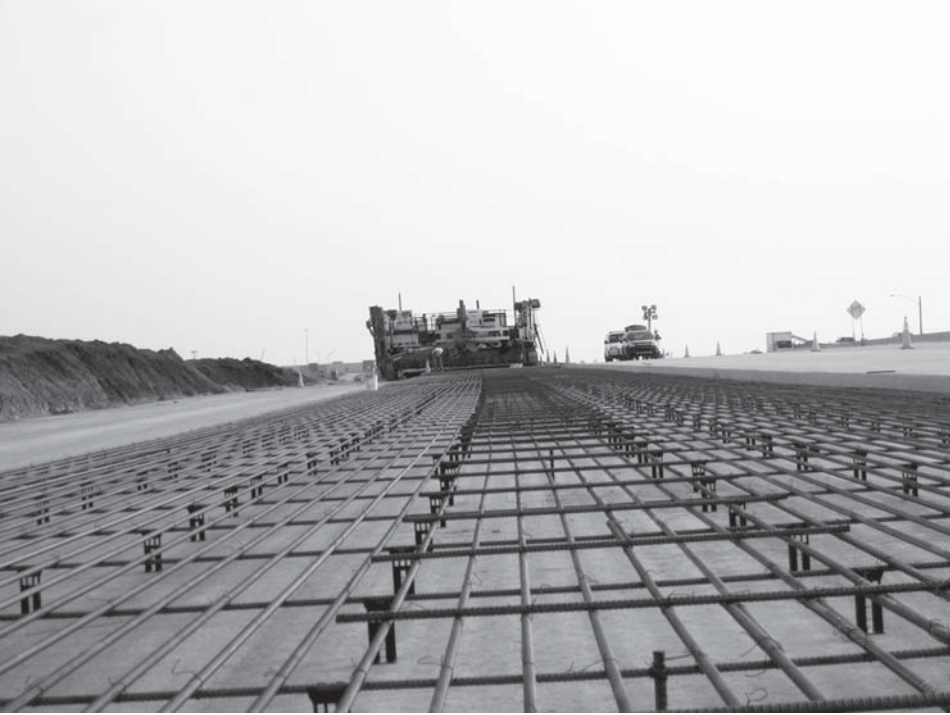
FIGURE 15.23 CRCP under construction.
