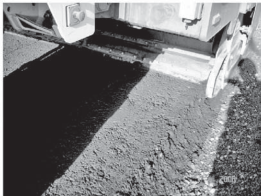
300 mm FDR with cement slurry with 5.8% cement
