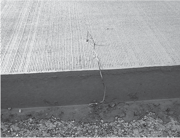
FIGURE 17.23 Field testing of concrete temperature for using the maturity test. (Courtesy of Wouter Gulden, ACPA-SE Chapter, Duluth, GA.)
