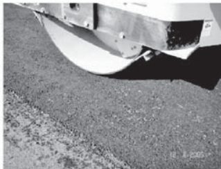
Compaction with steel drum roller
