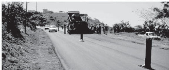
Paving the second lane: First lane opened to traffic immediately after compaction
