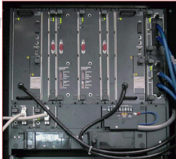
**Figure: LFCS - Field Control Unit (FCU)**
