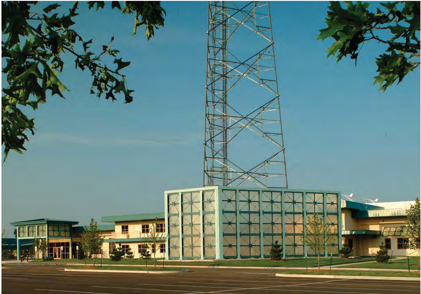
Station Addition Clear Channel Communications Tulsa
