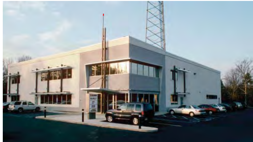
Building Facade before (above) after (below) Entercom Communications Greenville
