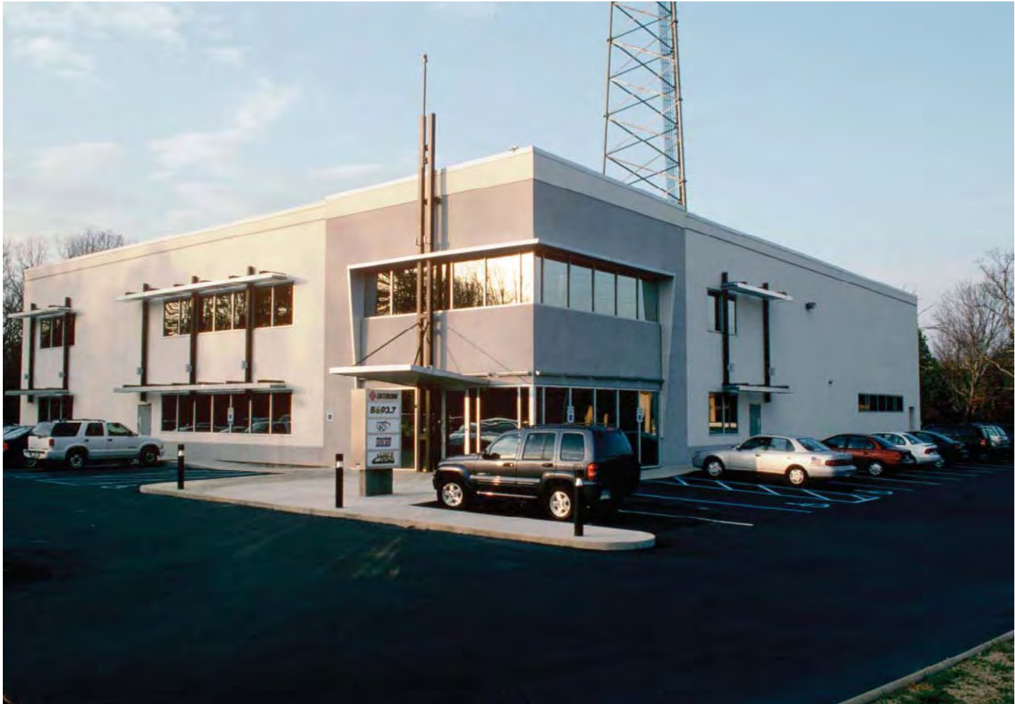
New Facility: Main Entry Renovation
