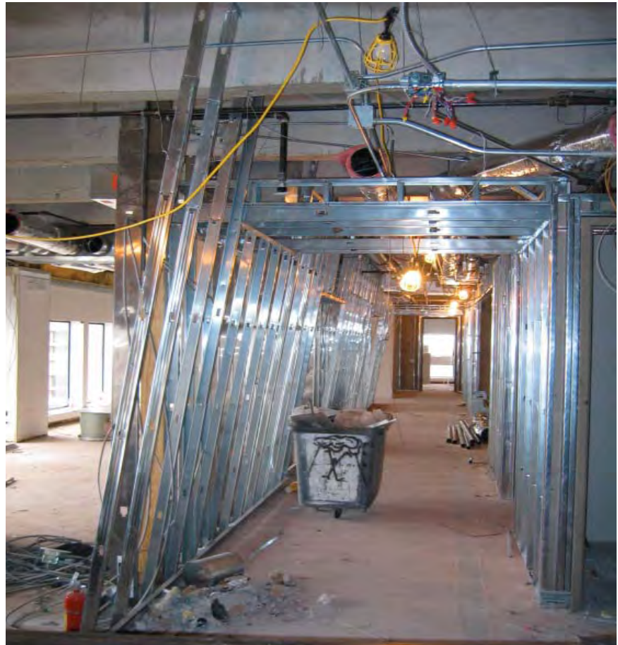
Construction Detail Entercom Communications Denver
