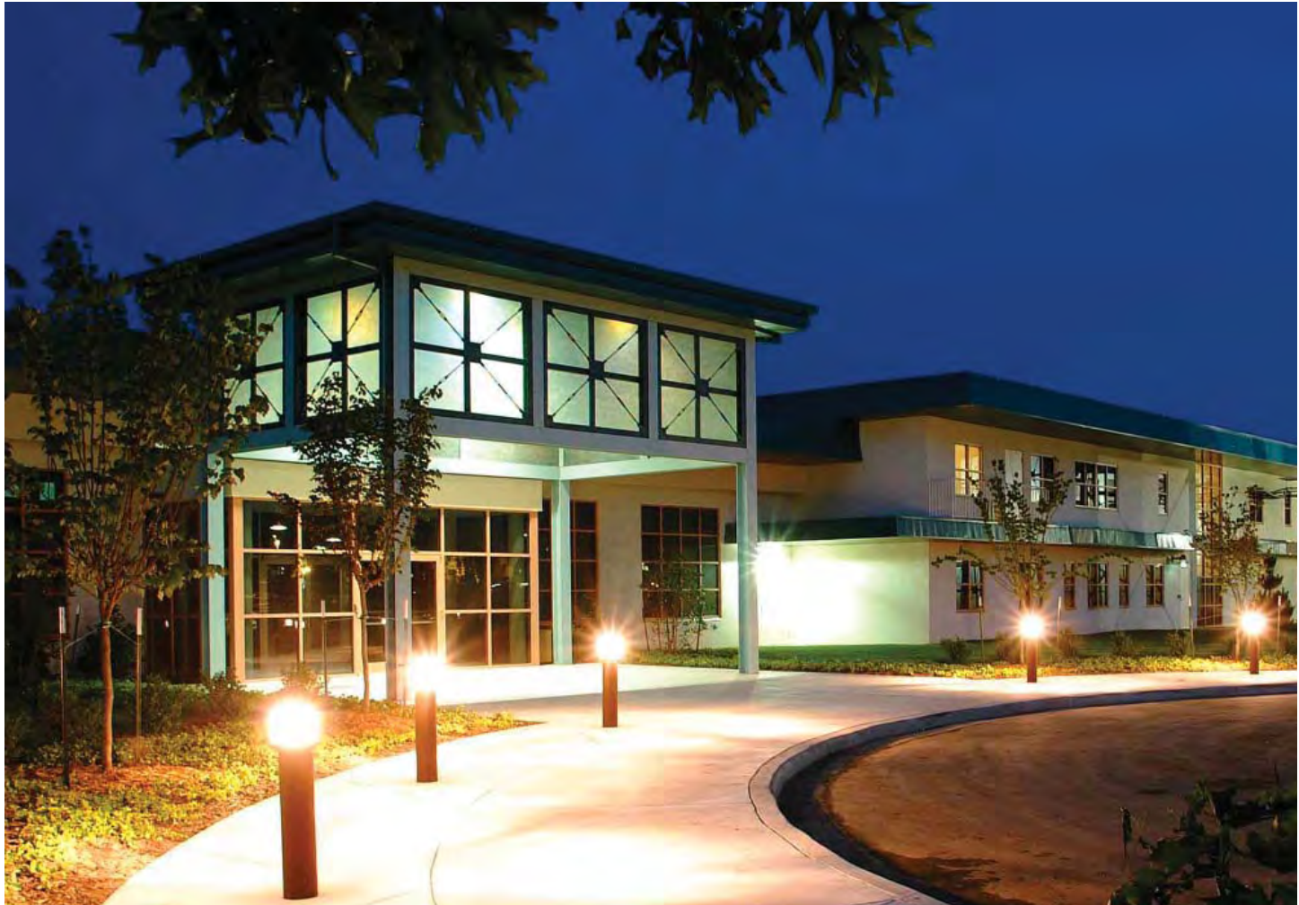
View of Renovation and New Entry Piece
