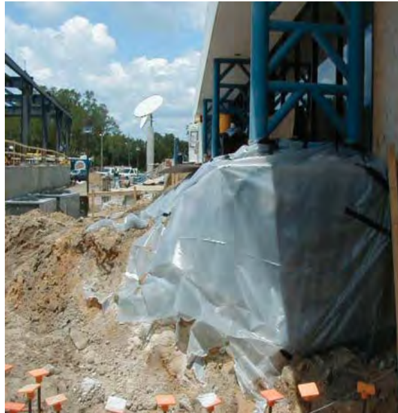
Construction Cox Radio Orlando
