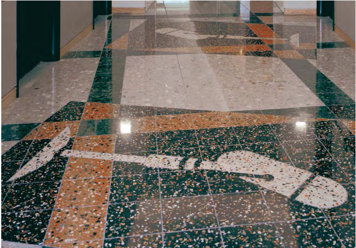
Elevator Lobby Floor Entercom Communications New Orleans
