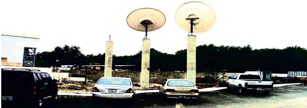
Construction Cox Radio Orlando
