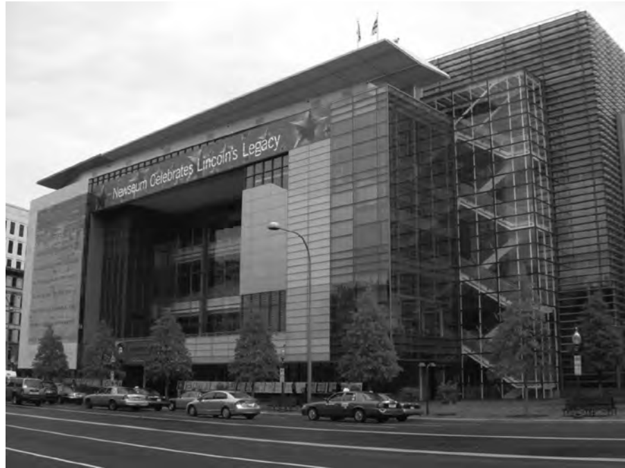
Figure 2-1 Radiant floor cooling project, Newseum, Washington, D.C. Asif Syed
