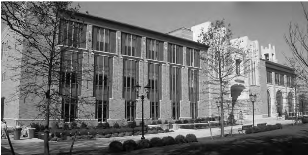
Figure 3–8 St. John's University, D'Angelo Building, Displacement ventilated classrooms in new construction. Asif Syed
