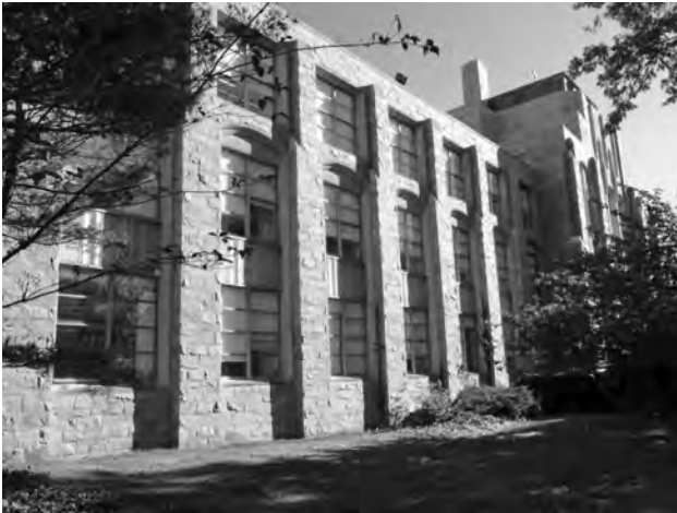
Figure 3–10 St. John's University, St. John's Hall, Renovation of existing 1950s building with displacement ventilation in classrooms. Asif Syed
