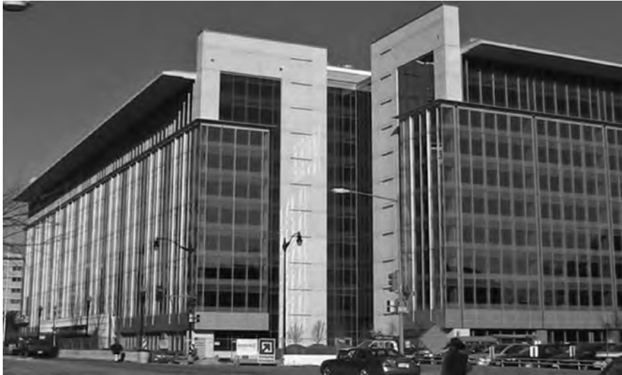
Figure 4–8 Constitution Center, Washington, D.C., chilled beam installation. TROX Technik
