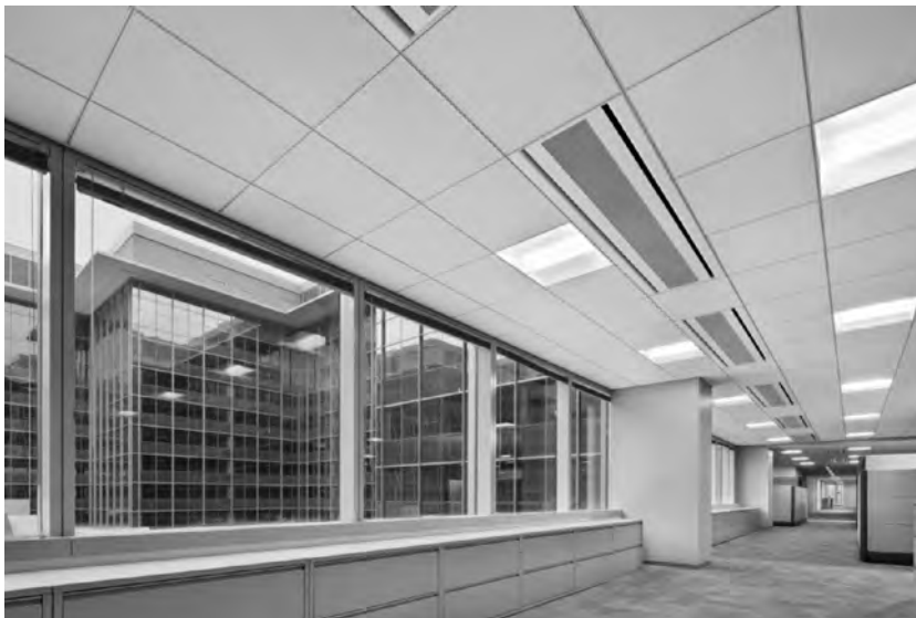
Figure 4-6 Chilled beam installation (in ceilings). Jeff Wolfram Photography, © JeffWolfram.com
