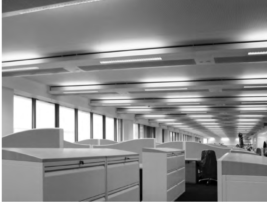
Figure 4–7 Multiservice chilled beam (without ceilings). TROX Technik
