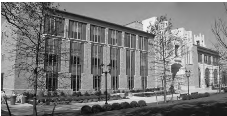
Figure 6–6 Displacement induction units at St. John's University, D'Angelo Center. Asif Syed
