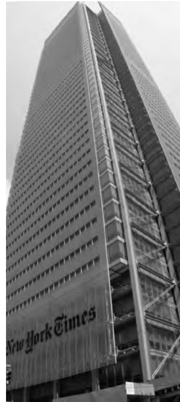
Figure 5–11 The New York Times headquarters building uses UFAD. Asif Syed
