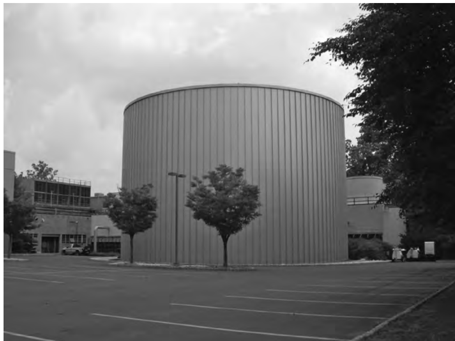
Figure 8–10 Outdoor chilled water storage tank. Asif Syed
