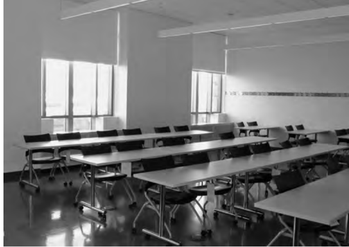
Figure 6-7 Interior classroom with induction units, St. John's University, D'Angelo Center. Asif Syed
