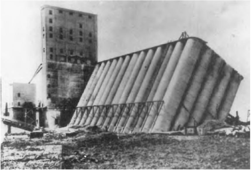
FIGURE 6.27 Transcona grain elevator bearing capacity failure.
