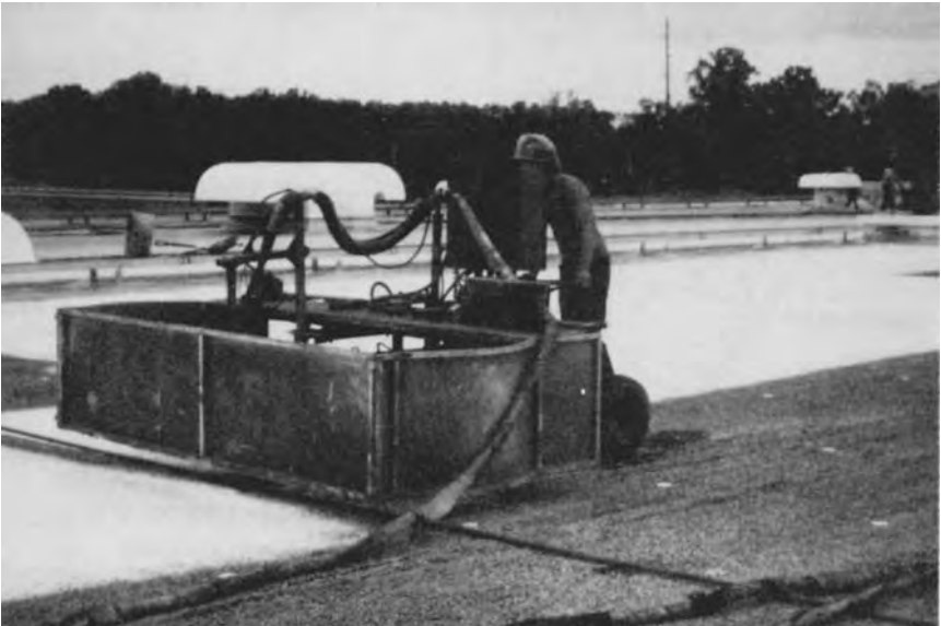
FIGURE 12.6 Robotic sprayer applying polyurethane foam.
