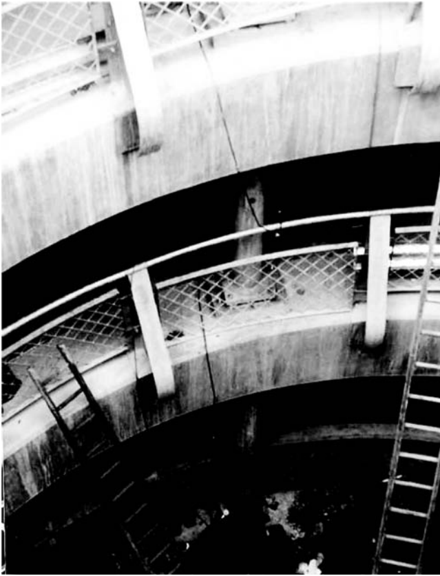
Figure 1.10 Additional steel columns.
