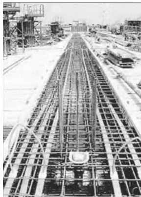
Figure 1.13 Typical beam under construction.
