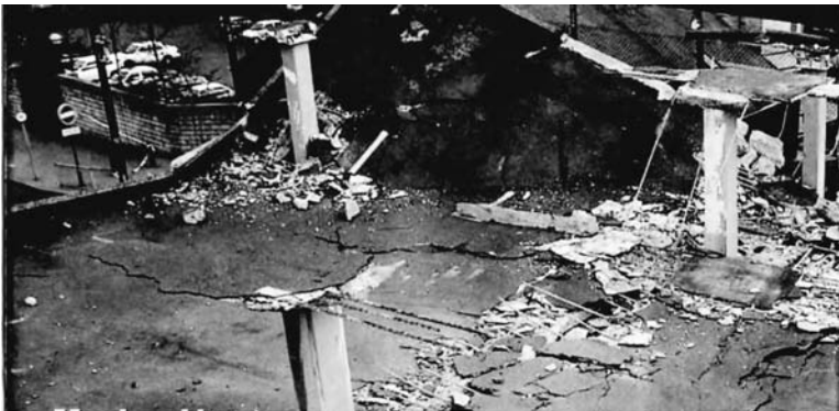
Figure 8.8 Collapse of roof of car park. (From Jonathan Wood, http://www.hse.gov.uk/research/misc/pipersrowptl.pdf .)
