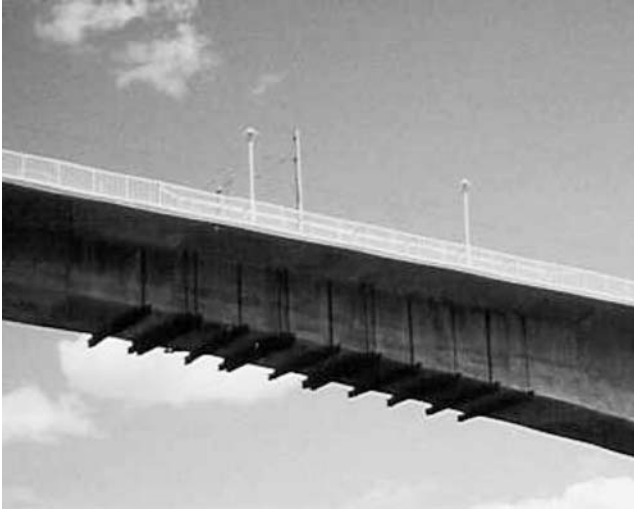
Figure 3.5 Temporary repair work on bridge.
