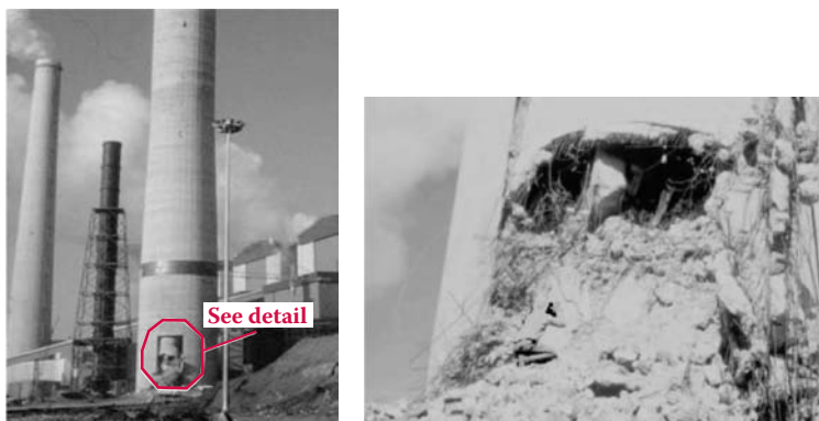
Detail: Close up of debris
