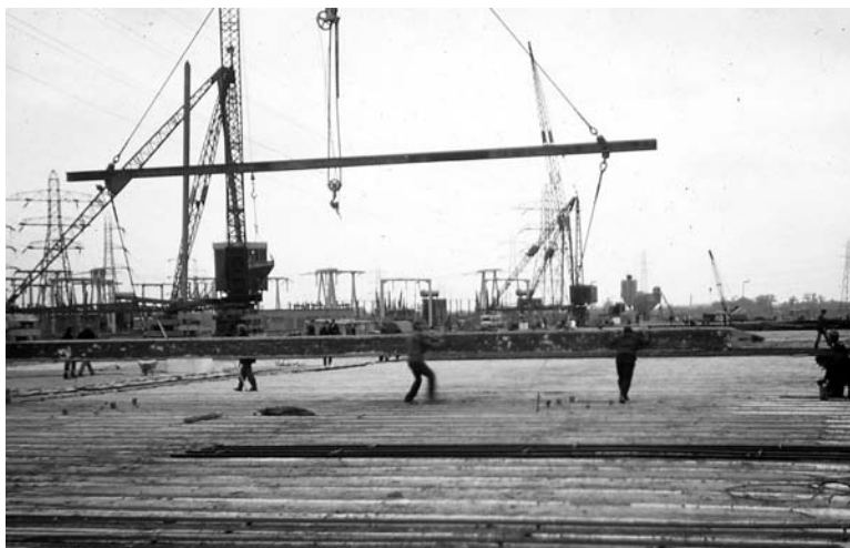
Figure 10.1 Pile casting yard.
