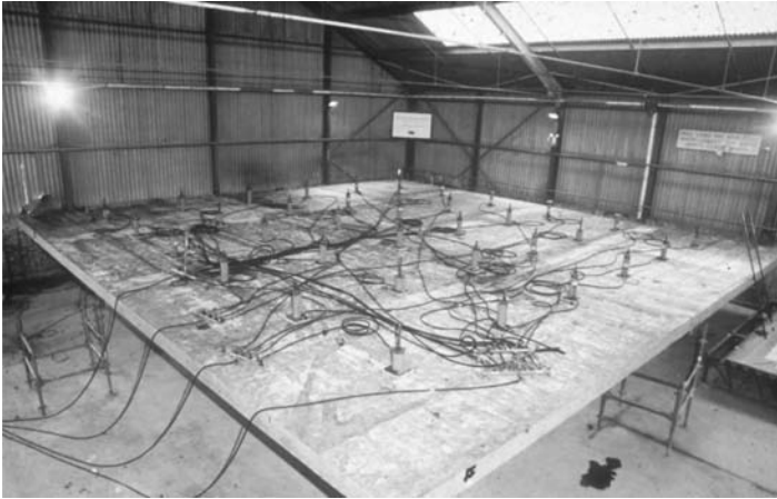
Figure 13.5 Construction of test flat slab. (Courtesy of Richard Scott.)
