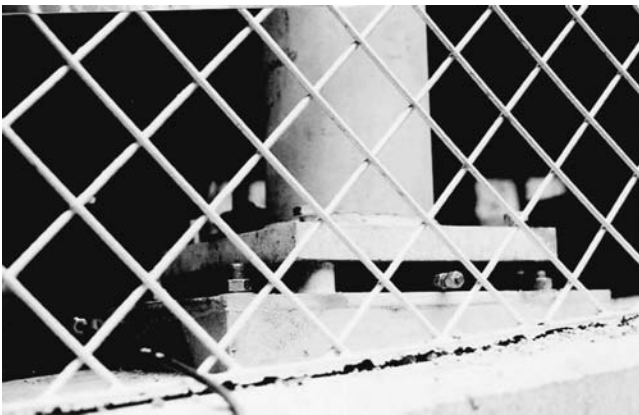
Figure 1.11 Flat jacks fitted under each new column.
