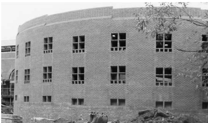
Figure 1.9 Car park with circular ramps.
