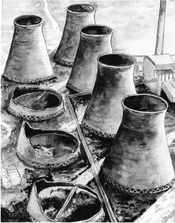
Figure 3.1 View of collapsed cooling towers. (Courtesy of Gillian Whittle.)
