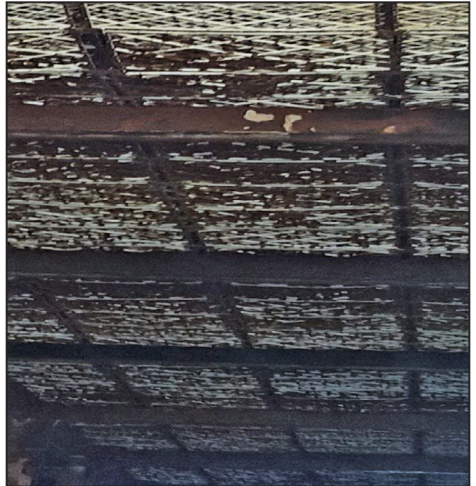
Fig.4 Scaled pp splash grid fill in the same thermal power plant
