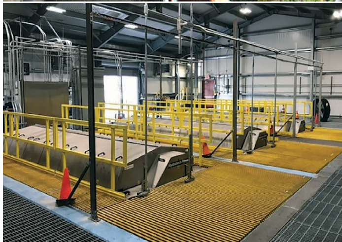
« Frame type » DiscFilters retrofitted into major US Power generator's old cooling water filtration system; only 3 of 8 basins were required
