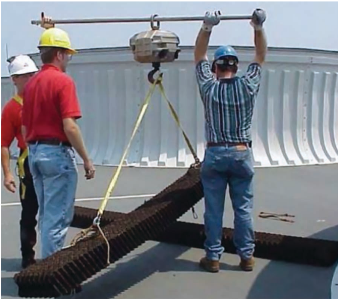
Figure 7 - Fill removal and weighing (EPRI, 2015)
