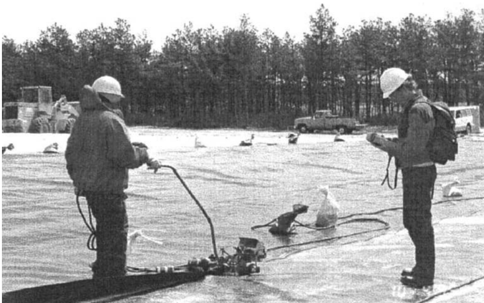
FIGURE 37.9 Monitoring seaming of a geomembrane liner.
