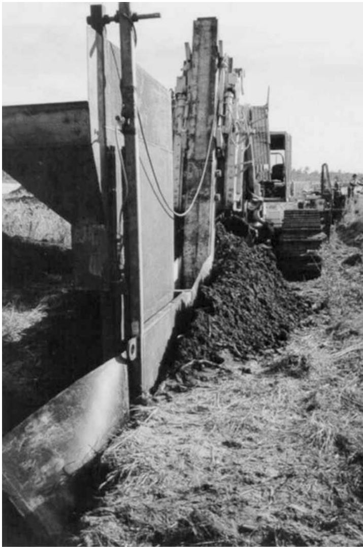
FIGURE 37.18 One pass trencher for installation of an HDPE vertical barrier system. (Photo courtesy of Groundwater Control, Inc.)
