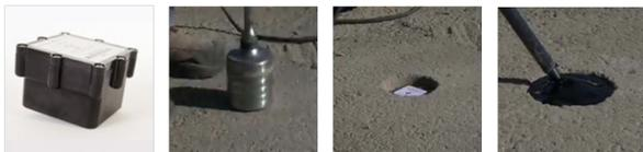
Figure 14: Installation procedure for embedding the sensors in the pavement.
