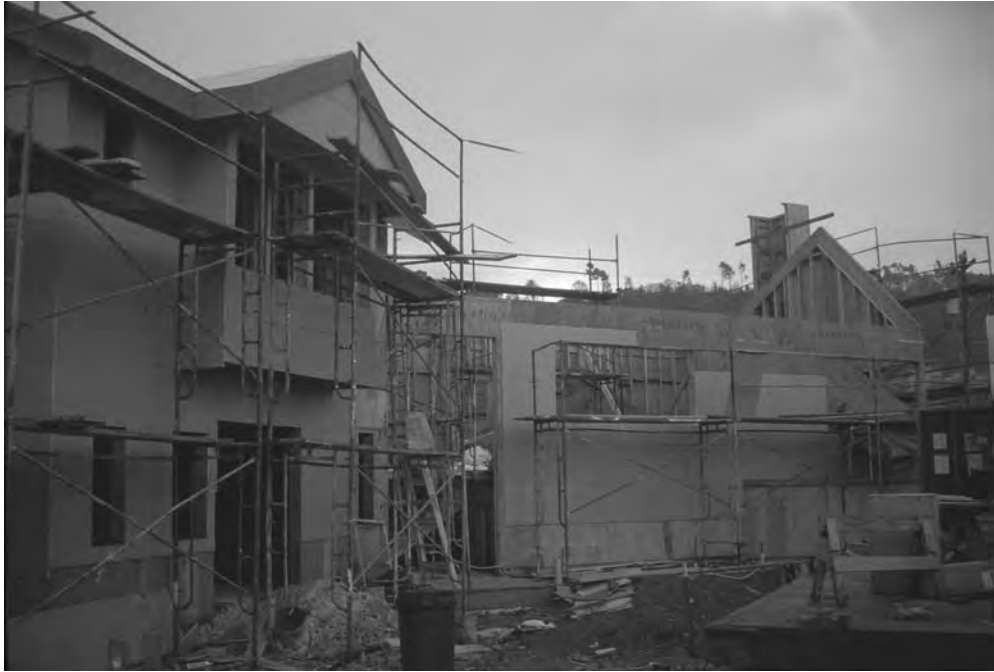
Figure A.5 Roof framing on second floor complete and preparing for the long rafters for the solar roof over living/kitchen/dining section.
