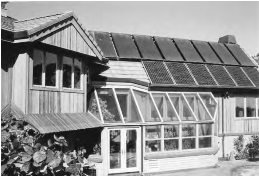
Figure 1.5 Completed Berkeley Solar house configuration.
