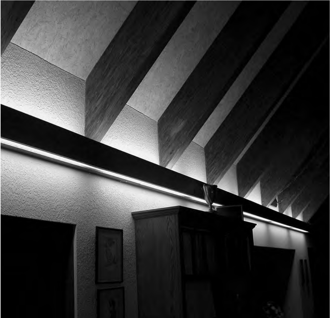
Figure 7.13 Photograph showing soffit lighting of ceiling rafters.
