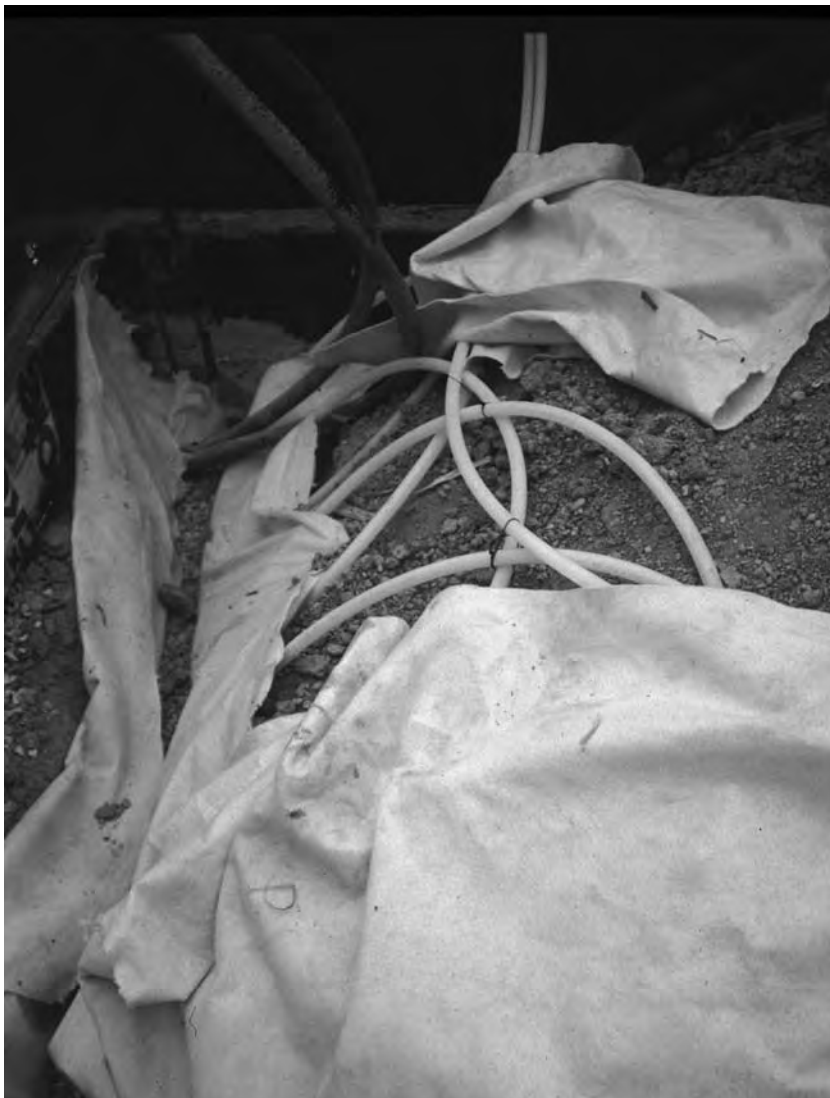
Figure 7.7 Photograph showing installation of ground coils.
