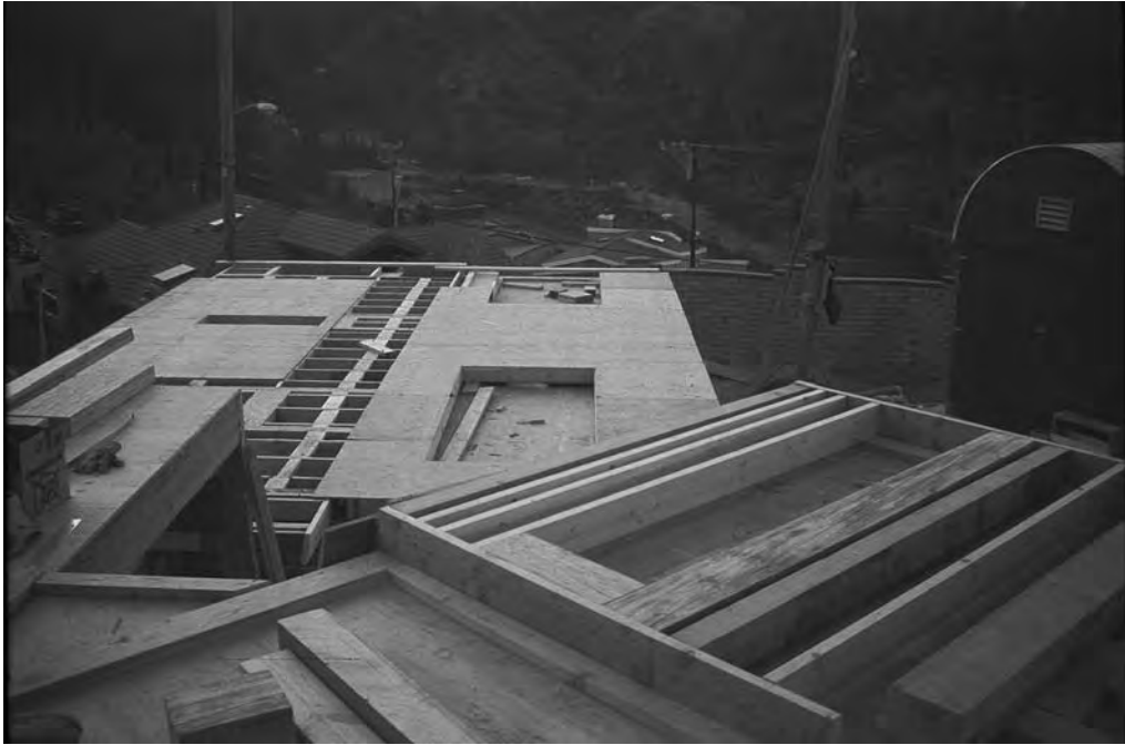
Figure A.3 Assembled second floor walls ready to tilt up.
