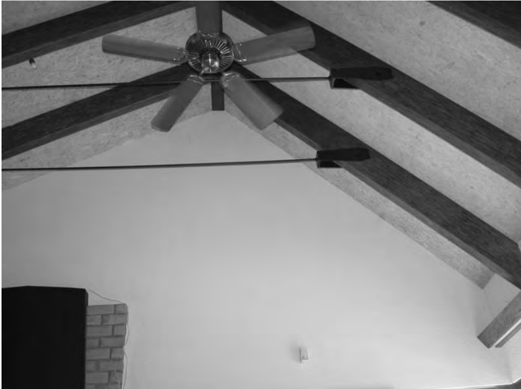
Figure 7.3 Exposed beam ceiling inside of 45° slope roof.
