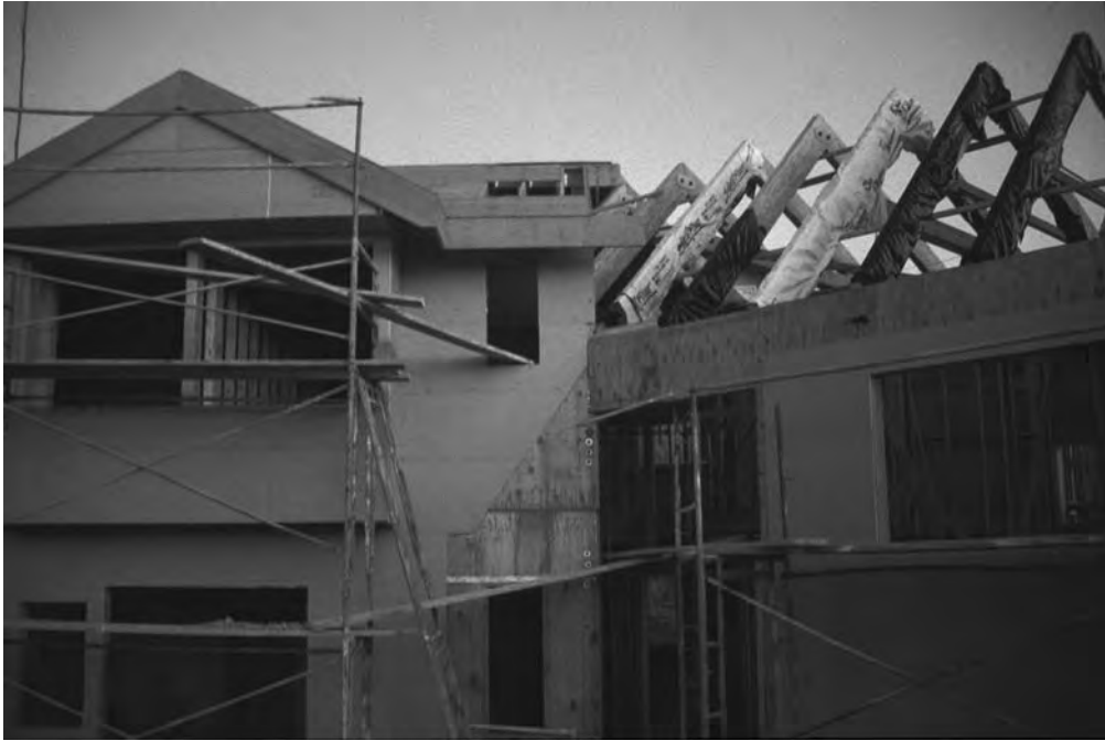
Figure A.7 Solar roof rafters in place preparing for the topping of large insulating R-control foam panels.
