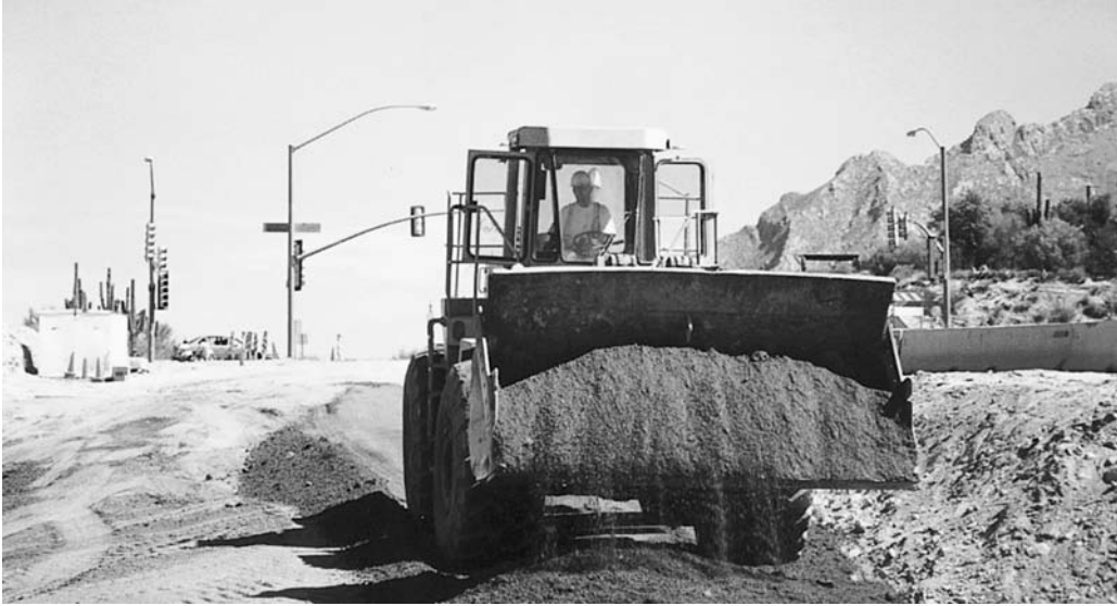
FIGURE 4.1 A highway under construction.
