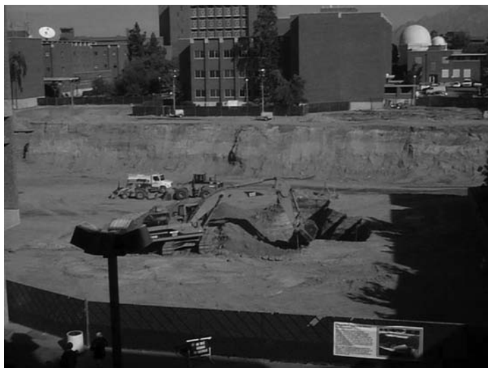
FIGURE 8.1 An excavation near a high-rise building. The applied loading history of soil elements at the same depth at the edge of the excavation and at, say, the center of the building will be different.
