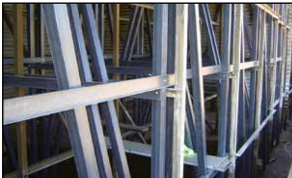
Figure 7: New Fiberglass Coil Supports alongside Existing Supports
