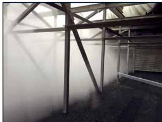
Figure 9: Clear Boundary between Dry and Wet Areas in the Tower Plenum
