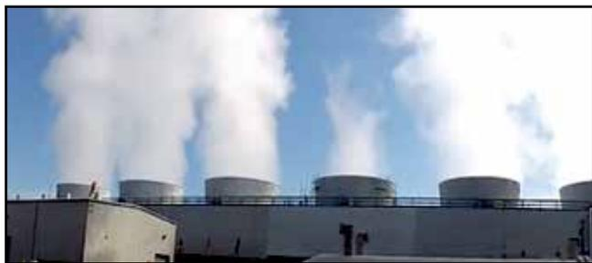
Figure 10: The 4th Cell from the Left Is Operating In Wet-Dry Mode
