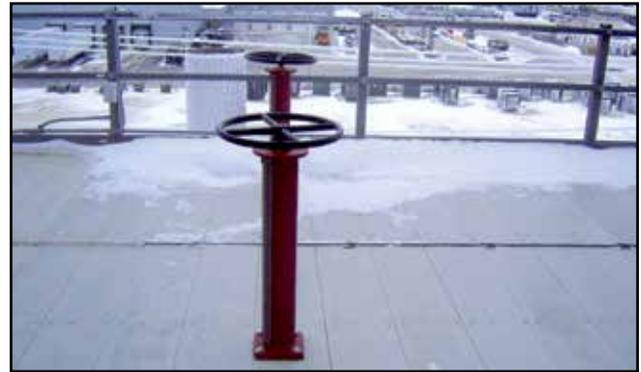
Figure 14: Valve Actuators on Fan Deck
