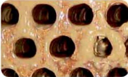
Biofilm on a heat exchanger tube sheet
