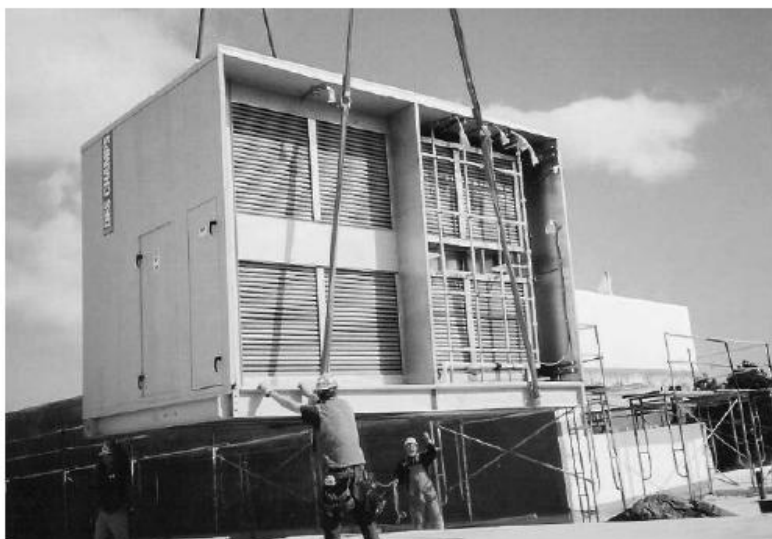
Fig. 7.20 A heat pipe heat exchanger with spray bars (visible on the RHS). These are used on the exhaust side for indirect evaporative cooling, in addition to sensible heat transfer (Courtesy Deschamps Technologies).
