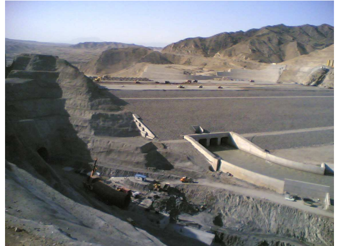
Fig.2 shows excavation and Embankment of the dam
