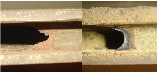
Figure 5. Erosion on the blades trailing edge of first impeller of third section.
