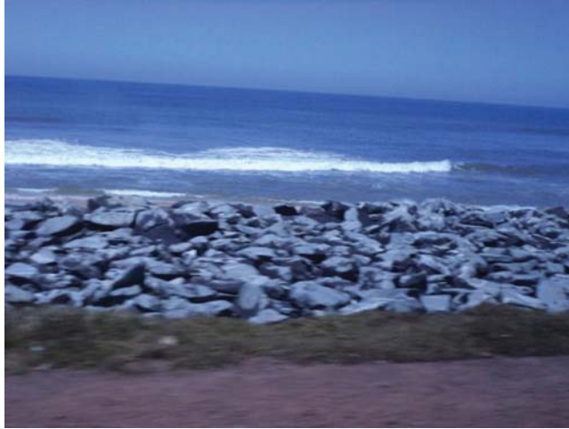
Figure 6.4 Boulder placed on seashore to protect from tides.
