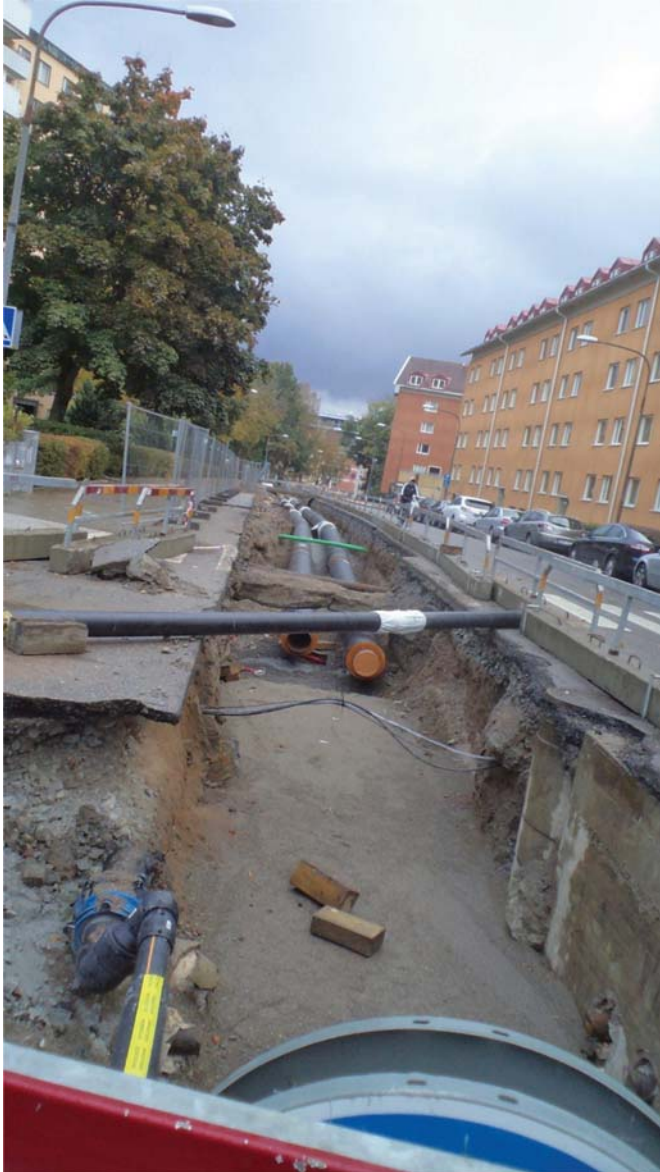
Figure 2.12 Laying of pipe in progress in Europe.
