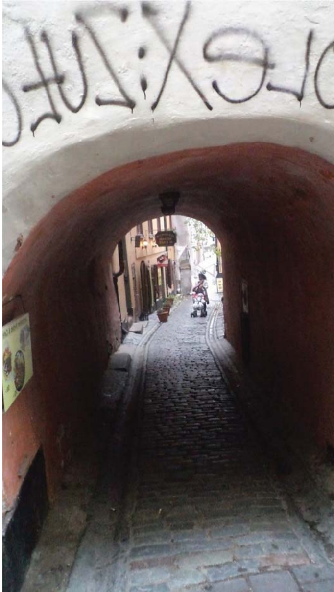
Figure 3.16 Storm water drains in narrow passage way of Stockholm.
