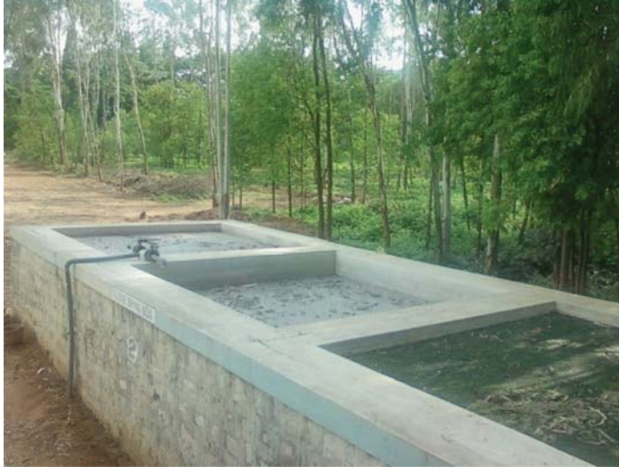
Figure 4.48 Sludge drying beds.
