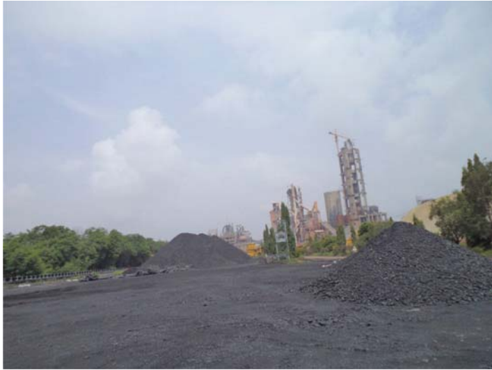
Figure 1.7 Raw material storage in cement plant.
