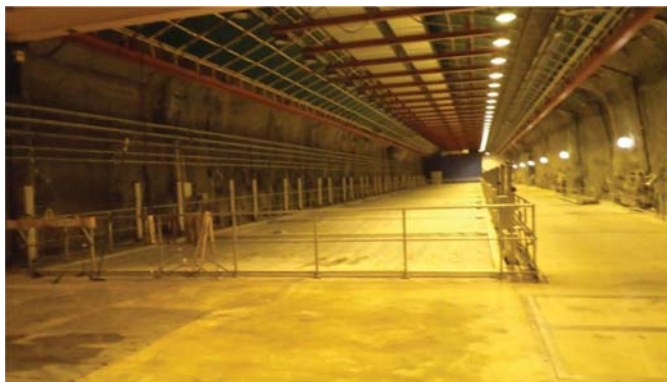
Figure 4.5 Rapid sand filters in sewage treatment plant at Bromma, Stockholm, Sweden.
