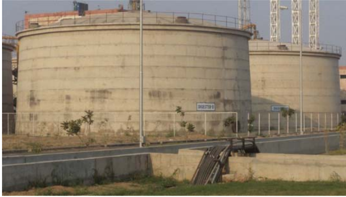
Figure 4.49 View of digesters.
