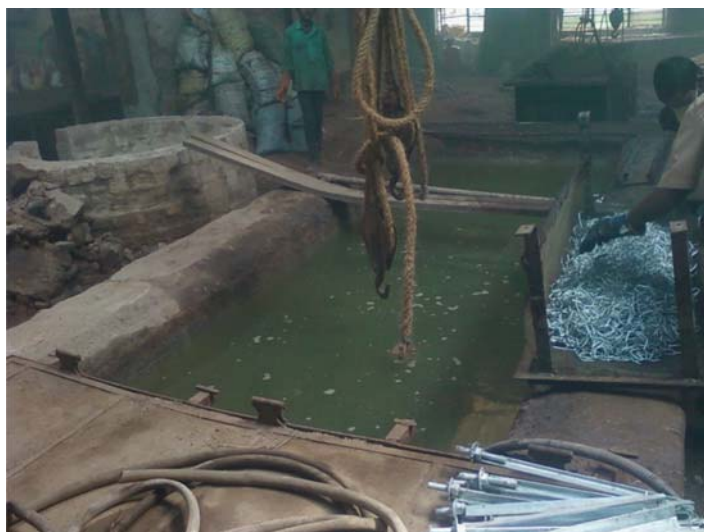
Figure 5.14 A typical galvanizing rinsing tank.
