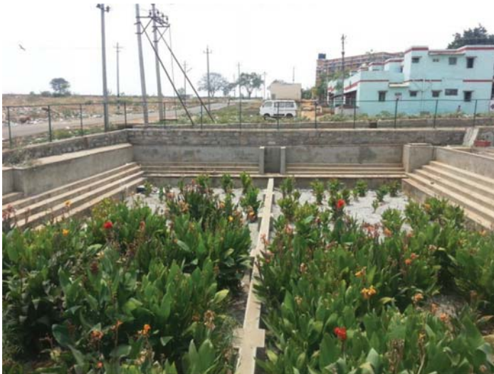
Figure 4.34 View of constructed wetlands.
