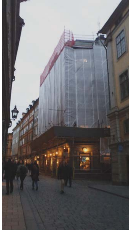
Figure 8.20 Building under construction covered completely to avoid dust nuisance.
