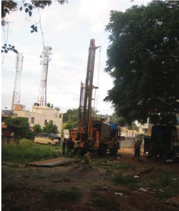
Figure 3.6 Bore well drilling under progress.
