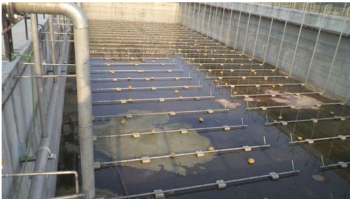
Figure 4.23 Piping arrangement for submerged aerators.
