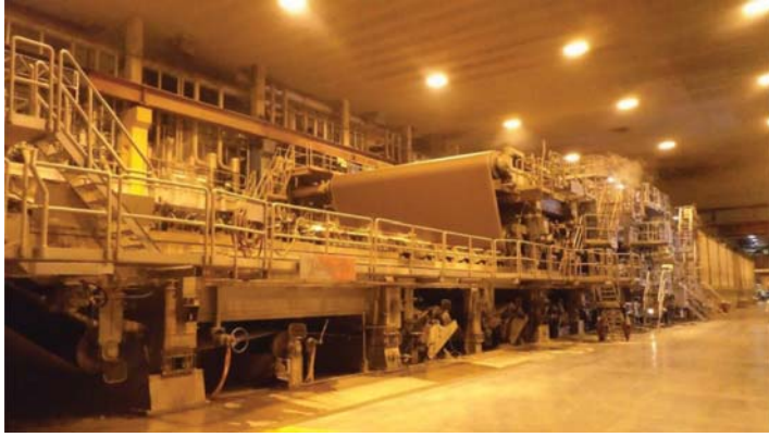
Figure 5.27 View of paper mill.
