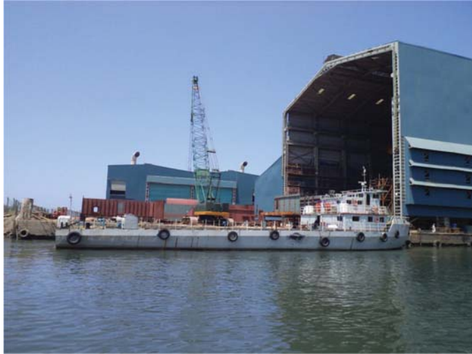
Figure 1.12 Ports and harbours generate a range of wastes, which include minerals and damaged products.
