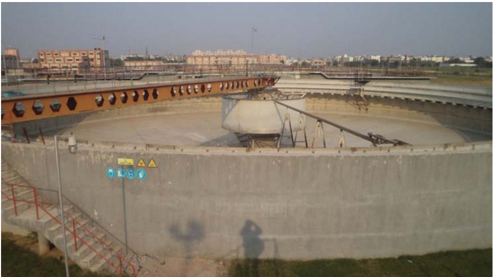
Figure 8.7 Safety signs and handrails on stairs of sedimentation tank.
