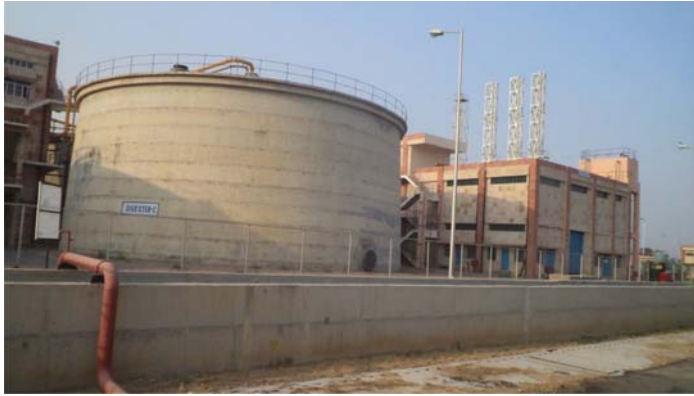
Figure 4.8 Sludge digester and generator building at Okhla, Delhi, India.
