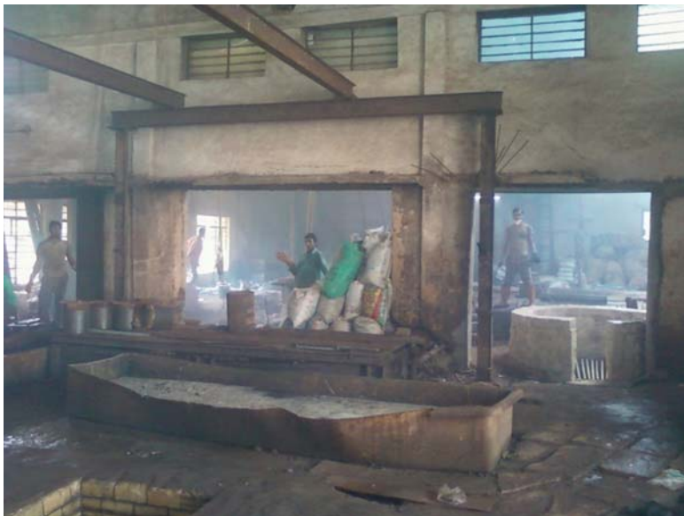
Figure 8.15 Effluent from operations with poor safety precautions.
