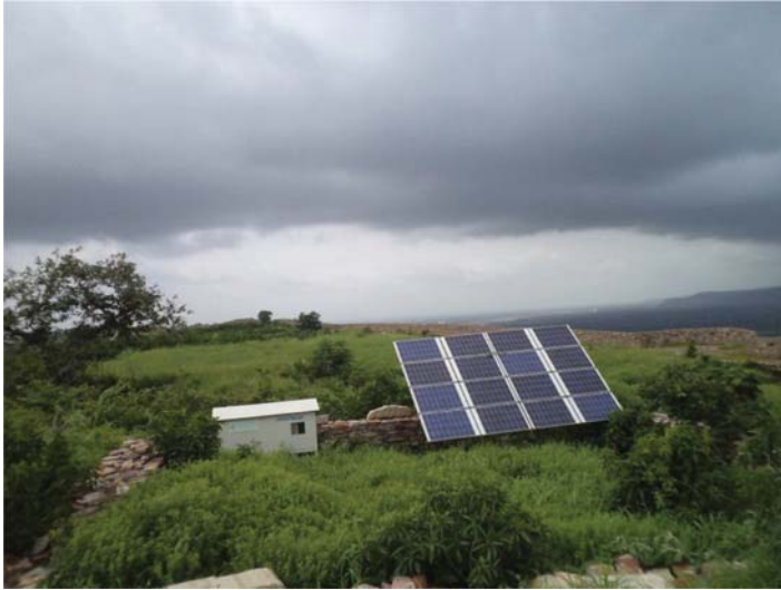
Plate 4.51 Solar energy is an attractive idea but still not practical due to high cost associated with installation of photovoltaic cells.
