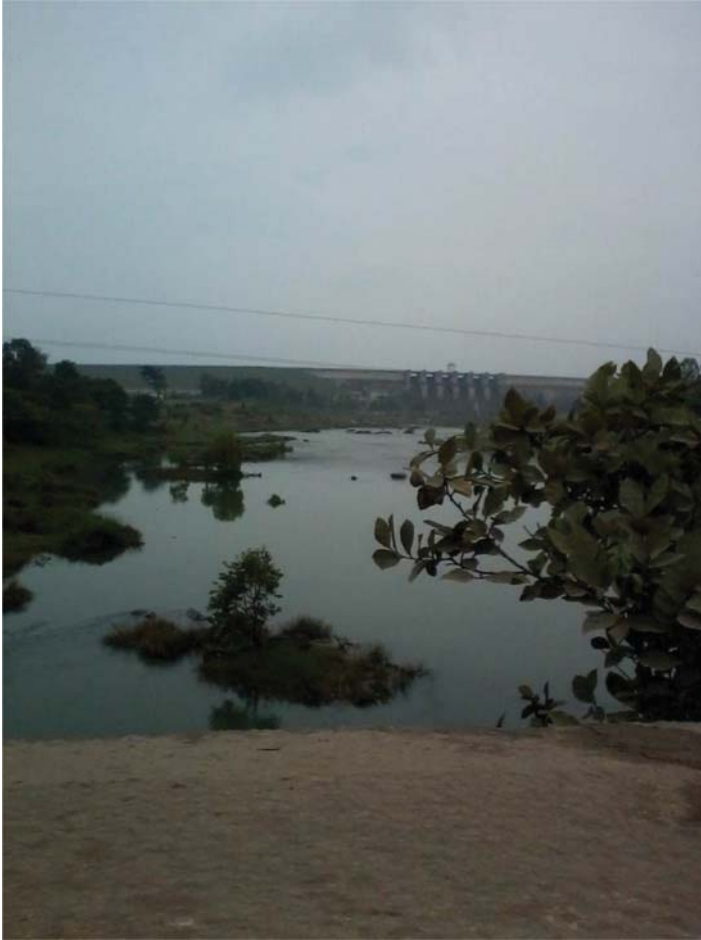
Figure 3.2 View of dam across river.
