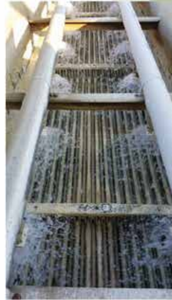
Poor Water Distribution
