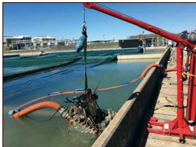
Figure 3 - Robot being deployed into a basin using custom crane
