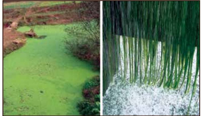
Figure 5 (Left). Algae completely covering a pond surface. and Figure 6 (Right). Algae hanging from plastic tower fill.
