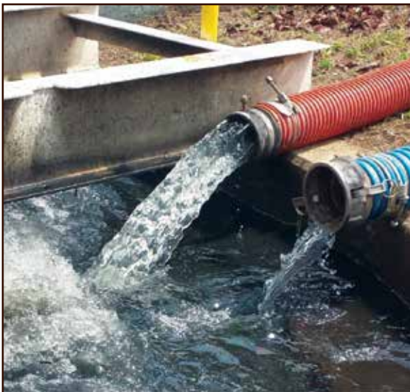
Figure 8 - Clean water pumped into the basin after remediation process
