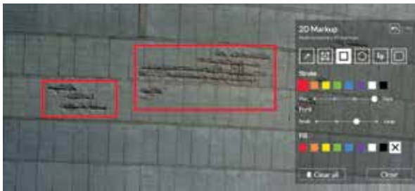
Figure 2 – Inspection-grade photo from 3D model
