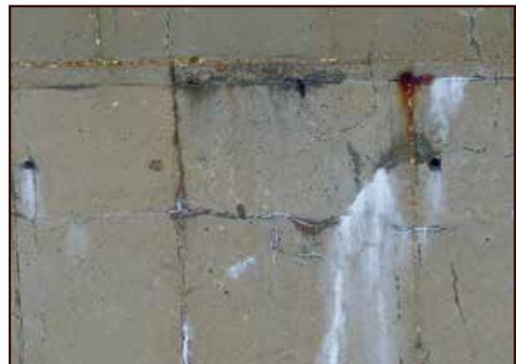
Drone Photo of Cracks and Corrosion at 400'
