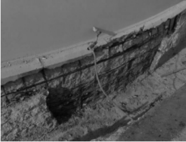
FIGURE 10.2 Removal of delaminated concrete from ring beam.
