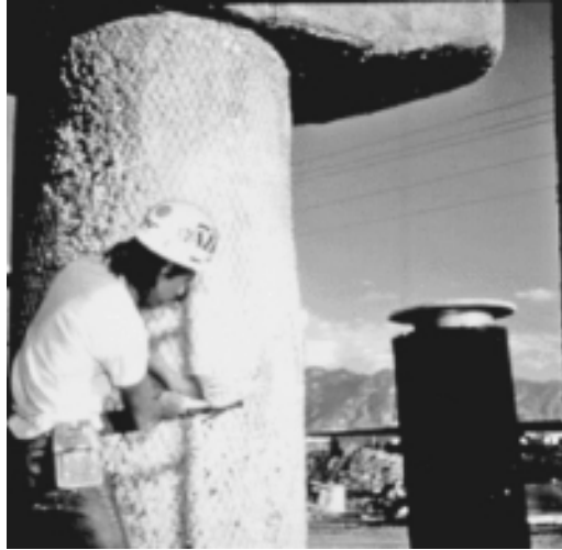
FIGURE 9.10 Fixing titanium on a concrete column.
