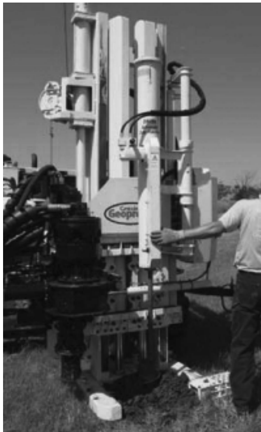
FIGURE 13.4 Rig for the standard penetration test.
