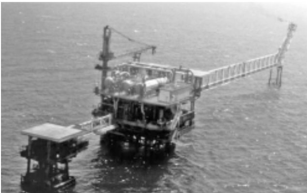
FIGURE 12.1 Production platform with bridges.
