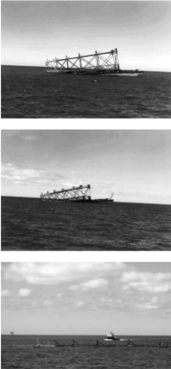
FIGURE 12.38 (a) Step 1—launching of jacket. (b) Step 2—launching of jacket. (c) Step 3—laying the jacket on the sea by floating.
