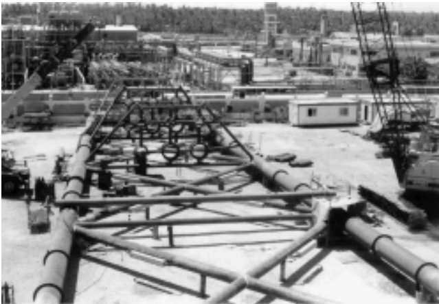
FIGURE 12.32 Assembly conductor guide to the jacket.
