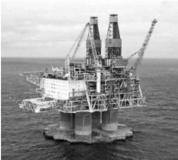
FIGURE 12.4 Concrete gravity platform.
