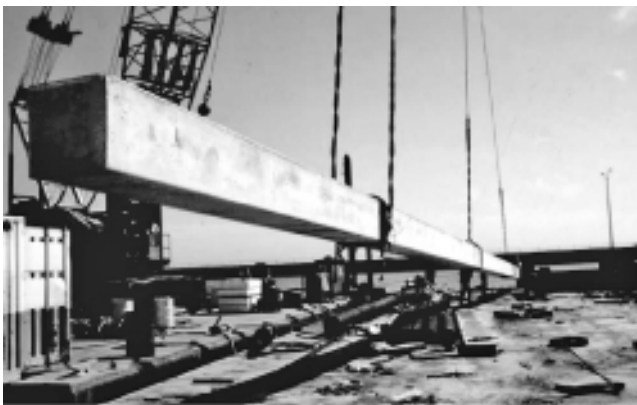
FIGURE 13.15 Lifting of the concrete pile.
