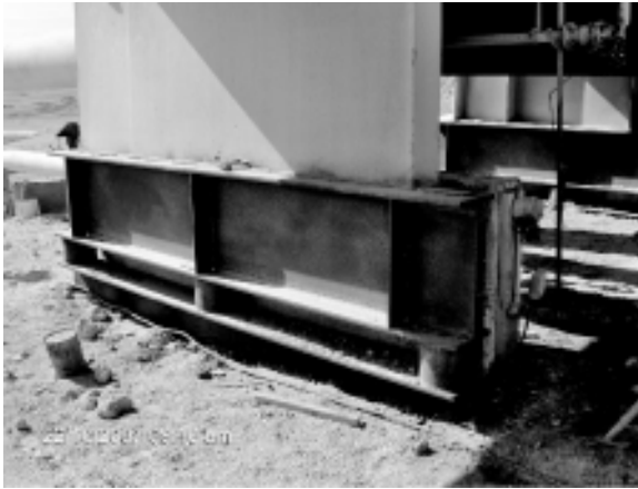
FIGURE 10.1 Temporary repair using steel sections.
