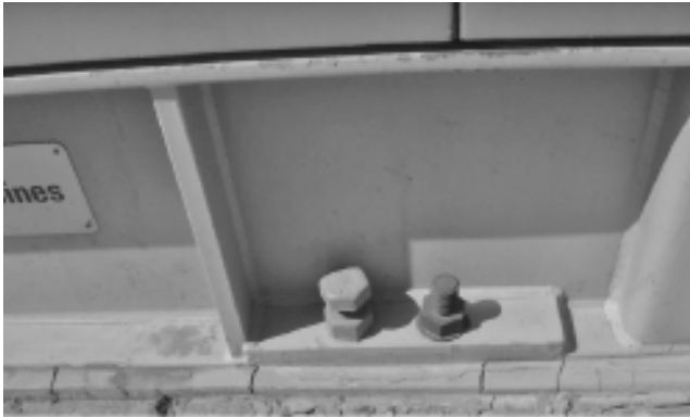
FIGURE 4.3 Fixing the skid to concrete.
