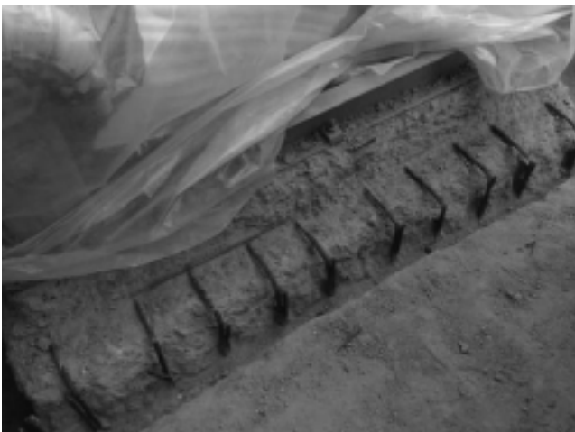
FIGURE 10.3 Removal of concrete cover from pump foundation.
