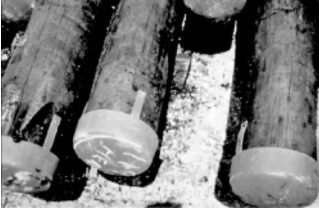
FIGURE 13.11 Wood pile with steel cap.
