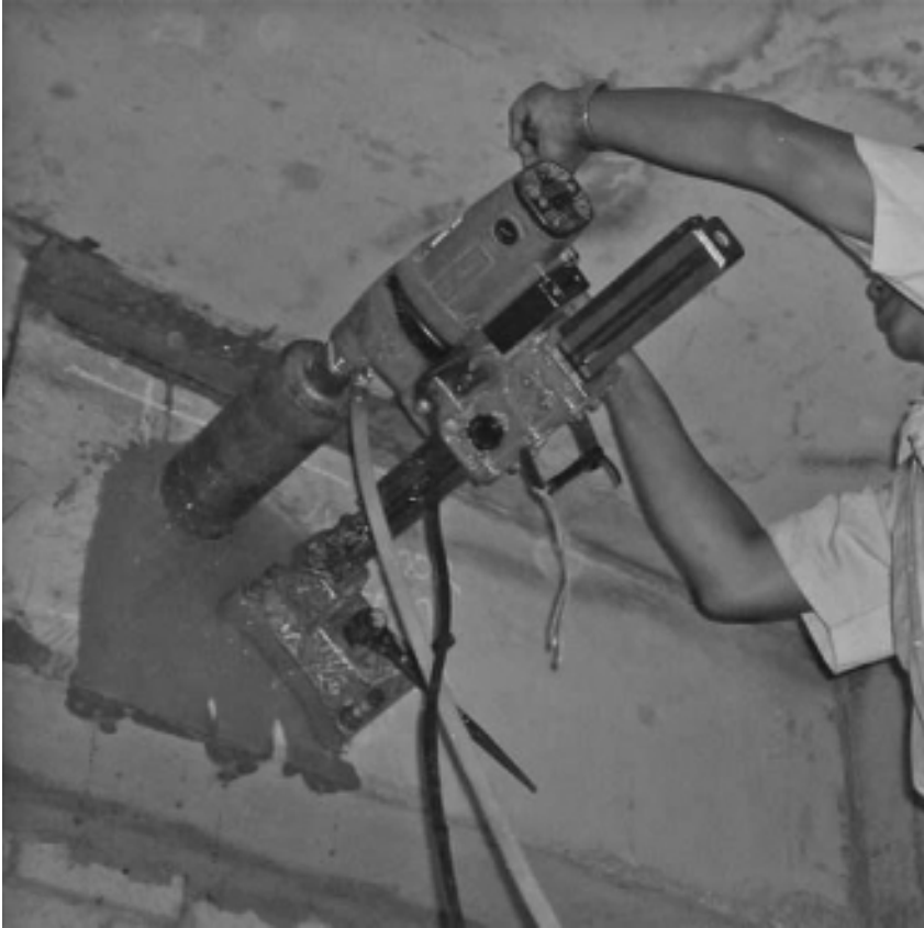
FIGURE 8.3 How to take a core sample.
