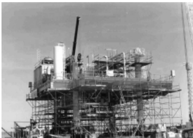
FIGURE 12.33 Assembly for topside with facilities.
