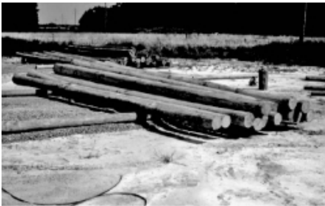
FIGURE 13.10 Preparation of wood piles.
