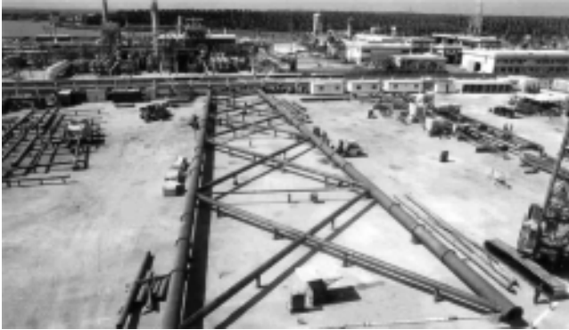
FIGURE 12.29 Jacket fabrication on the yard.
