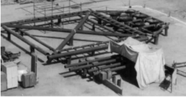
FIGURE 12.31 Fabrication of conductor guide.
