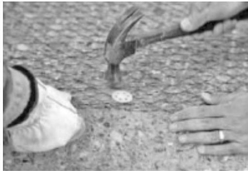
FIGURE 9.12 Fixing titanium mesh by plastic binder.
