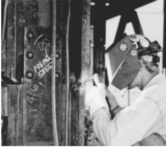
FIGURE 7.24 Welding in an existing building.
