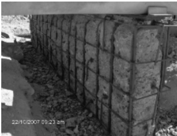
FIGURE 10.4 Repair of concrete pedestal.
