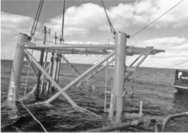
FIGURE 12.39 Lifting and installing of jacket.
