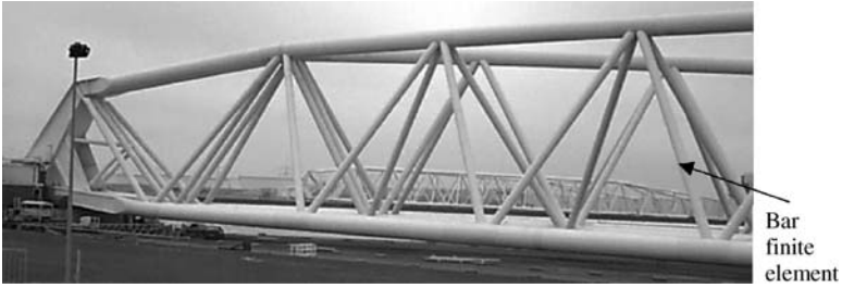
Figure 2.1 A bridge truss.
