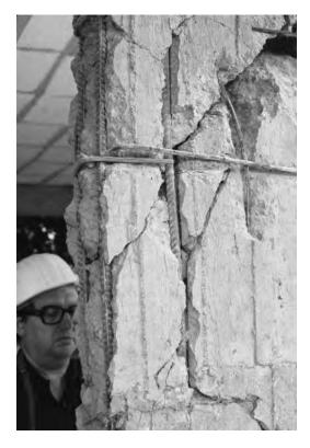
Figure 11.16 Shear wall failure due to shear: Kalamata, Greece (1986).
