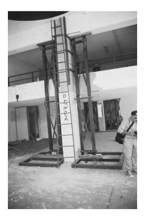
Figure 12.18 Steel profile props for the repair of a damaged column; Kalamata, Greece (1986).
