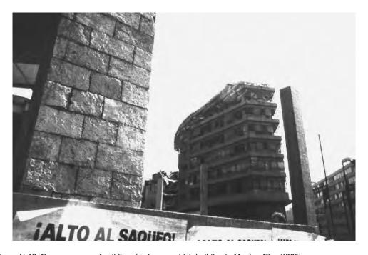
Figure 11.48 Consequences of soil liquefaction on a high building in Mexico City (1985).
