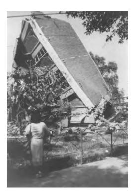
Figure 11.40 Torsional collapse of a building in Mexico City (1985).
