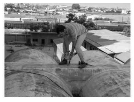
Figure 14.12 Hammer tests at MELISSARI Complex (Thessaloniki).
