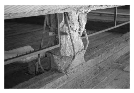
Figure 11.9 Explosive cleavage failure of a short column: Kalamata, Greece (1986).
