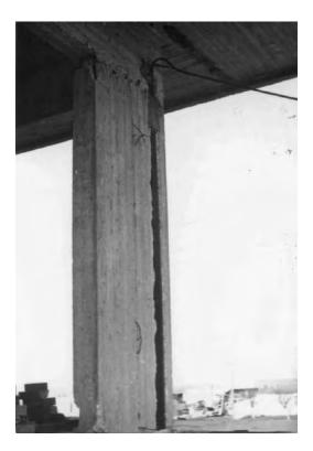
Figure 11.13 Shear wall crack at the construction joint at the top of an R/C wall, Kalamata, Greece (1986).
