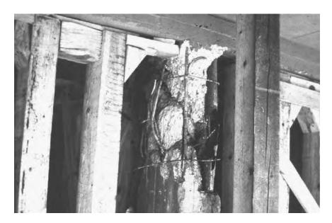
Figure 12.17 Timber propping of a damaged column; Kalamata, Greece (1986).
