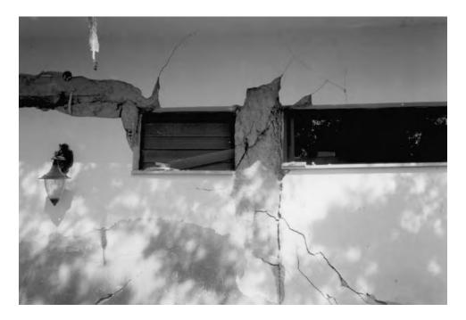
Figure 11.8 Explosive cleavage failure of a short column: Kozani, Greece (1996).
