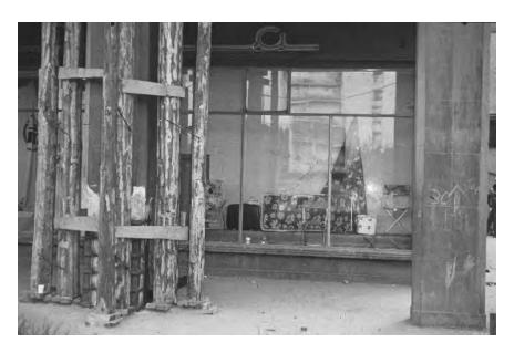
Figure 12.16 Timber propping of a damaged column; Bucharest, Romania (1977).
