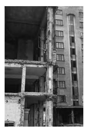
Figure 11.46 Collapse of a building in Bucharest during the 1977 earthquake. The building, as depicted in the illustration, had been repaired after the 1940 earthquake.
