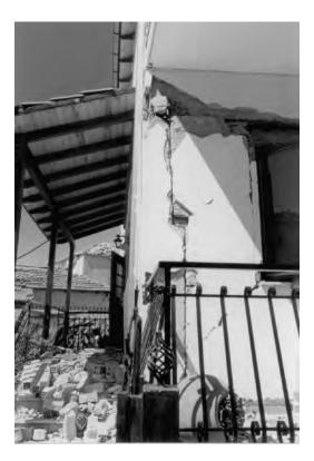
Figure 11.32 Damage to masonry walls: Kozani, Greece (1996).
