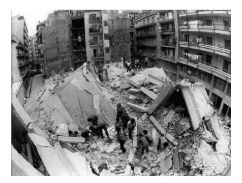
Figure 11.49 Collapse of an eight-storey corner building in Thessaloniki, Greece (1978).
