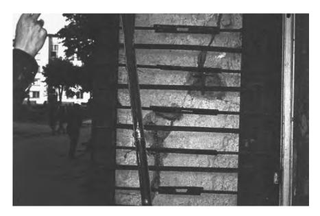
Figure 12.19 Confinement of an R/C wall using external profiles, for temporary propping and in parallel final repair.
