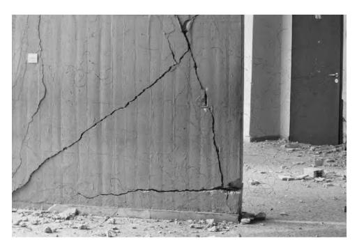
Figure 11.15 Shear wall failure: Kalamata, Greece (1986) failure to shear and in parallel to bending.
