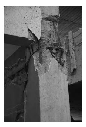
Figure 11.26 Failure of an exterior joint in a multistorey building Kalamata, Greece (1986).
