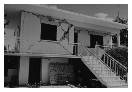
Figure 11.31 Damage to masonry walls: Kalamata, Greece (1986).
